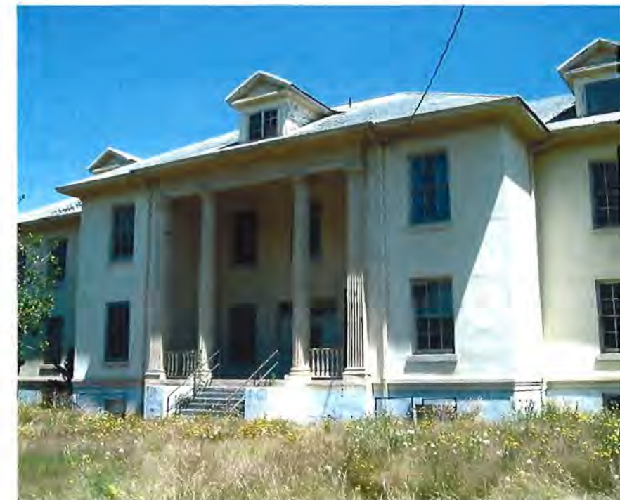
Renovation of the Crescent campus buildings is planned
