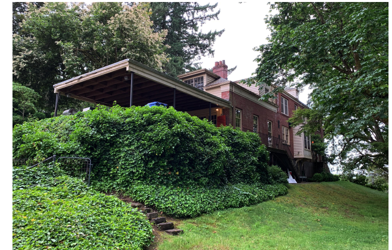
VIEW FROM NORTH-EAST
