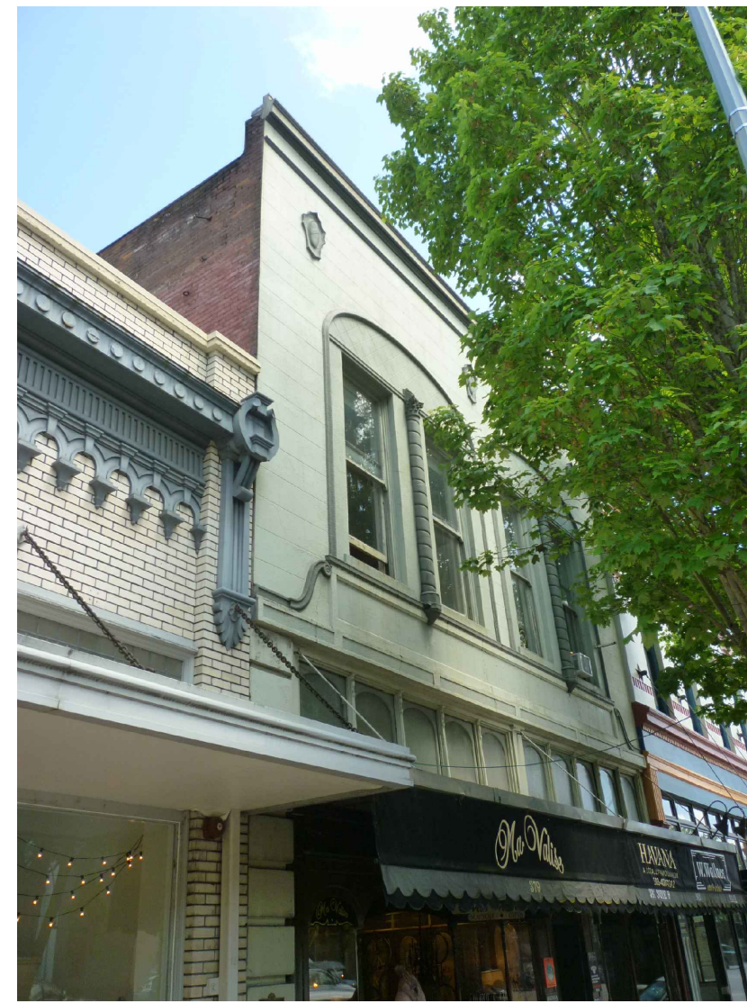
EXISTING SOUTH FACE
