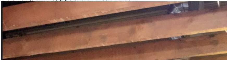
Jesiah and Destin heat stripped the beautiful siding that had been hidden under drywall in the kitchen. The drywall also hid a crumbling chimney pipe and a transom window.
