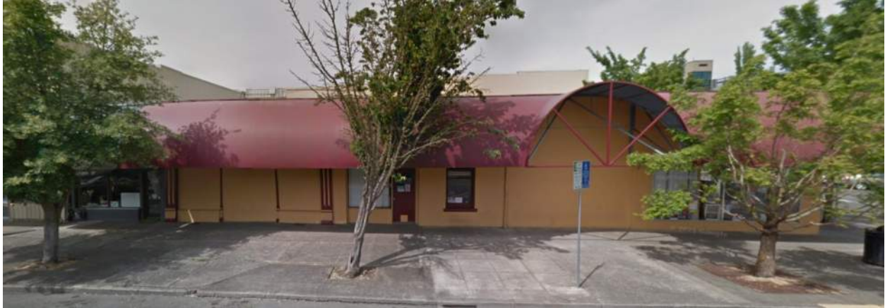
South façade of building frontage (looking north from Chemeketa St. NE)
