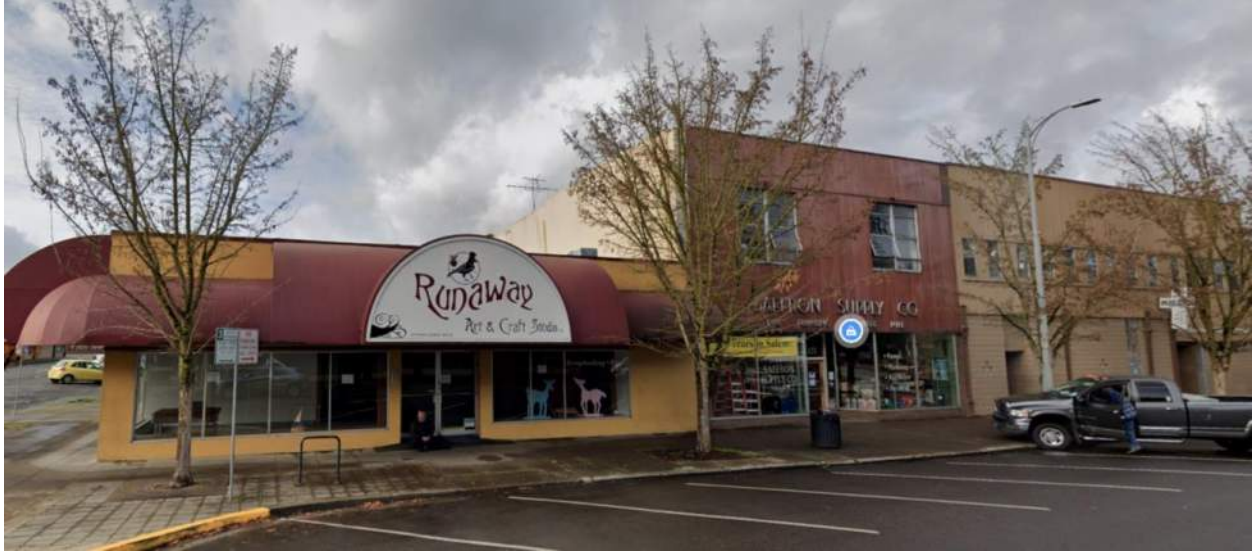
East façade of building frontage (looking west from Commercial Street NE);
