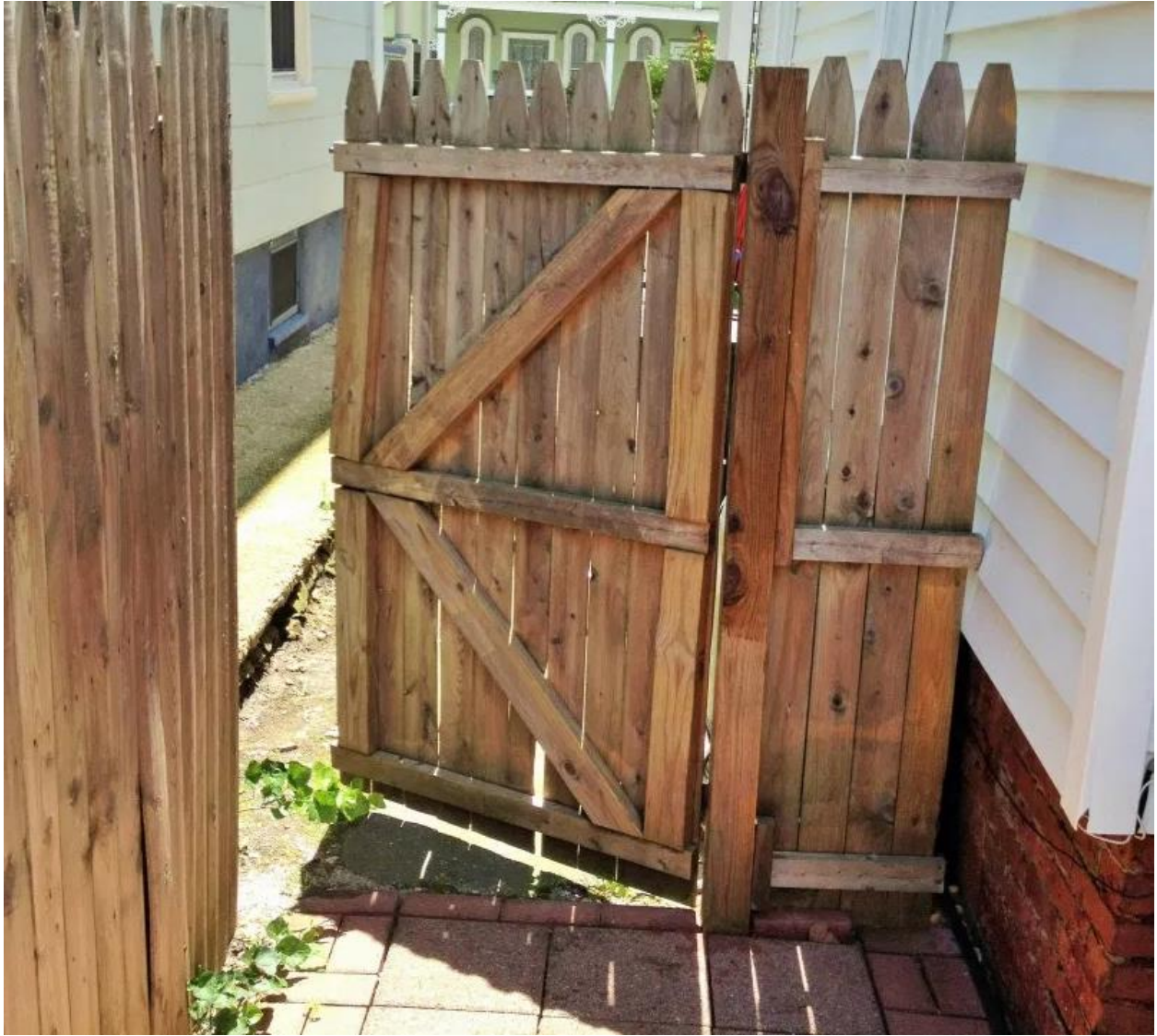
Cedar fence with gate abutting historic house (example)
