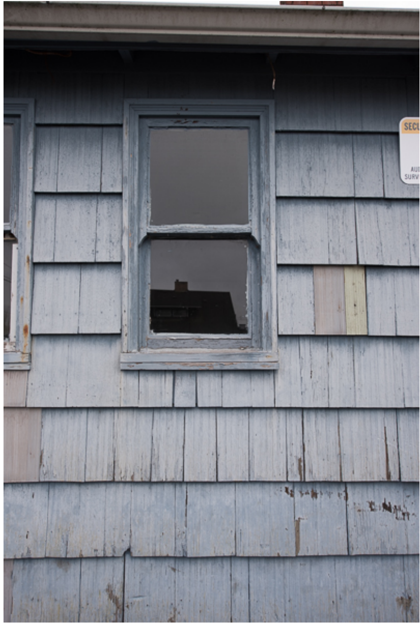
Figure 2: East Kitchen Window 4/3/2020
