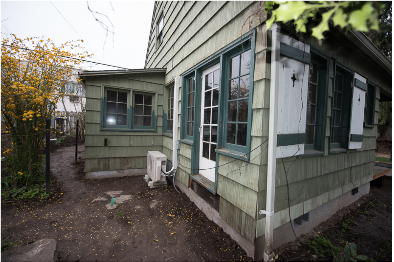
Figure 6: East Doorway and East Front Corner
