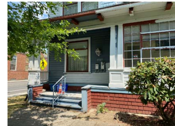
EXISTING HOUSE AND PORCH
