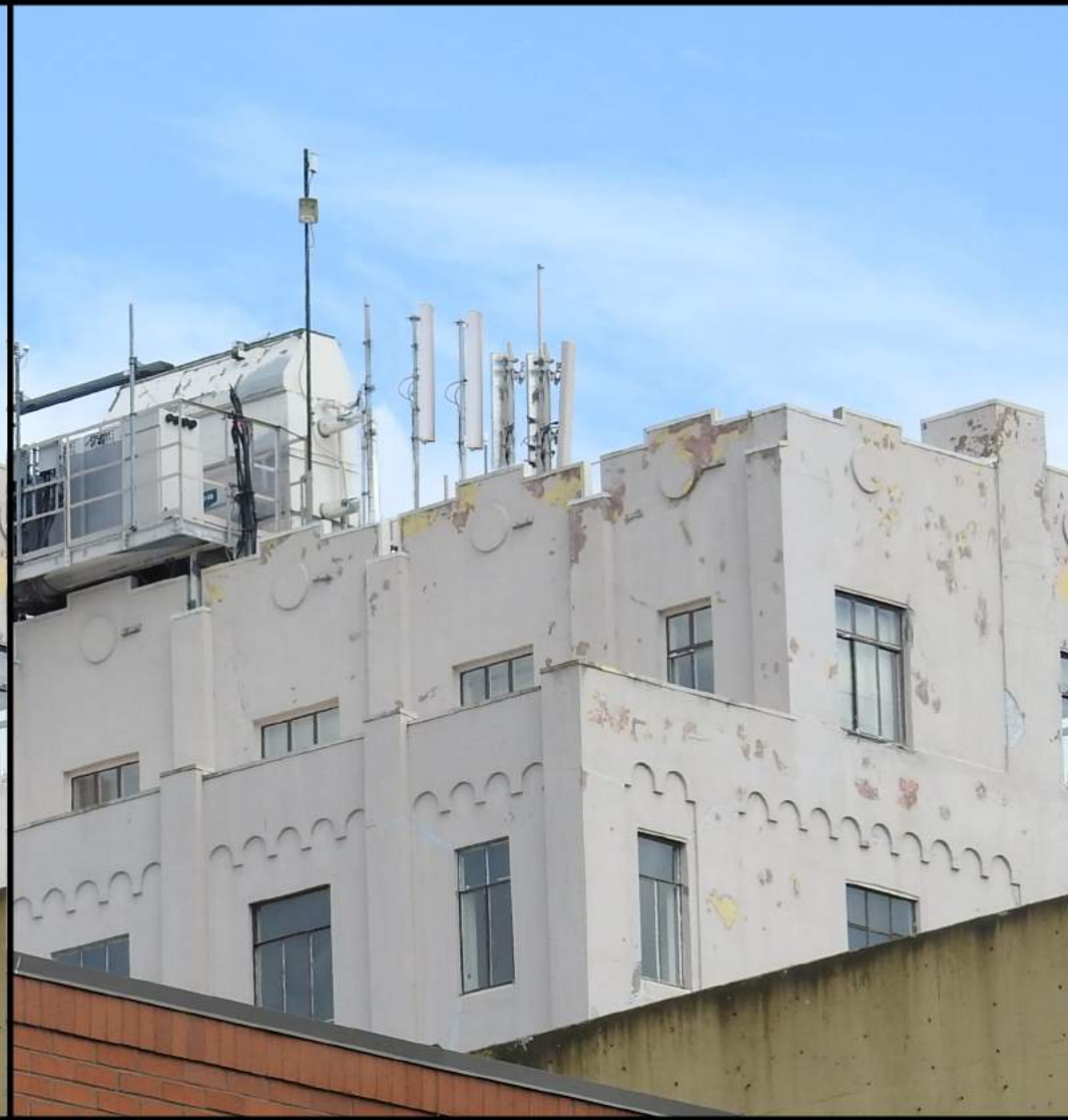
After - Looking North East
