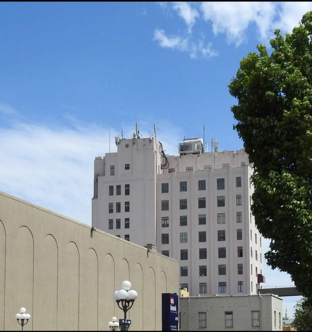
Before - Looking East
