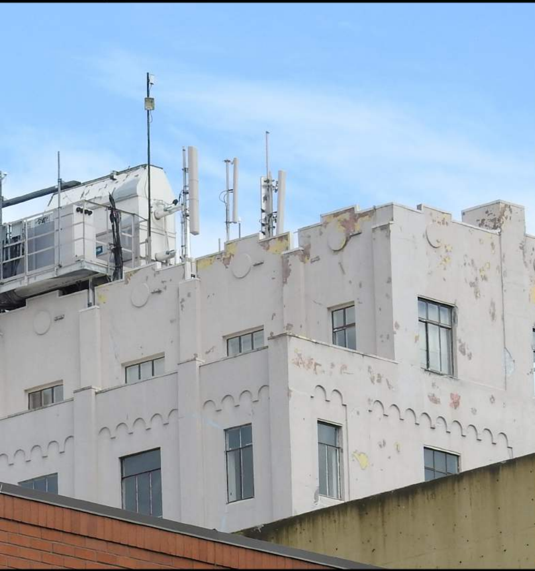
Before - Looking North East
