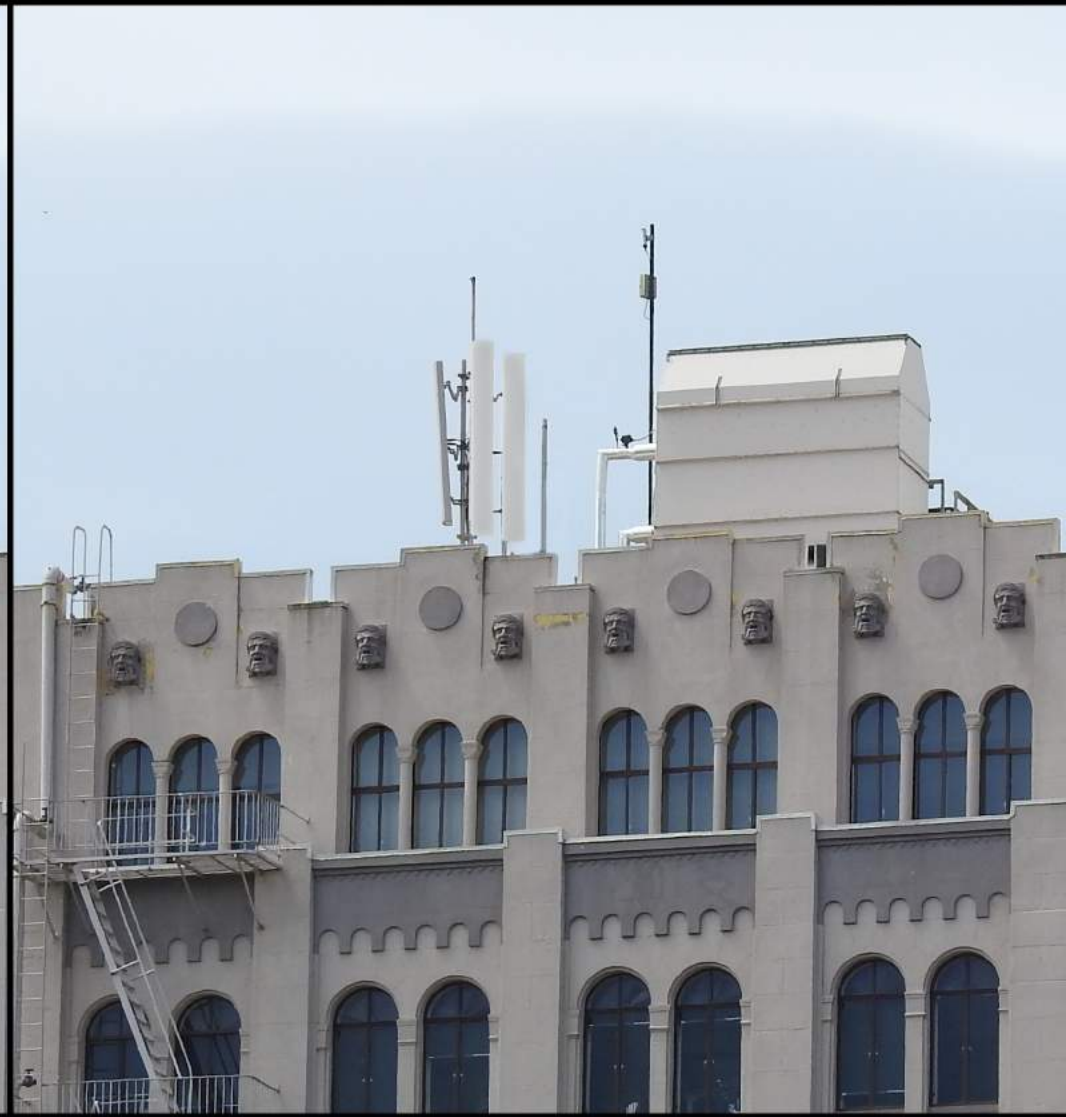
After - Looking West
