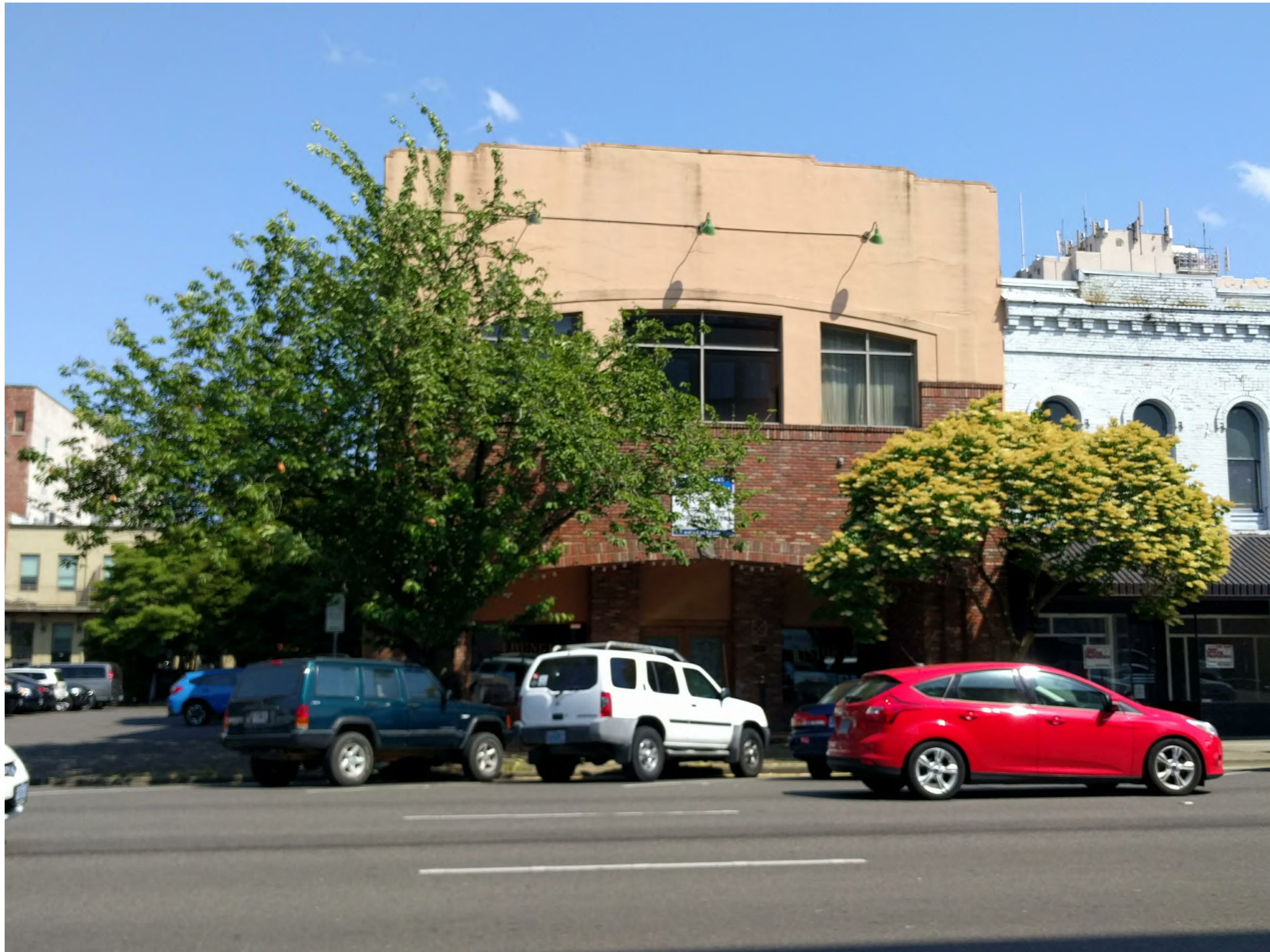
WEST BUILDING ELEVATION - VIEW FROM COMMERCIAL STREET
