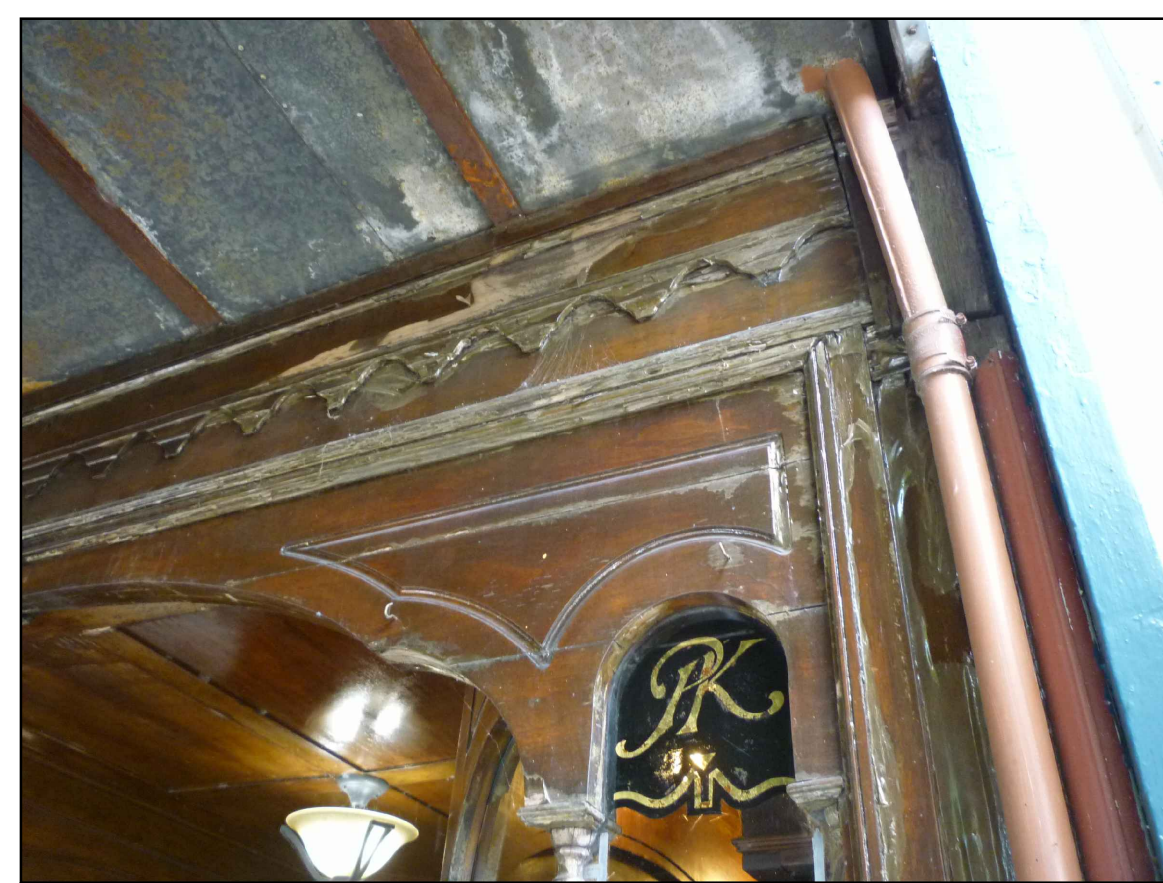
A. EXISTING WOOD PANELING AND TRIM TO BE REFINISHED. DOWNSPOUT AND CANOPY TO BE REMOVED
