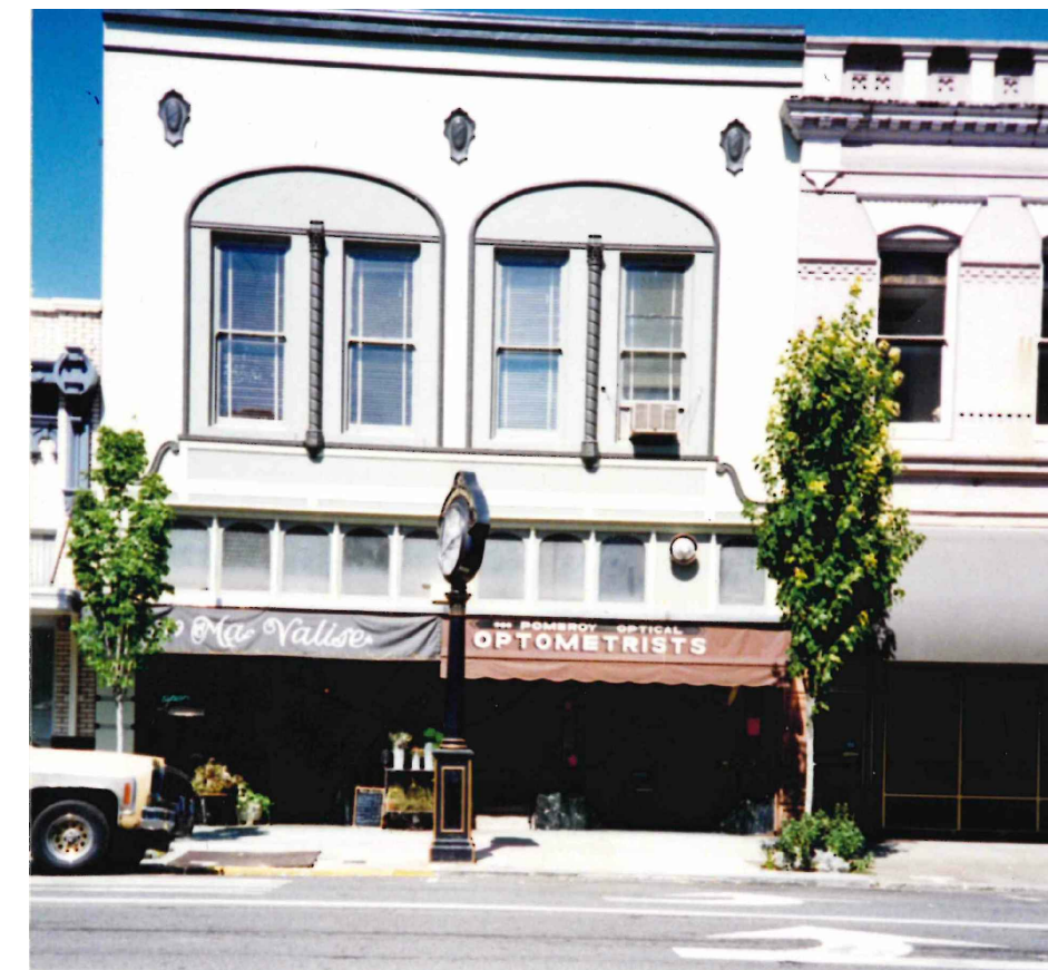
BUILDING EXTERIOR - 1980's
