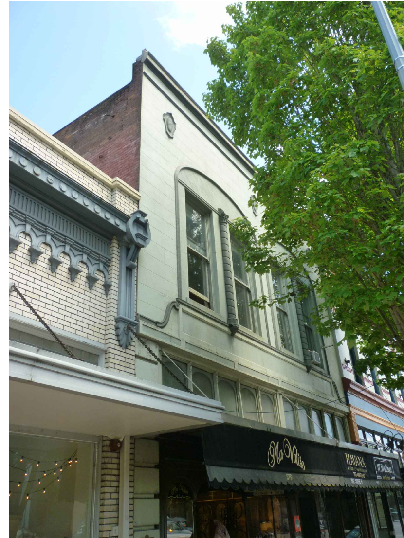
EXISTING SOUTH FACE
