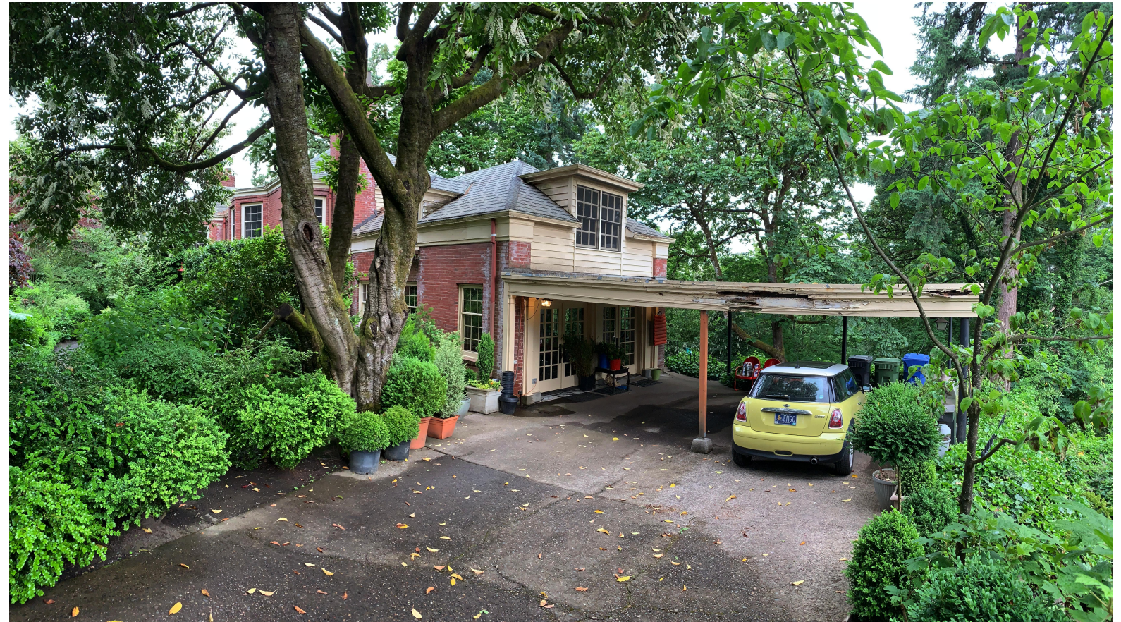
VIEW FROM DRIVEWAY
