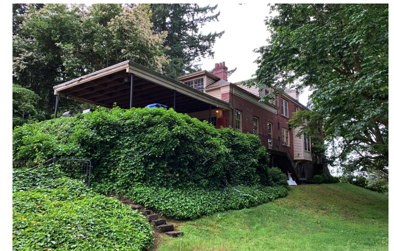
VIEW FROM NORTH-EAST
