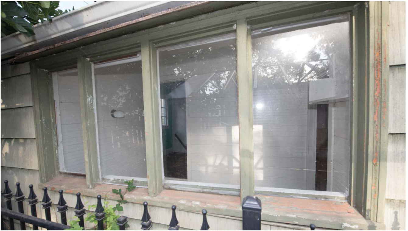
Figure 33: East Porch Windows
