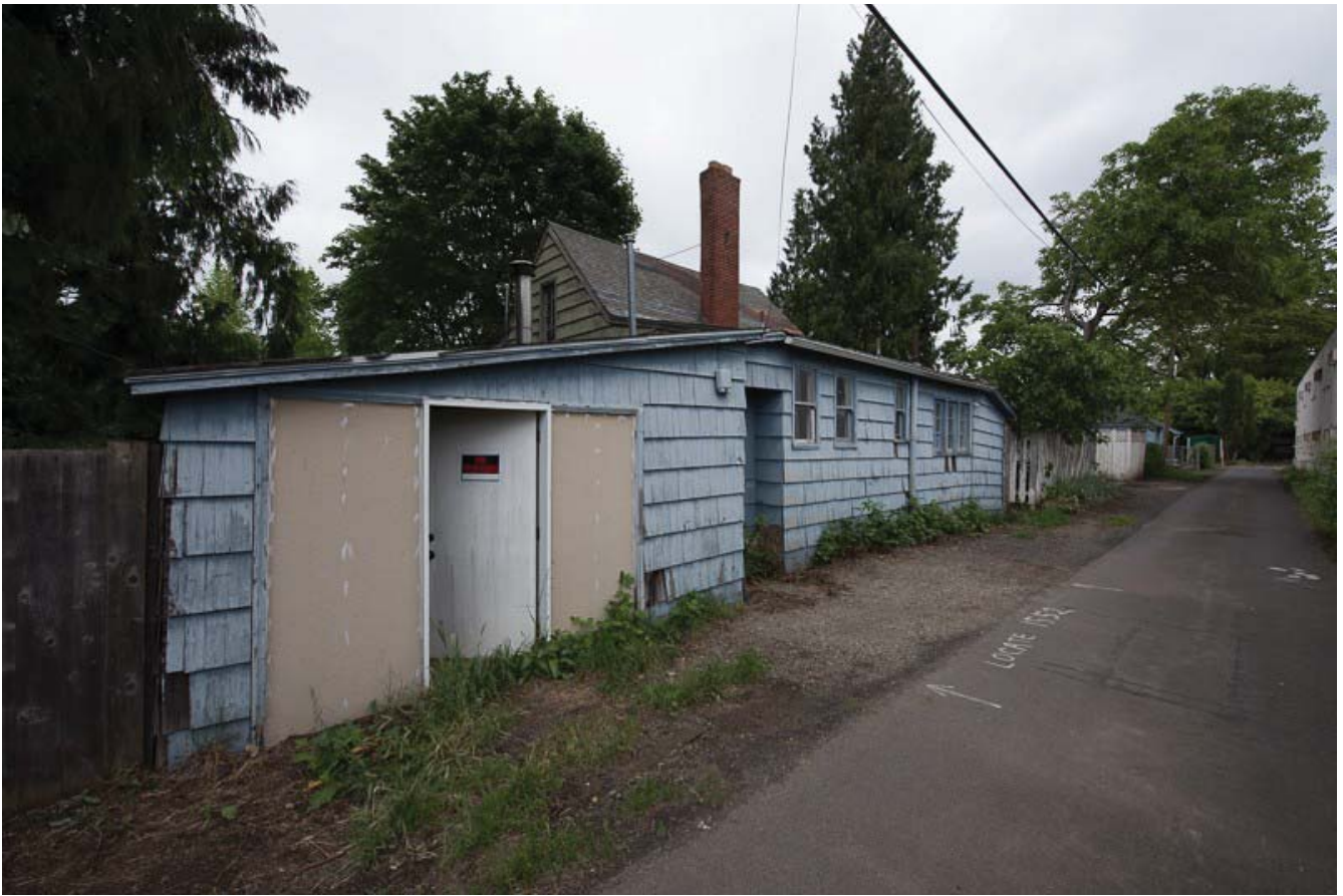
Figure 11: Garage Door Infill as of May 27, 2019
