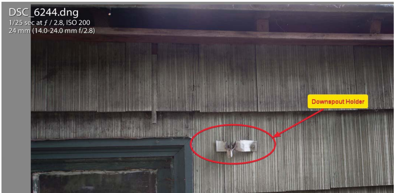
Figure 9: Garage Downspout Holder Remnant
