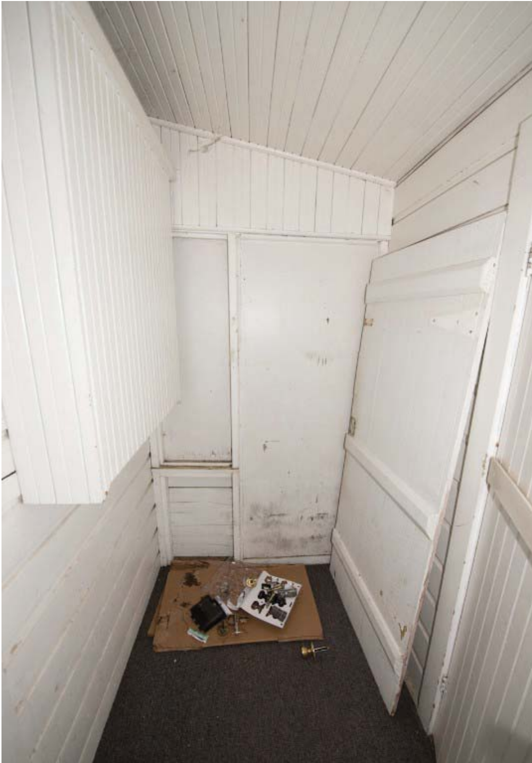
Figure 18: East Proch Inside Facing South
