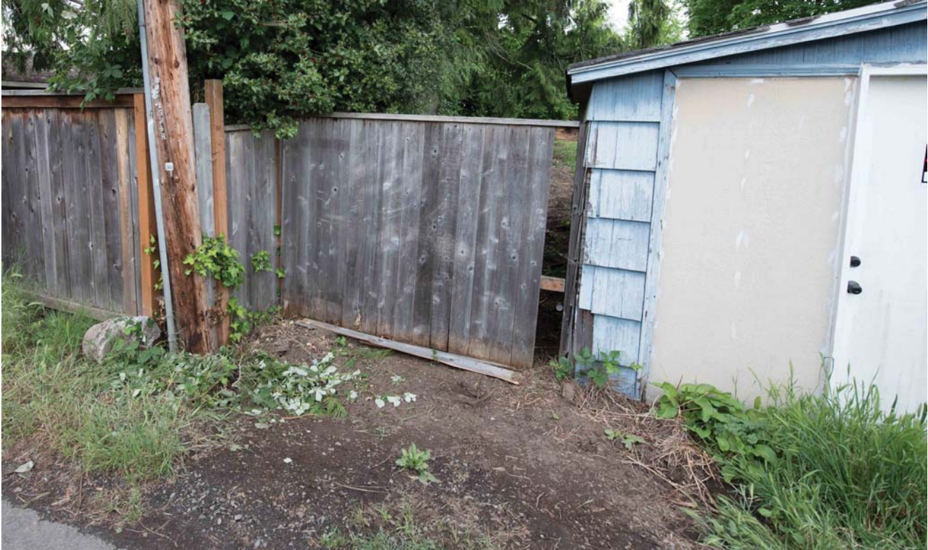
Figure 25: Western 7' Wide Fence There are two fences between the structure and the property lines facing the alley.
