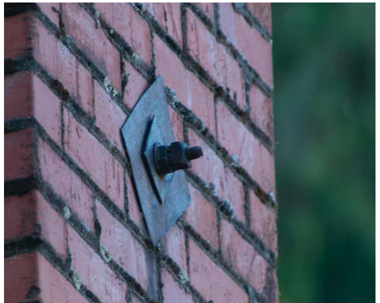
Figure 22: Chimney Brace Plate Detail
