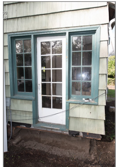
Figure 1: Eastern Façade -- October, 2019
