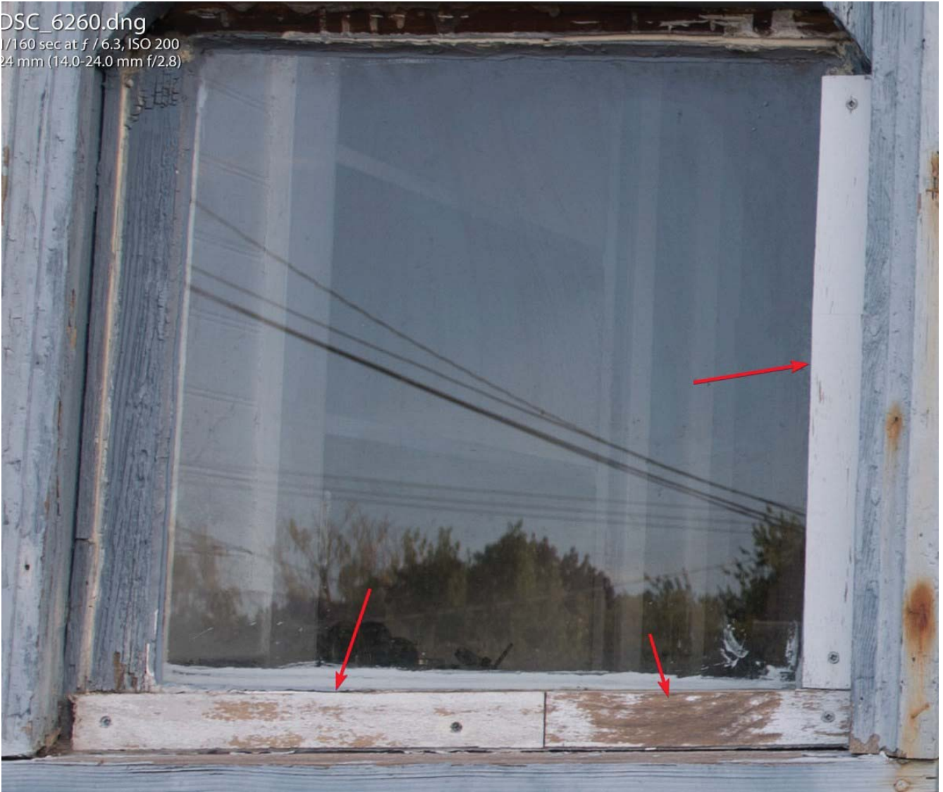
Figure 32: Kitchen Window With Sleeper Support
