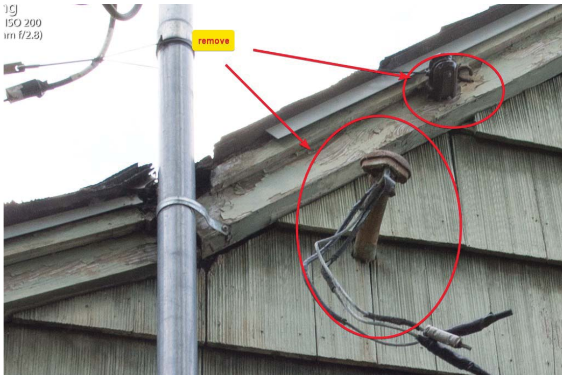
Figure 15: Prior Power Line Mast
