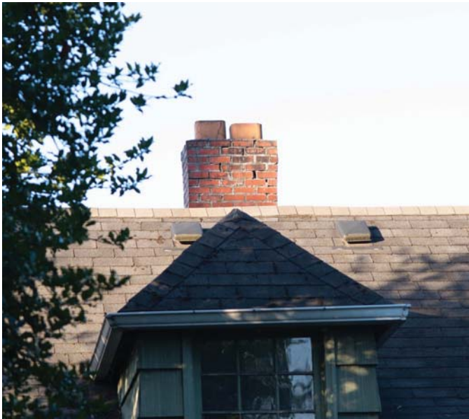
Figure 23: Chimney View Looking South Towards Front of Cottage
