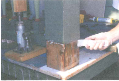
Hammering against a scrap of flooring closes the gaps
