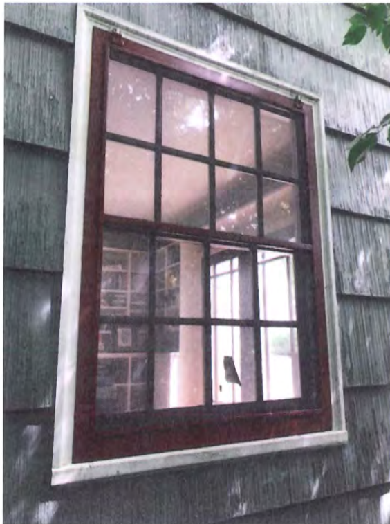
West Façade – 1 st Floor – Window 5
