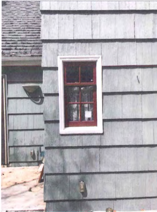
South Façade – 1 st Floor- Window 4 (Historic)
