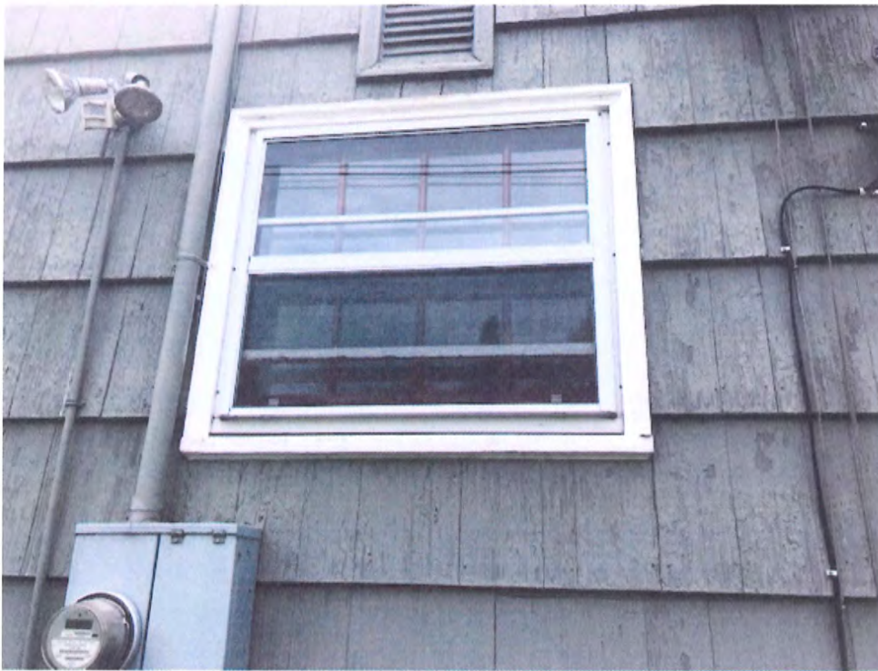
East Façade – 1 st Floor – Window 3
