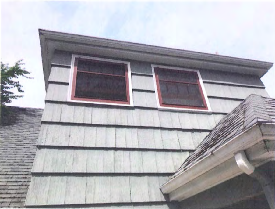
South Façade – 2 nd Floor – Window 10, 11, historic
