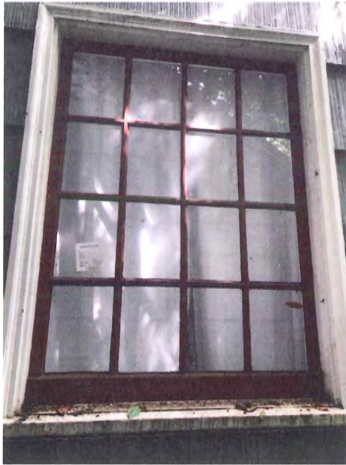
West Façade- 1 st Floor – Window 6
