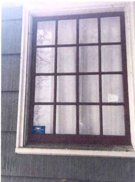
West Façade – 1 st Floor –Window 7
