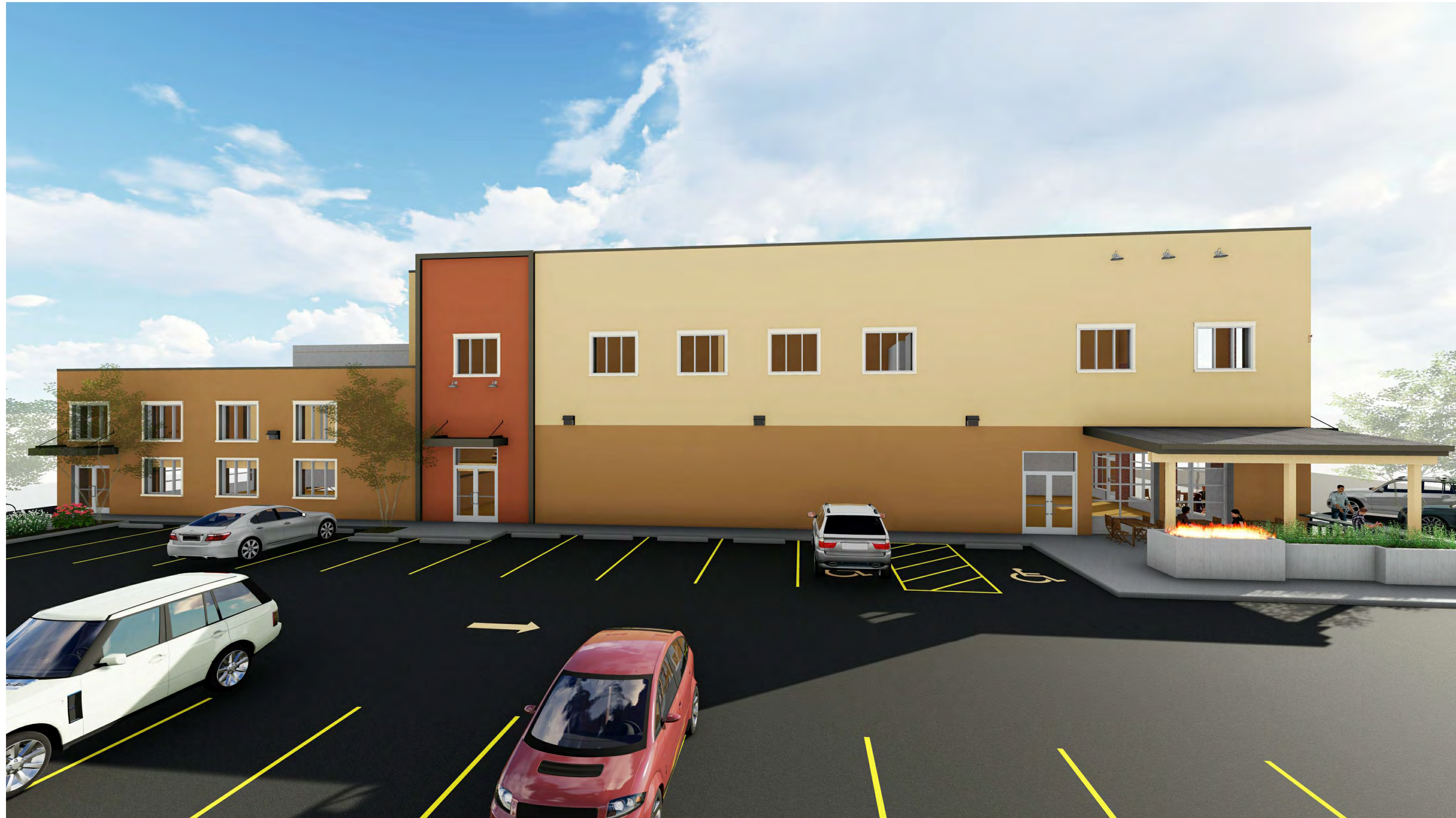
BUILDING PERSPECTIVE - VIEW FROM PARKING AREA LOOKING SOUTH
