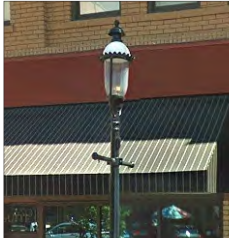
STANDARD PEDESTRIAN LIGHT POLES (APPROXIMATELY EVERY 90 FEET)
