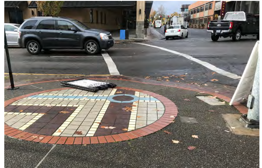
Remnants of previous streetscape project
