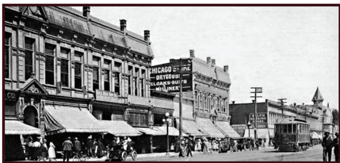
Bush-Breyman Block and Bush and Brey Block buildings on Commercial Street, looking toward the Court Street intersection.
