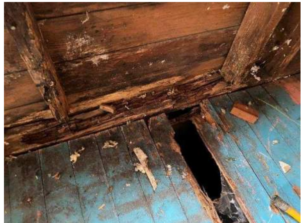
Photo 12: Floor Deterioration
