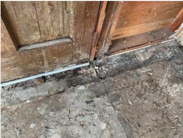
Photo 5: Floor Deterioration
