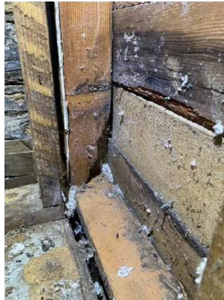
Photo 10: Wall Damage
