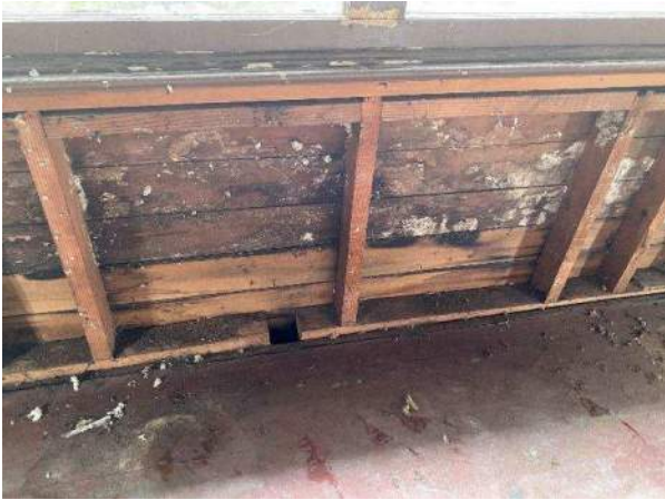
Photo 3: Sheathing Damage
