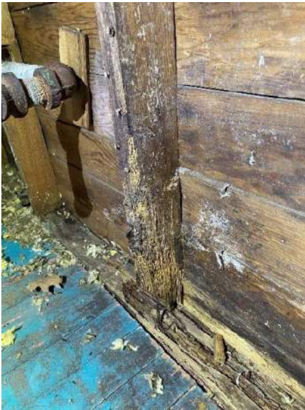
Photo 9: Stud Damage
