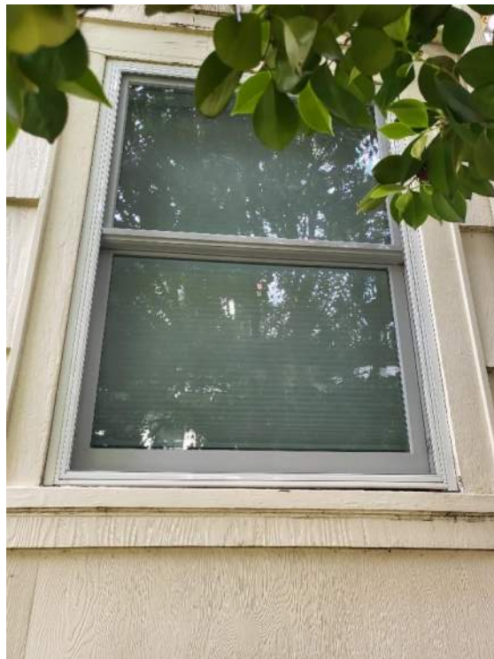
New windows on secondary façade(east)—replaced- not subject to review
