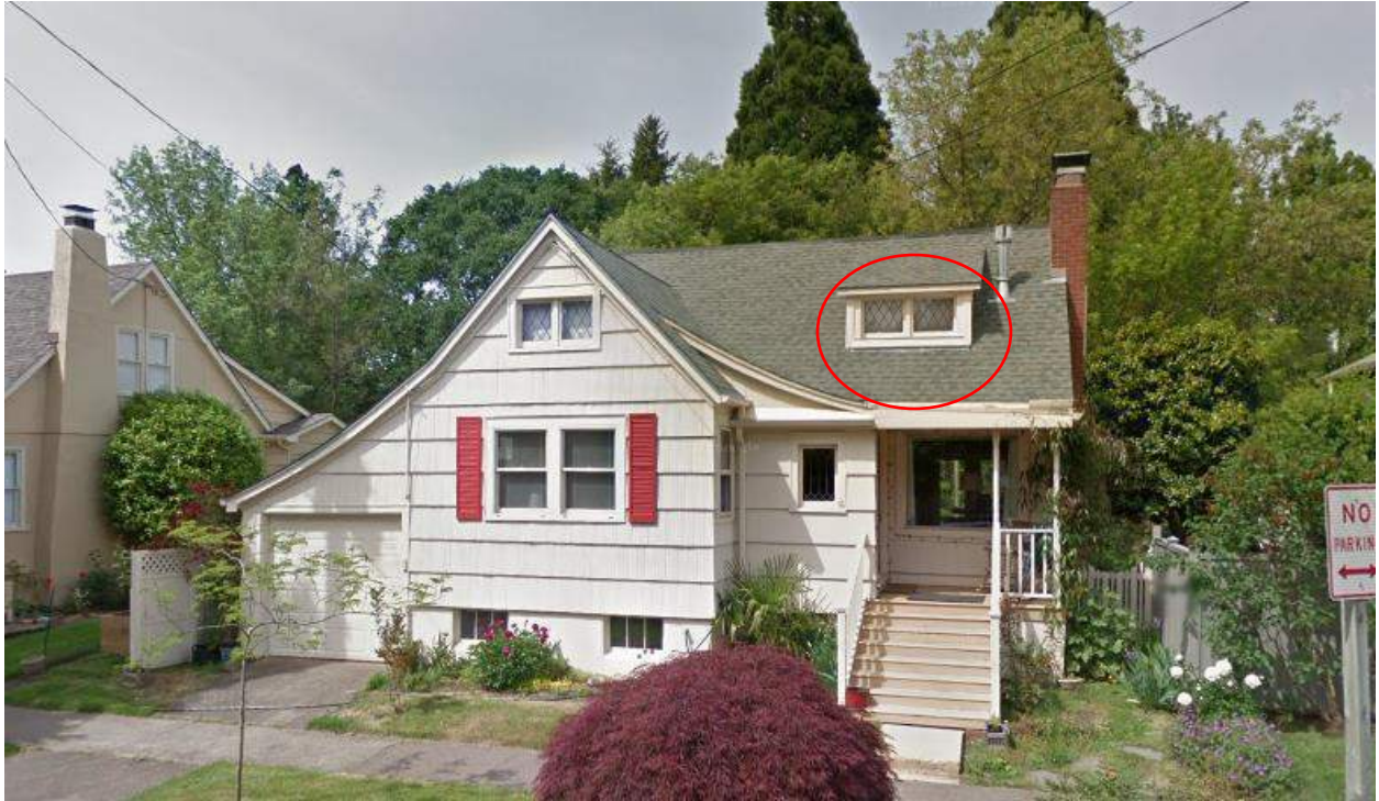
Primary Façade of Jeanette Pooler House (1920) NC to Court Chemeketa District
