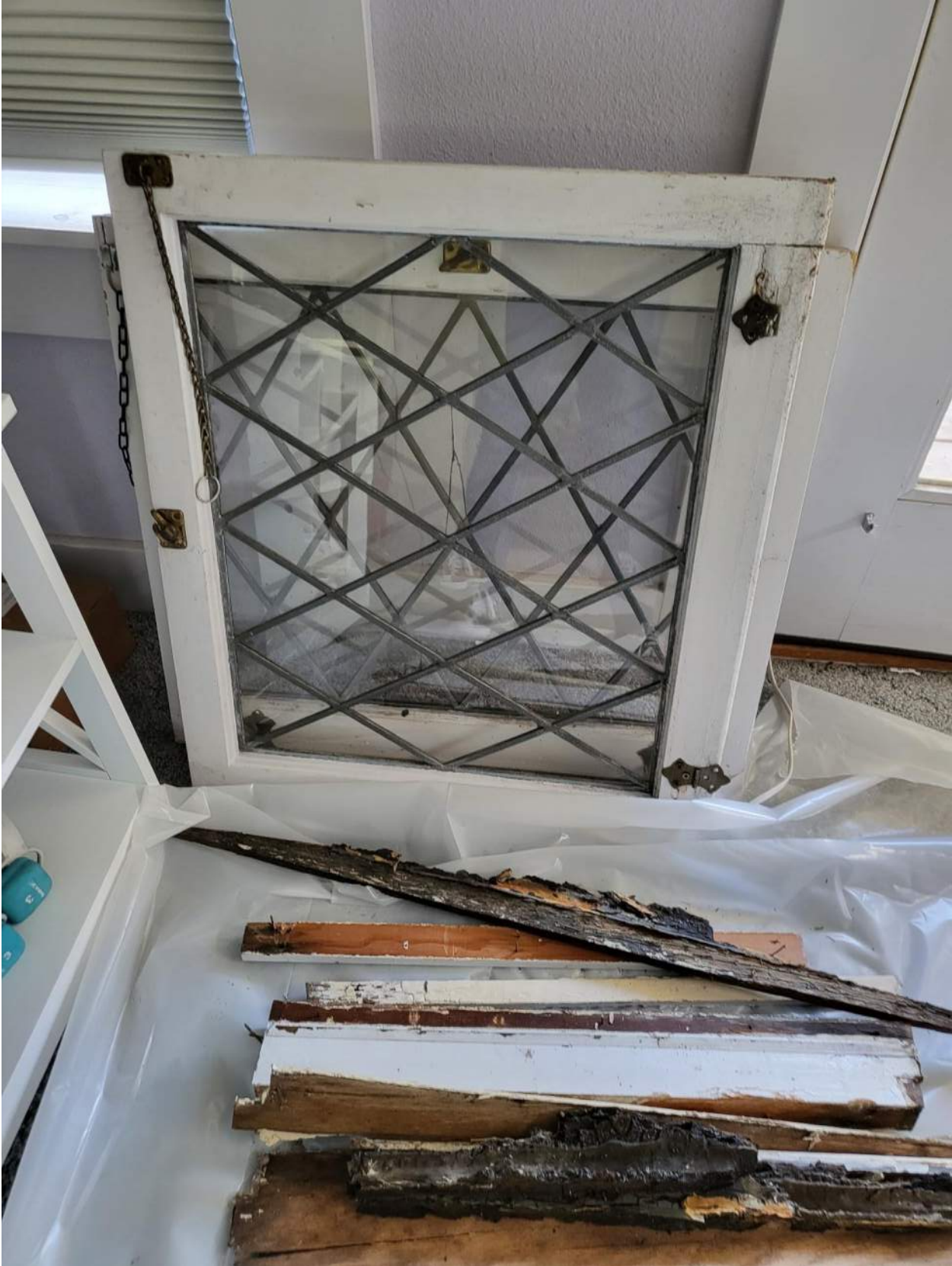
Existing window removed from frame
