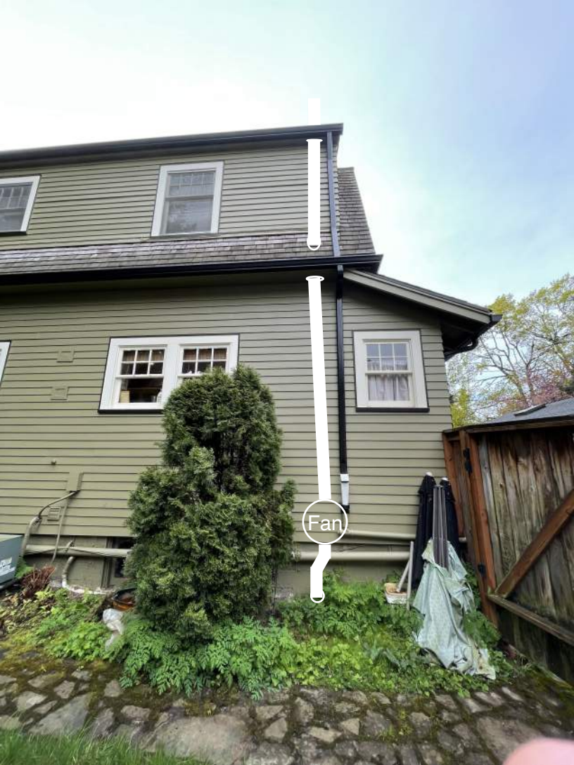
Approximation of residence with radon Mitigation system installed.
