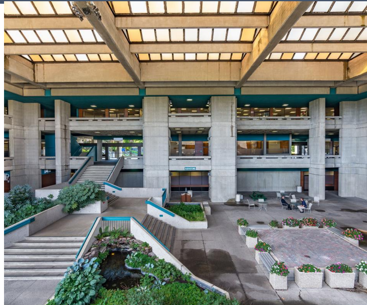
Salem Civic Center Atrium
