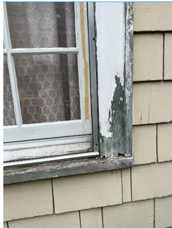
East Elevation: Chimney with Window detail (showing corner/bottom sill in need of repair)
