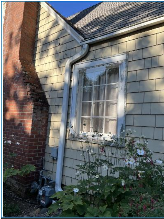
East Elevation: Chimney with Window detail (showing corner/bottom sill in need of repair)
