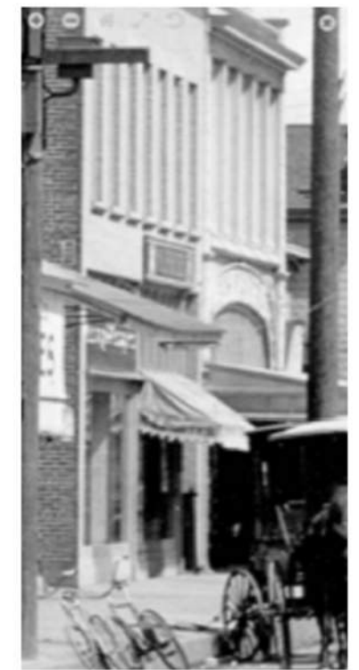
HISTORIC SOUTH ELEVATION
