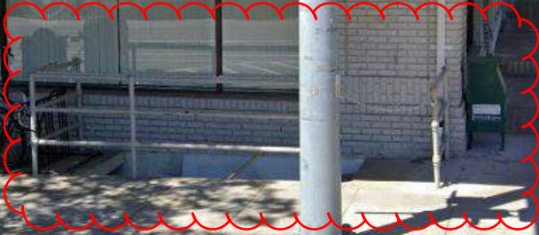
VIEW OF STAIRS FROM HIGH STREET
