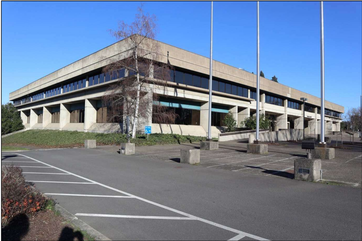
Photo 17 of 40. City Hall west and south elevations, looking northeast.
