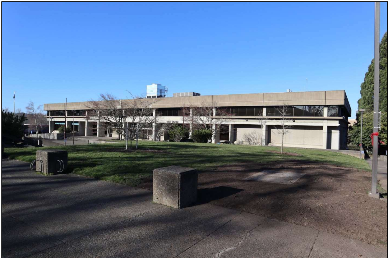
Photo 18 of 40. City Hall south elevation, looking northwest.
