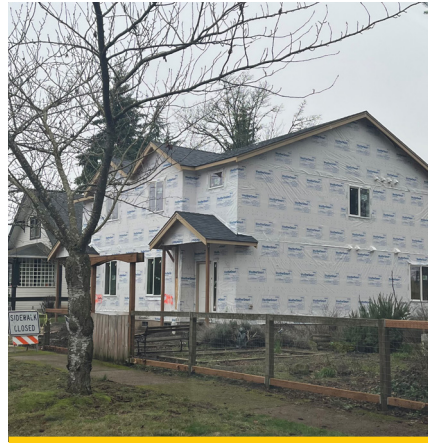
Figure 9 Two of the four units at 2140 Trade St SE
