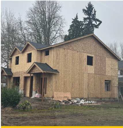
Figure 8 Two of the four units at 2140 Trade St SE
