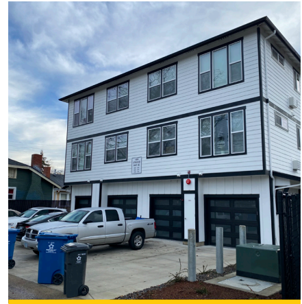
Figure 10 New six-plex at 488 Strand Ave SE
