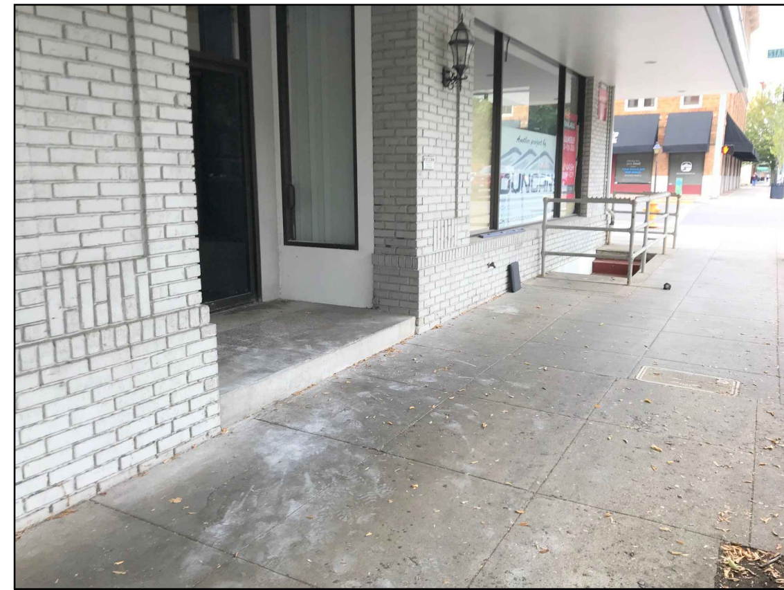
2 105 HIGH STREET ENTRANCE - EXISTING SCALE: NTS
