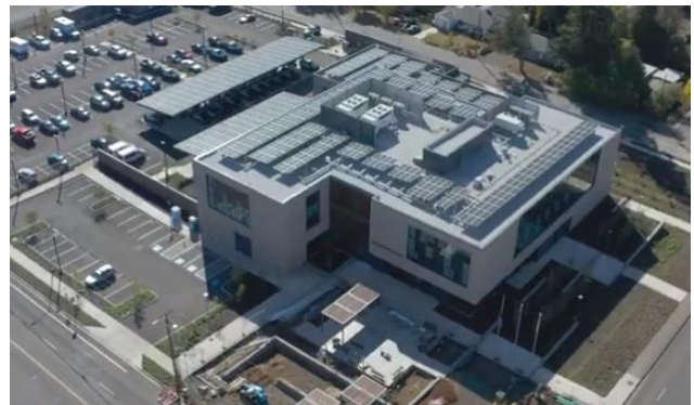
The Beaverton Public Safety Center has a backup power system that includes a generator, solar energy, and a battery energy storage system.
