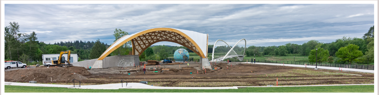
Gerry Frank | Salem Rotary Amphitheater under construction (2021)
