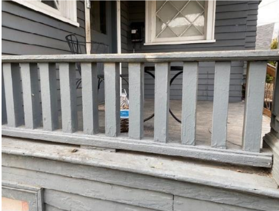
Photo #1: Existing Condition: Front Porch looking west
