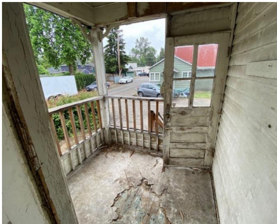
Photo # 8: Existing Condition – interior of rear porch (southeast corner)
