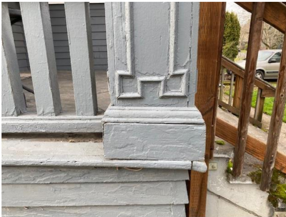
Photo #2: Existing Condition: Front Porch column detail
