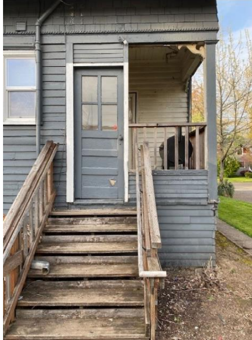
Photo #5: Existing Condition – Detail of porch -rear (south) façade of Hewitt House – looking north
