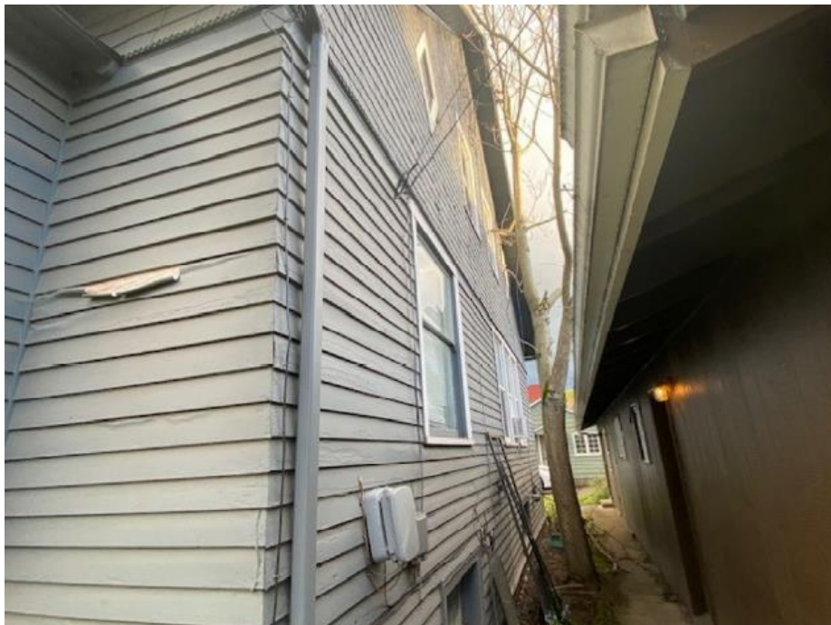
Photo#10: Existing Condition- West Façade looking south
