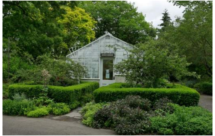
Buildings and Structures: Greenhouse (Conservatory) in 2020
