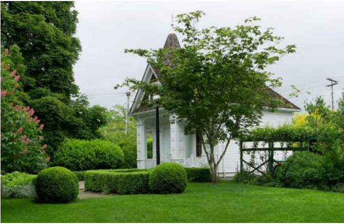
Buildings and Structures: Deepwood Carriage House in 2020
