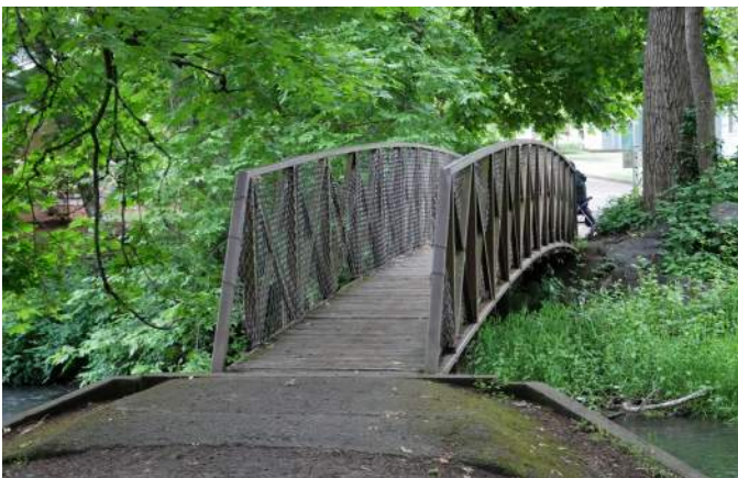
Buildings and Structures: Pringle Creek Bridge at Waller Street in 2020
