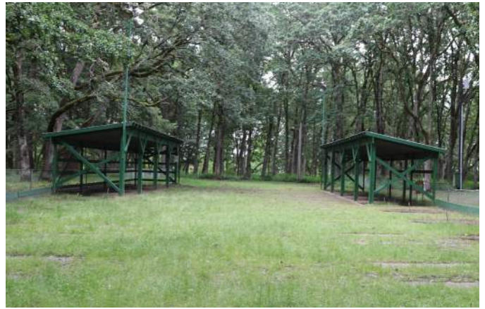
Buildings and Structures: Horseshoe Courts in 2020
