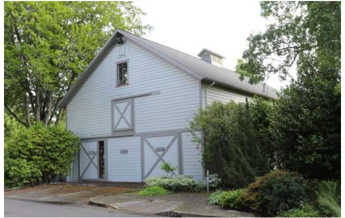
Buildings and Structures: Bush Barn Art Center in 2020
