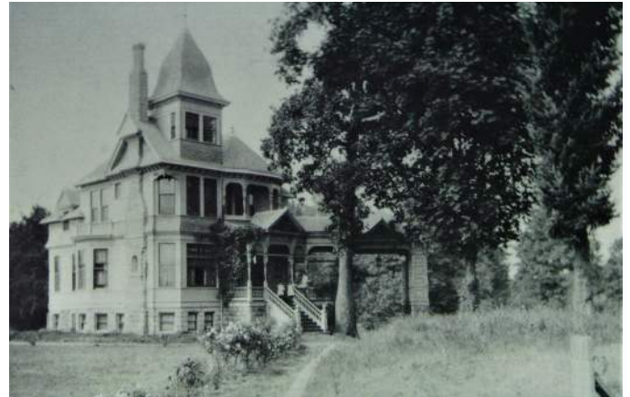
Vegetation: (undated photograph) Deepwood Entry Garden (source unknown)
