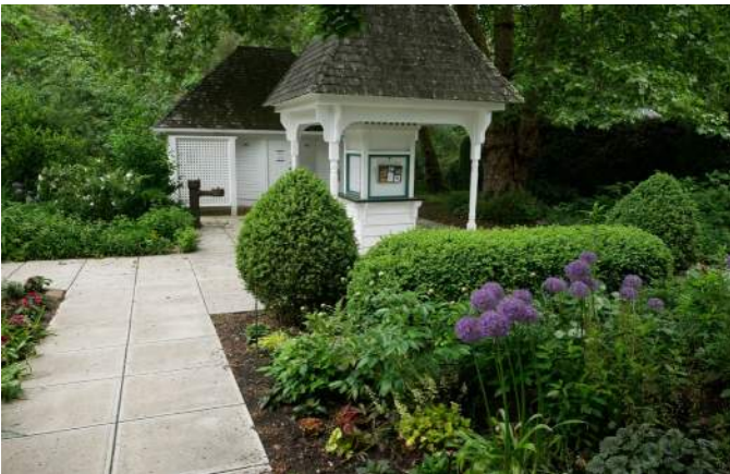
Buildings and Structures: Deepwood Restroom and Kiosk in 2020
