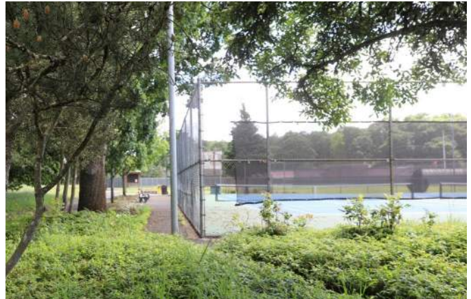
Buildings and Structures: Bush's Pasture Park Tennis Courts in 2020
