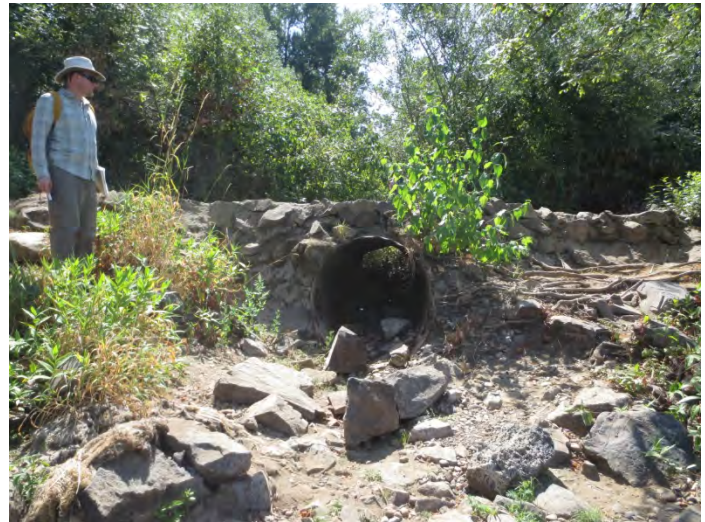
Oxbow Slough culvert
