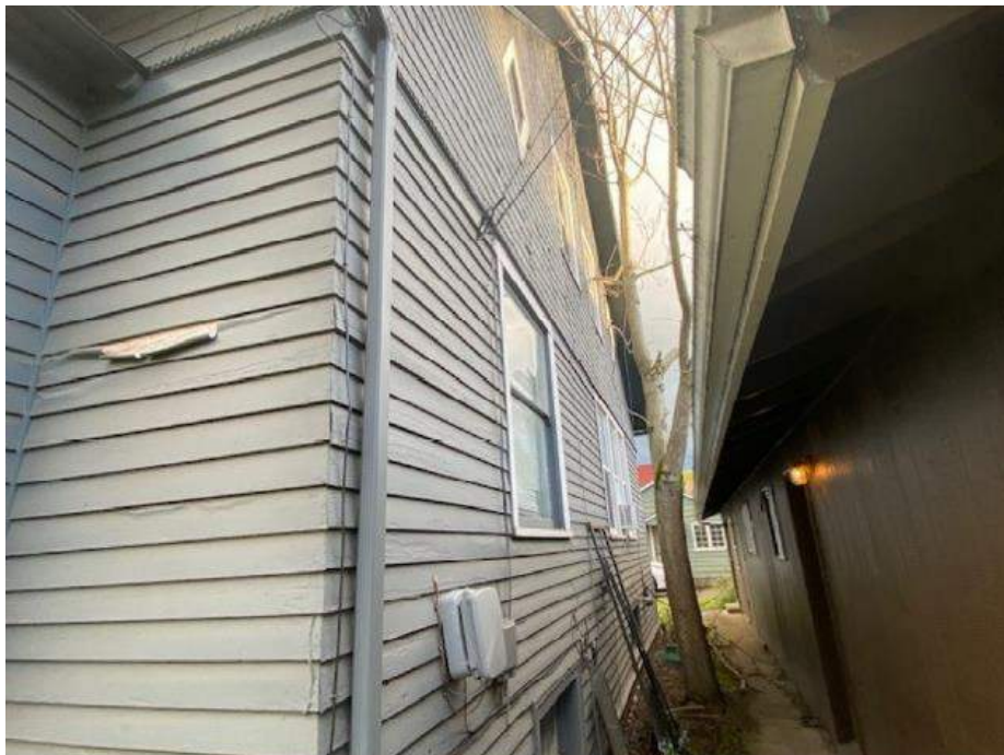
Photo#10: Existing Condition- West Façade looking south
