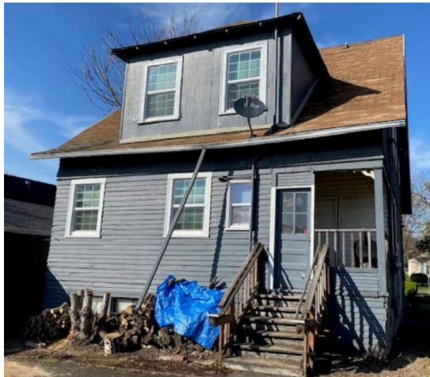
Photo #4: Existing Condition – rear (south) façade of Hewitt House – looking north
