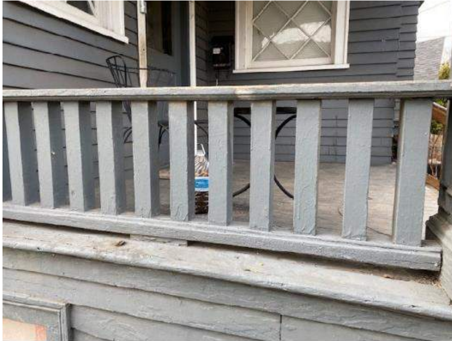
Photo #1: Existing Condition: Front Porch looking west
