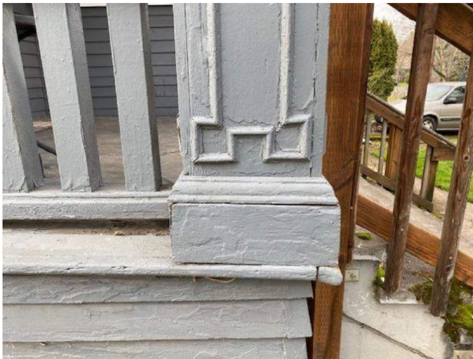
Photo #2: Existing Condition: Front Porch column detail
