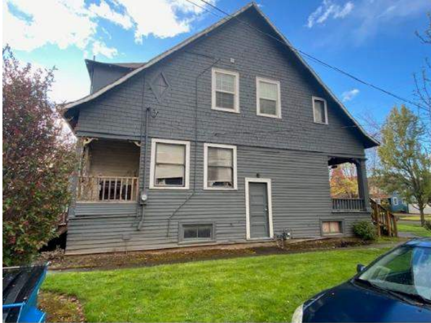
Photo #3: Existing Condition siding/porches – East Façade of Hewitt House – looking northwest
