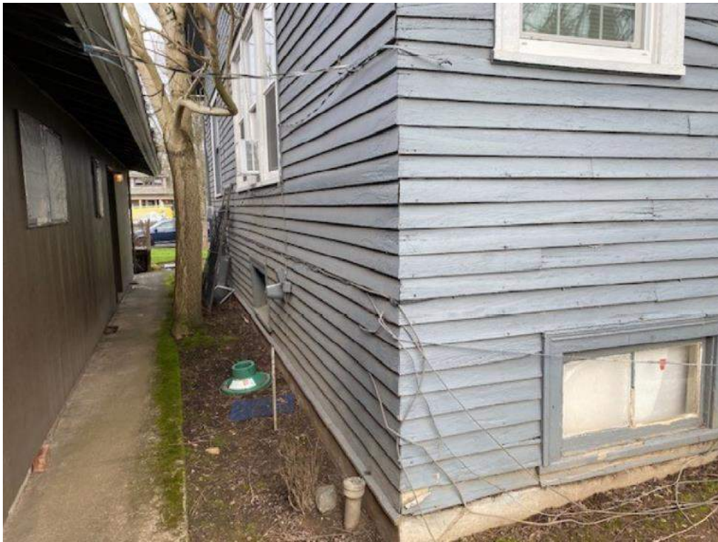
Photo#11: Existing Condition- West Façade looking north
