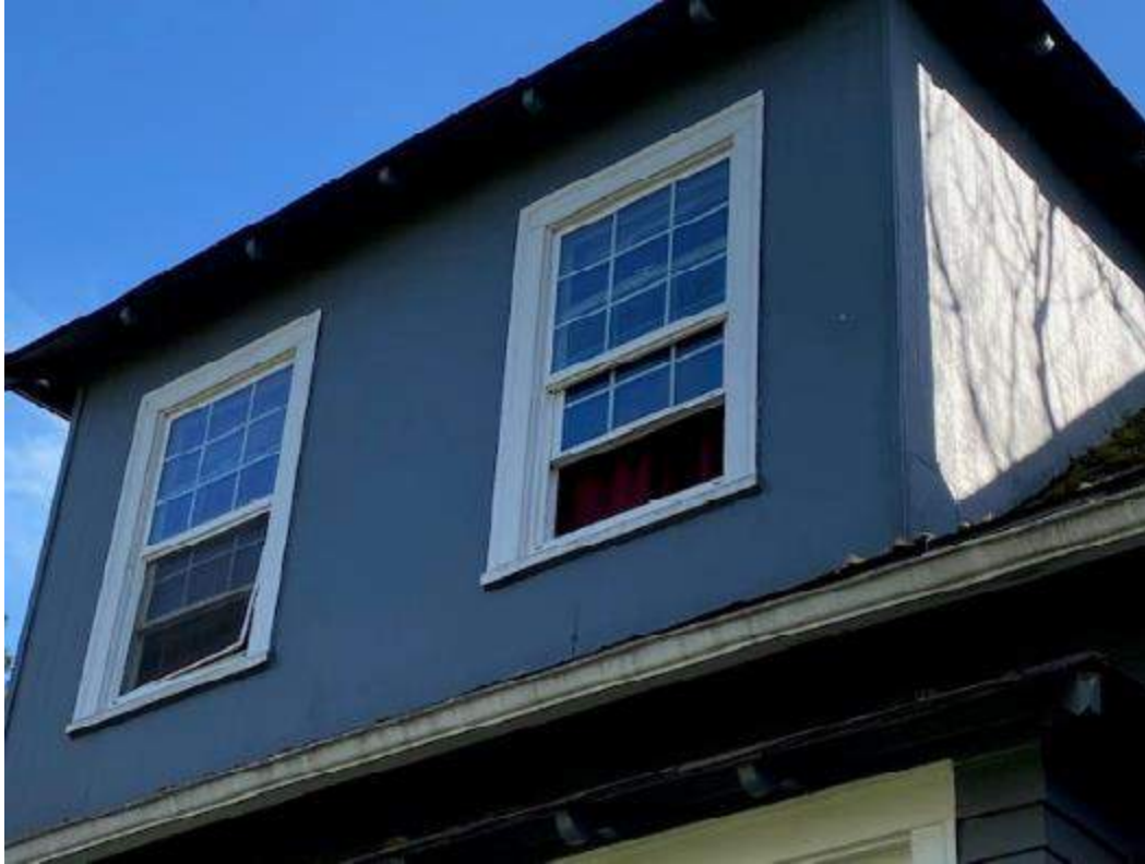
Photo#9: Existing Condition- Detail Rear Dormer (south façade)- looking north
