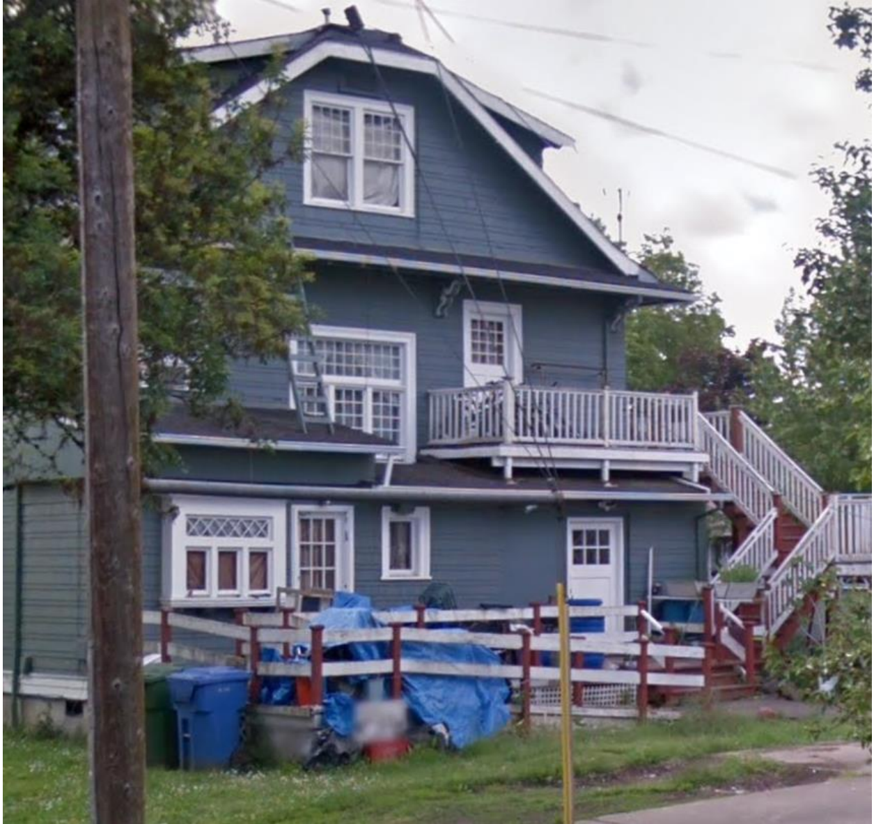
Existing Deck – Rear (West) Façade- 2 nd story
