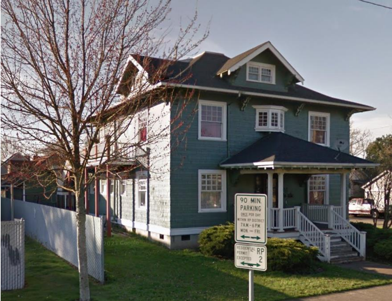
Existing deck- Secondary Façade (South)
