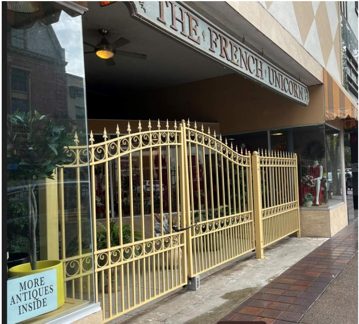
Installed gate- 170 Liberty Street NE
