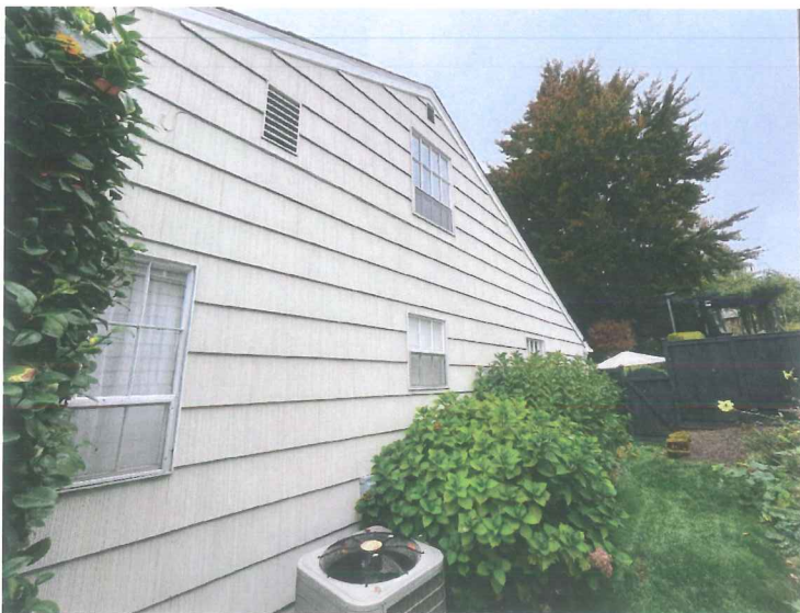
Figure 2 – Photo of East façade
