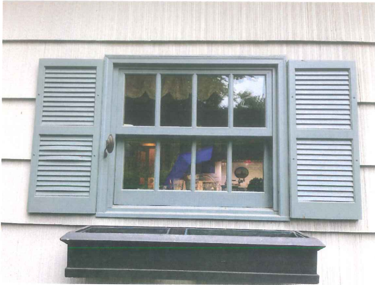
Figure 5 – Photo of kitchen window on back (north) side of house (Marvin Ultimate Wood Double Hung Simulated Divided Lite)
