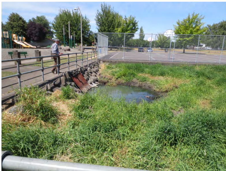
Figure 7. Claggett Creek Outfall
