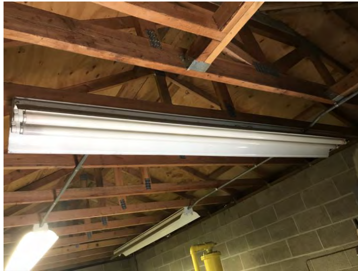
Figure 3.18 Light Fixtures without Lens Covers
