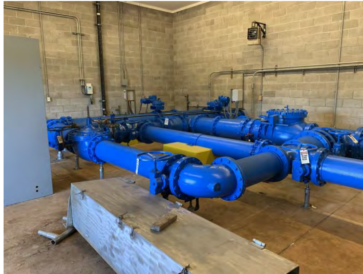
Figure 3.172 Unbraced Piping and Valves
