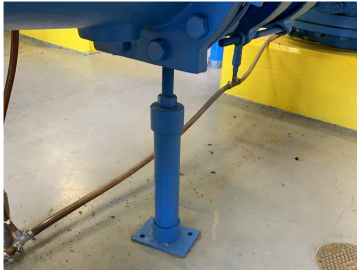
Figure 3.89 Pipe Support Stanchion Missing Anchors into Floor Slab
