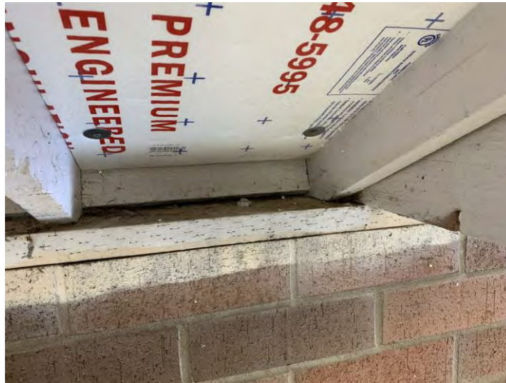
Figure 3.51 Inadequate Connection between Blocking and Masonry Wall Top Plate
