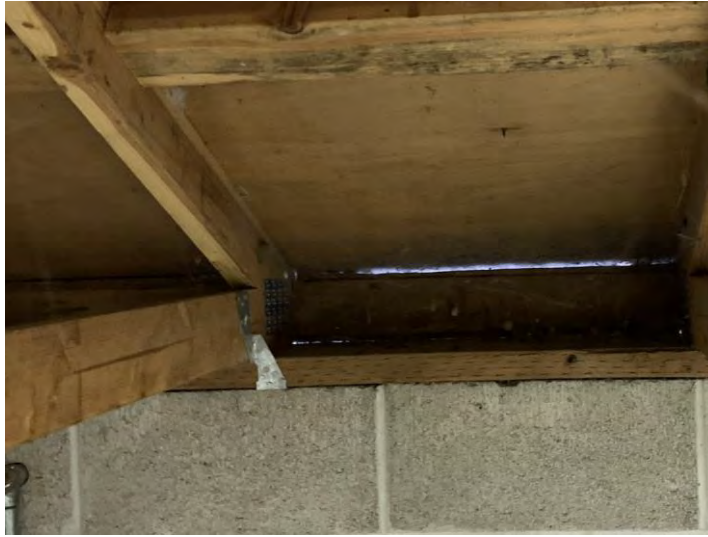
Figure 3.14 Roof Truss to Masonry Wall Top Plate Connection
