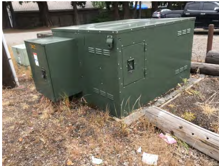
Figure 3.111 Unanchored Electrical Transformer
