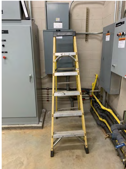
Figure 3.192 Unrestrained Step Ladder
