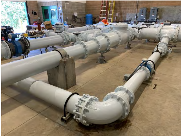
Figure 3.200 Unbraced Piping and Valves
