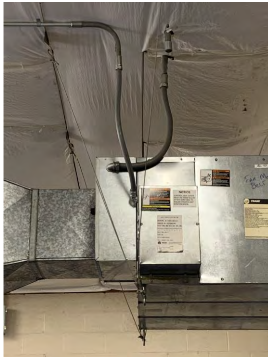
Figure 3.189 Suspended HVAC Unit
