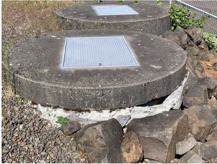
Figure 3.146 Concrete Deterioration at Lid to Wall Connection of South Valve Vault
