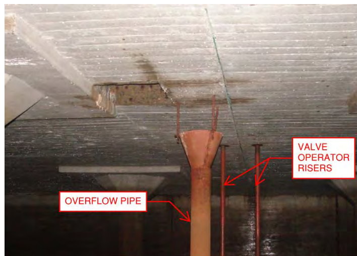
Figure 3.128 Overflow Pipe and Valve Operator Risers Not Adequately Braced (Source: 2011 Reservoir Condition Assessment by Murray, Smith & Associates)
