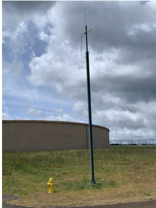
Figure 3.141 SCADA Antenna
