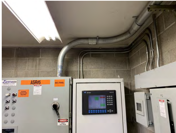
Figure 3.27 Conduit Top Connection to Motor Control Center without Flexible Connection
