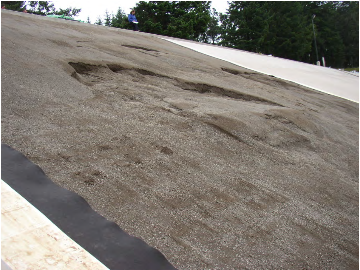
Exhibit 3-21: Photo of Slump Failure along Cut Slope of West Cell from 2008 (Photo Provided by the City of Salem)
