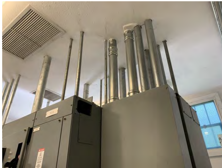
Figure 3.64 Conduits Connecting to Electrical Cabinets without Flexible Connections
