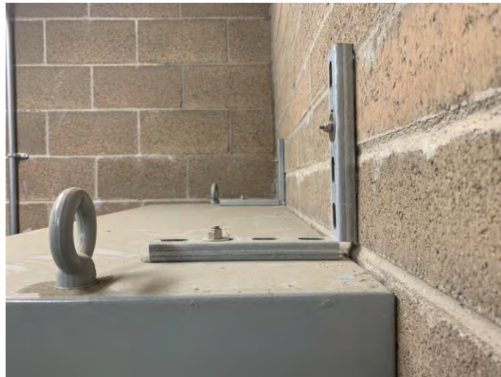
Figure 3.109 Anchorage at Electrical Cabinet with Bent Strut
