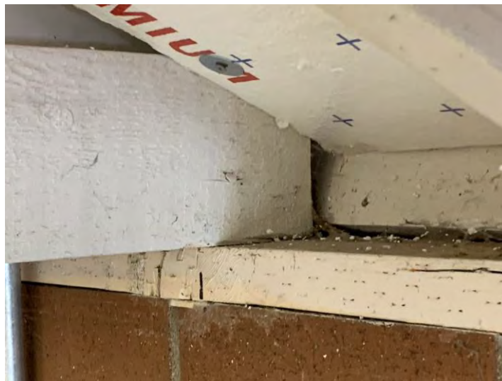
Figure 3.52 Inadequate Connection between Truss Chord and Masonry Wall Top Plate
