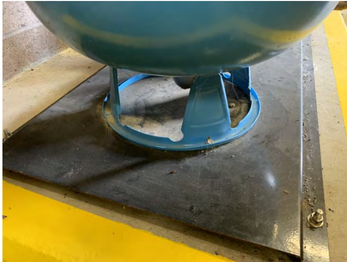
Figure 3.139 Irrigation Pressure Tank Missing Anchor
