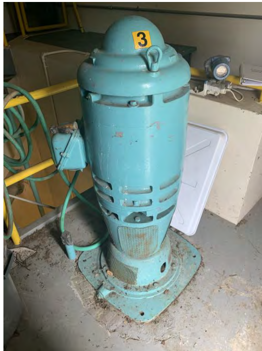
Figure 3.160 Unanchored Pump
