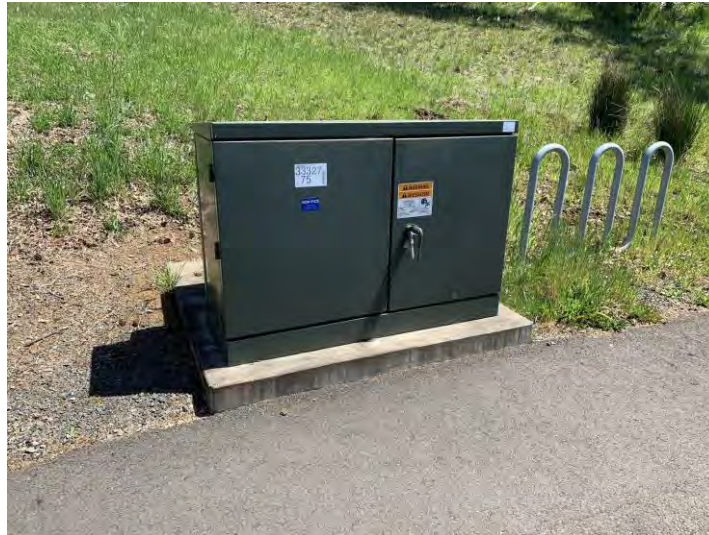
Figure 3.208 Unanchored Electrical Transformer
