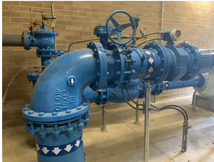
Figure 3.106 Unbraced Piping and Valves
