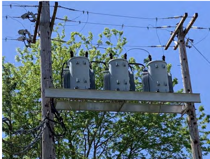
Figure 3.71 Pole-Mounted Electrical Transformers
