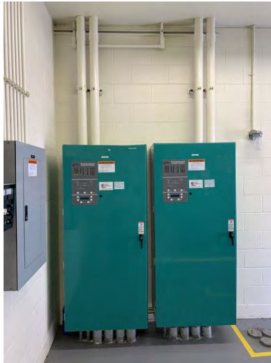
Figure 3.95 Conduits Connecting to Electrical Cabinets without Flexible Connections
