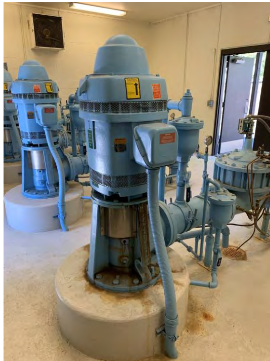
Figure 3.79 Unbraced Pump Motor
