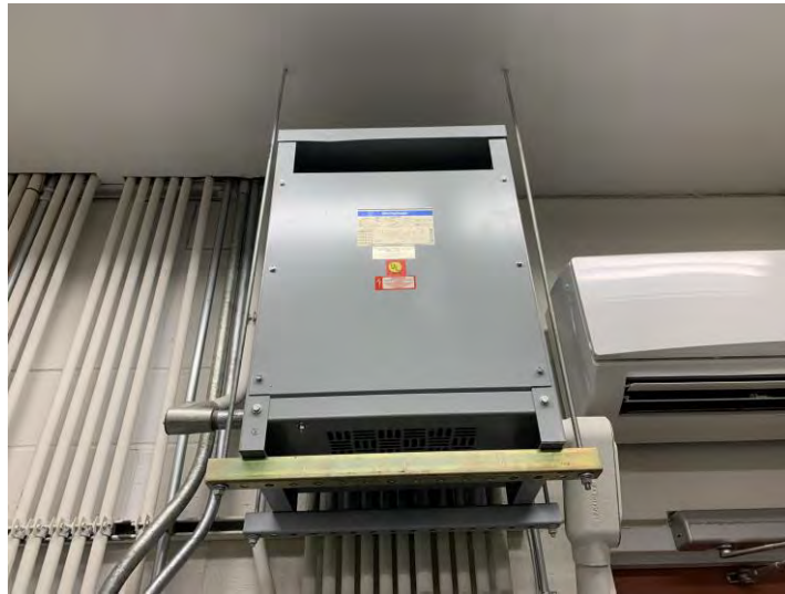
Figure 3.93 Unbraced Elevated Electrical Transformer
