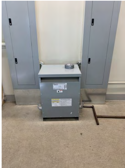
Figure 3.118 Electrical Transformer Missing Anchors into Floor Slab
