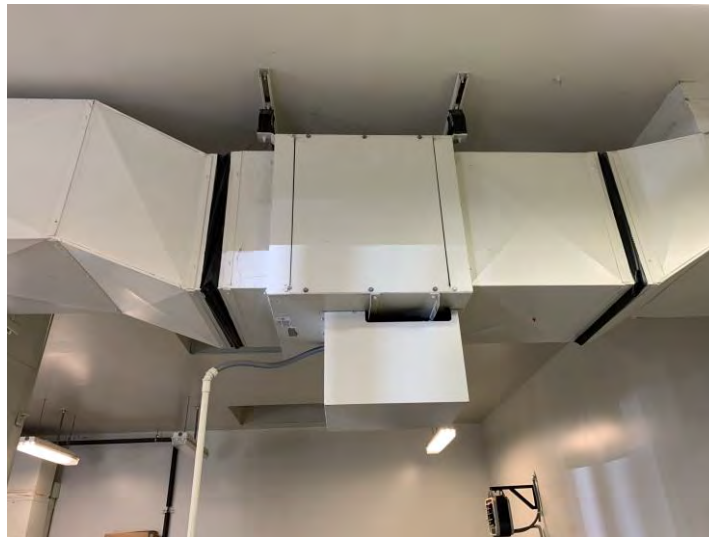
Figure 3.123 Unbraced Inline Fan Unit
