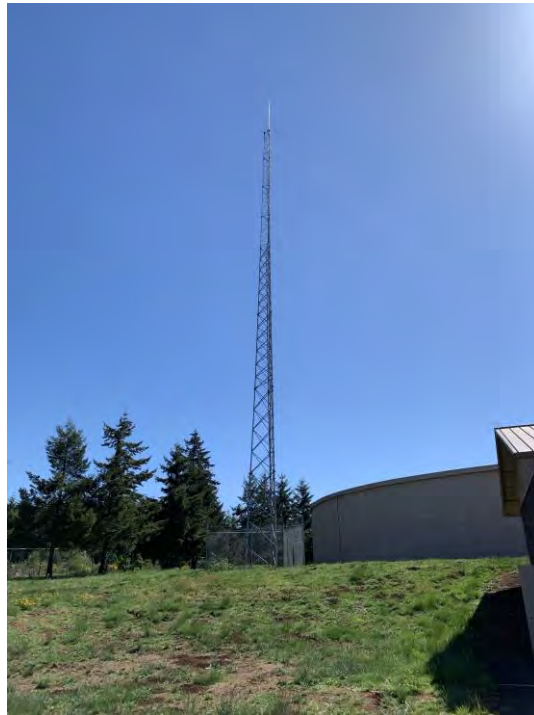
Figure 3.168 SCADA Antenna Supported by Lattice Tower
