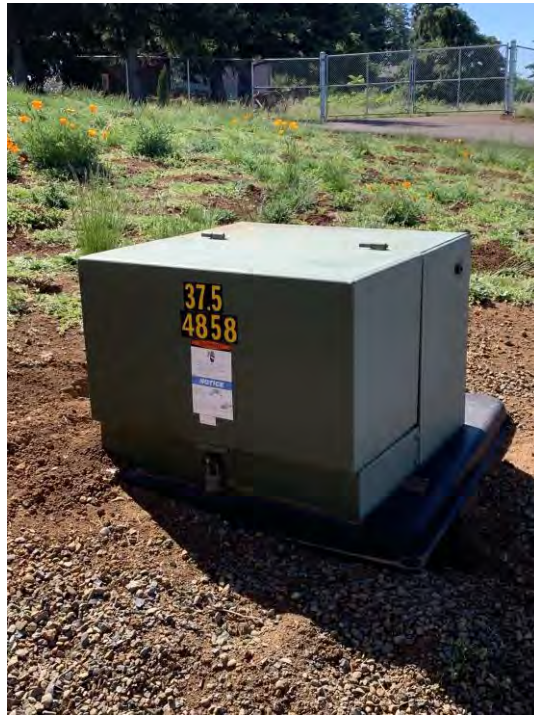
Figure 3.180 Unanchored Electrical Transformer
