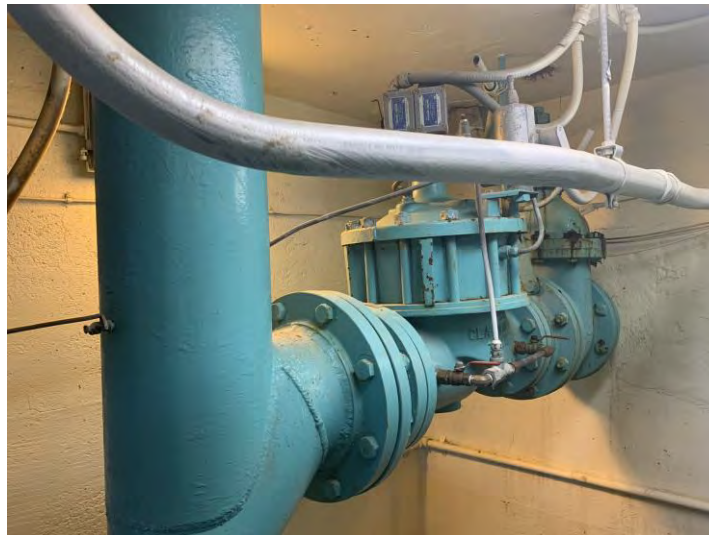
Figure 3.156 Unbraced Valve
