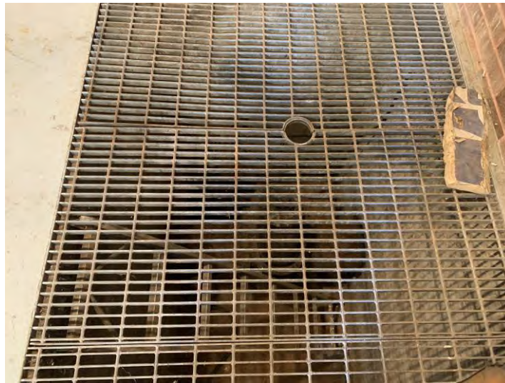
Figure 3.68 Grating without Clip Connection to Supporting Steel Framing
