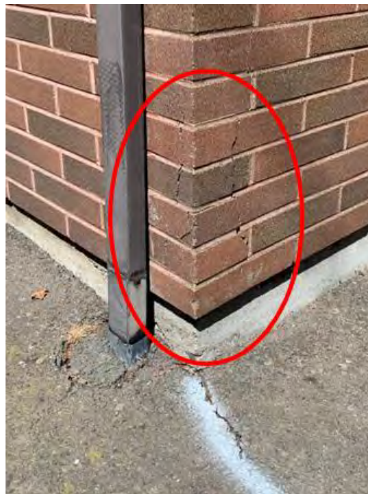
Figure 3.59 Cracking of Masonry Wall
