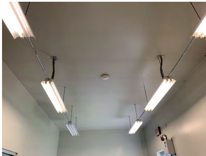
Figure 3.121 Light Fixtures without Lens Covers
