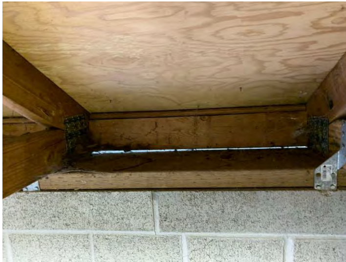
Figure 3.2 Inadequate Connection between Blocking and Masonry Wall Top Plate
