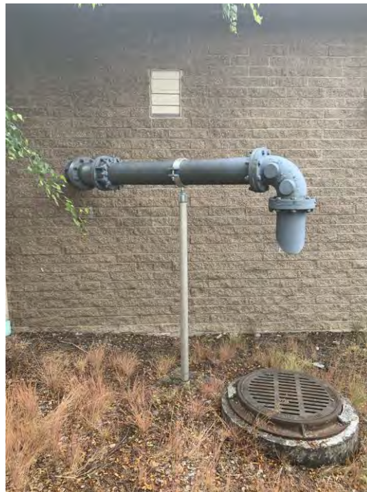
Figure 3.107 Unbraced Overflow Pipe on South Side of Pump Station
