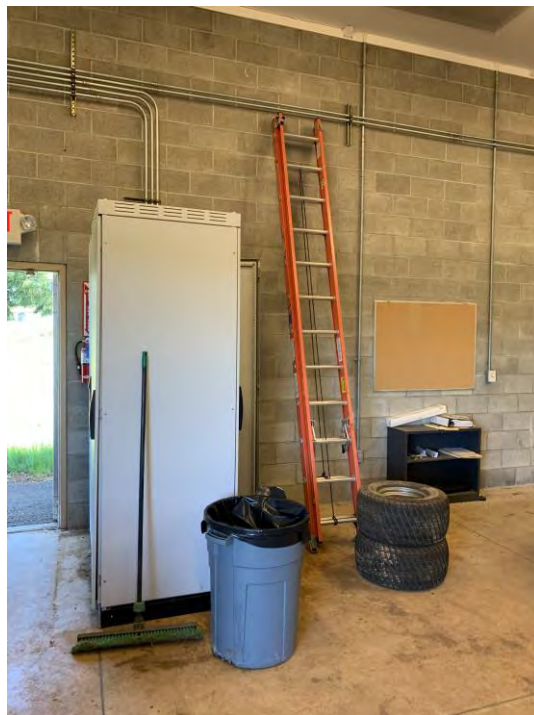
Figure 3.179 Unrestrained Ladder
