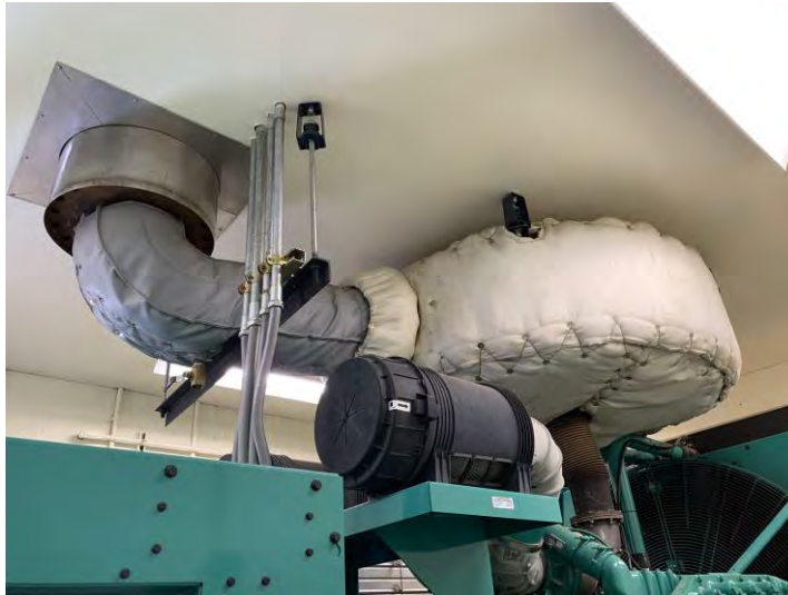
Figure 3.97 Unbraced Emergency Generator Muffler
