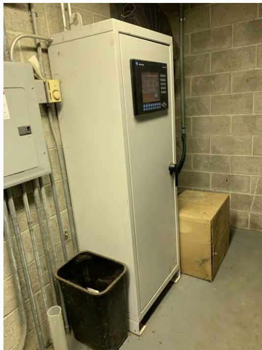
Figure 3.17 Unanchored Control Cabinet
