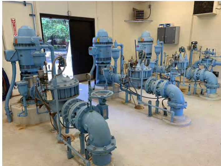
Figure 3.77 Unbraced Piping and Valves
