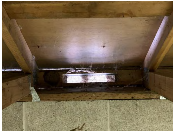
Figure 3.13 Inadequate Connection between Blocking and Masonry Wall Top Plate
