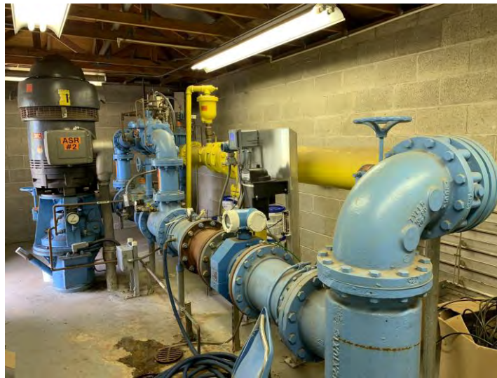
Figure 3.4 Unbraced Piping, Valves, and Air Relief Valve
