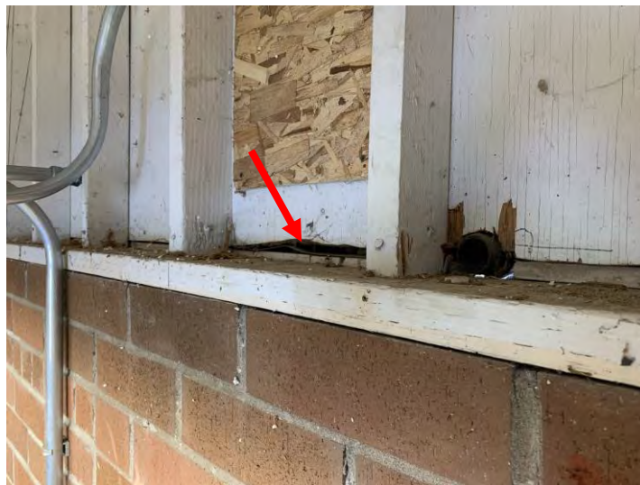
Figure 3.50 Sheathing Not Connected to Top Plate of Interior Masonry Wall
