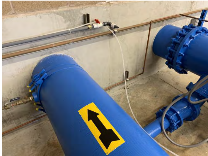
Figure 3.135 Rigid Pipe Connection Through Wall
