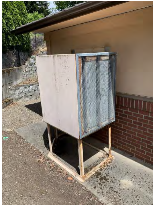
Figure 3.45 Unanchored Emergency Generator Air Intake Support Frame
