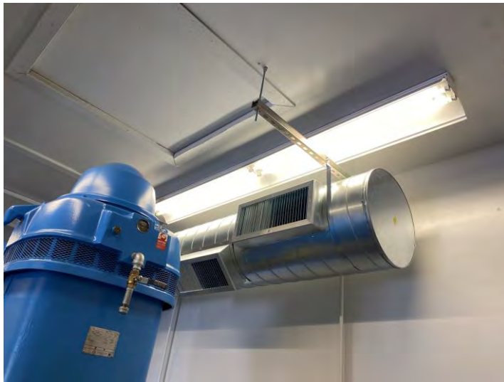
Figure 3.98 Light Fixtures without Lens Covers
