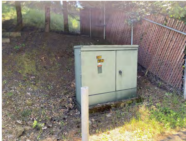
Figure 3.82 Unanchored Electrical Transformer
