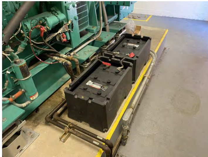
Figure 3.96 Unrestrained Emergency Generator Starter Batteries
