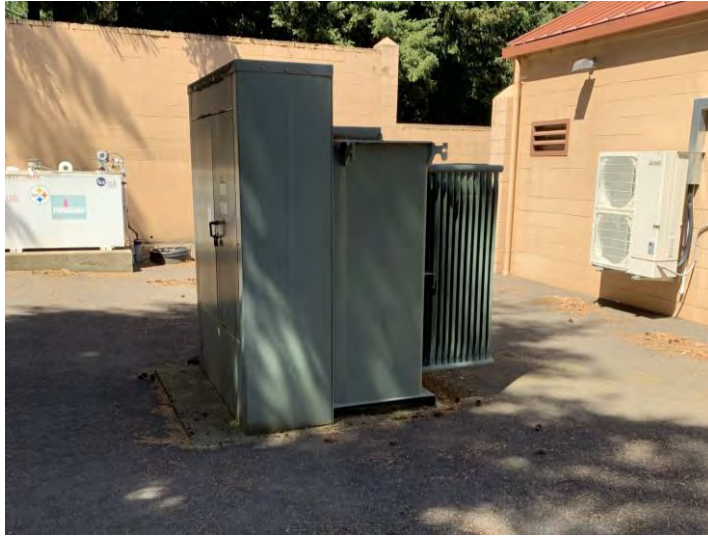
Figure 3.101 Unanchored Electrical Transformer
