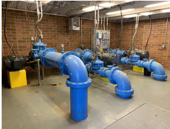
Figure 3.53 Unbraced Piping and Valves
