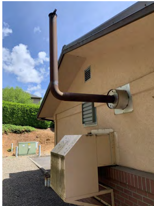
Figure 3.47 Unbraced Emergency Generator Exhaust Pipe
