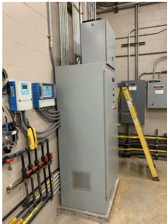
Figure 3.187 Control Cabinet with Unknown Anchorage Details
