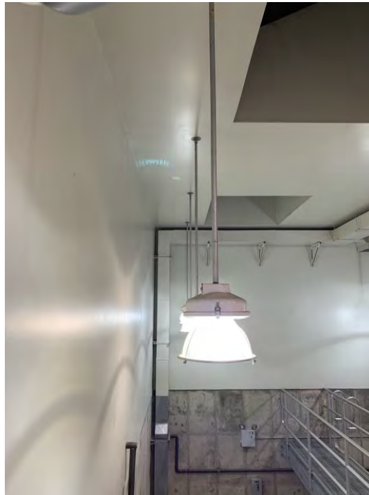
Figure 3.120 Unrestrained Pendant Light Fixtures
