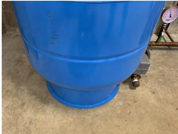
Figure 3.202 Unanchored Pressure Tank
