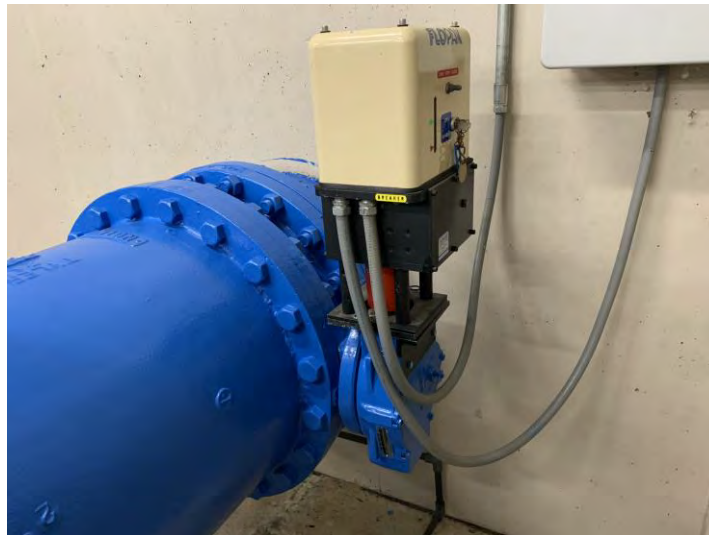
Figure 3.185 Unbraced Seismic Valve
