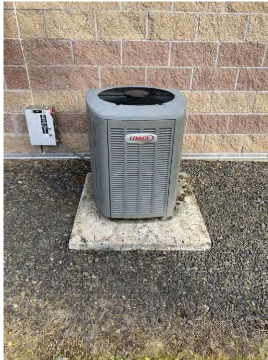
Figure 3.124 Unanchored HVAC Condenser Unit
