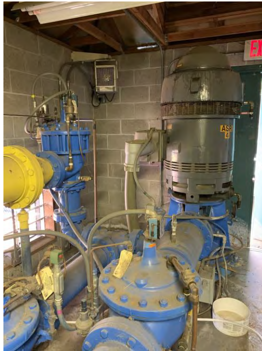
Figure 3.16 Unbraced Pump Motor
