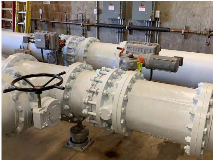
Figure 3.201 Unbraced Seismic Valves
