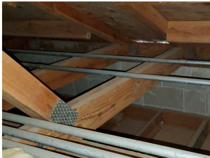
(b) As-built Framing Configuration Different than Shown on Original Design Drawings
