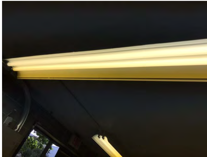
Figure 3.29 Light Fixtures without Lens Covers
