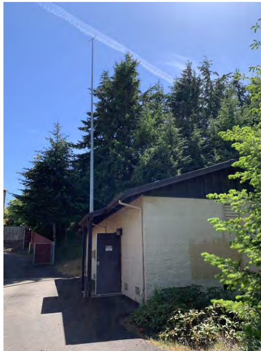
Figure 3.81 SCADA Antenna
