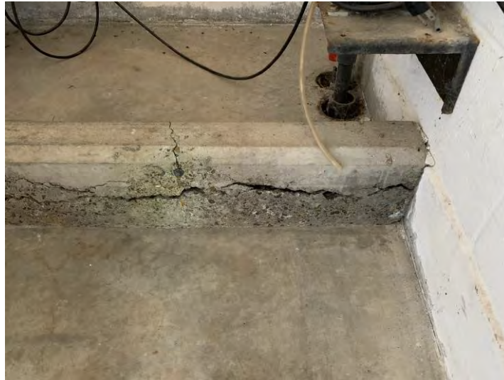
Figure 3.91 Deteriorated Concrete Curb
