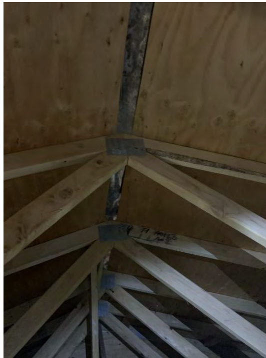
Figure 3.103 Roof Sheathing not Continuous to Ridge Line
