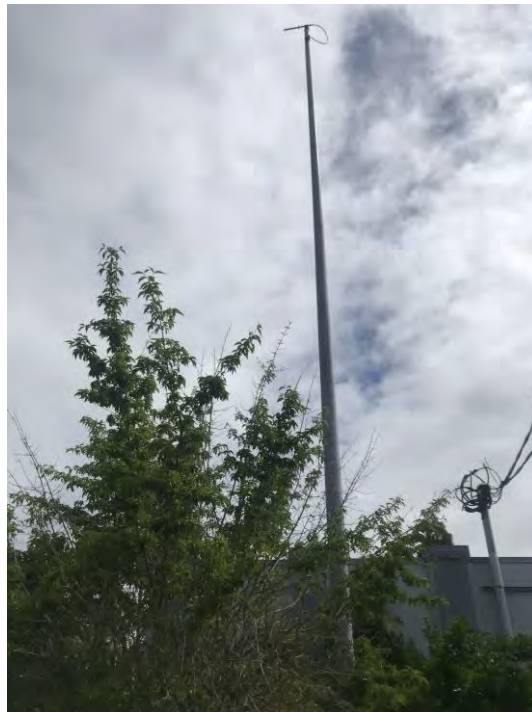
Figure 3.164 SCADA Antenna
