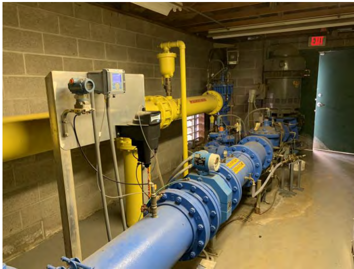
Figure 3.15 Unbraced Piping, Valves, and Air Relief Valve
