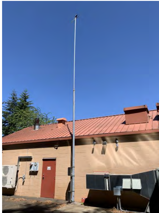
Figure 3.99 SCADA Antenna
