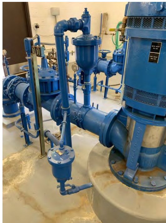
Figure 3.43 Unbraced Air Relief Valves
