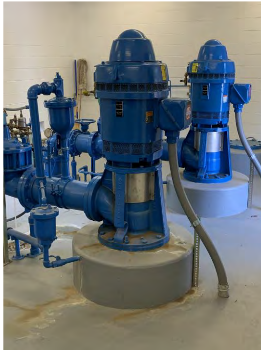
Figure 3.44 Unbraced Pump Motor
