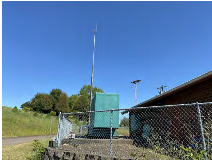
Figure 3.57 SCADA Antenna
