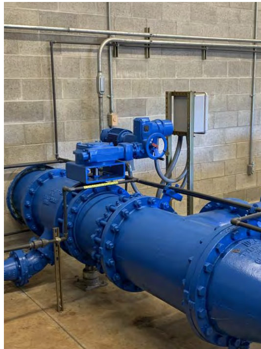
Figure 3.173 Unbraced Seismic Valve
