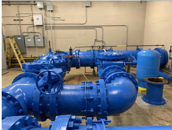
Figure 3.184 Unbraced Piping and Valves
