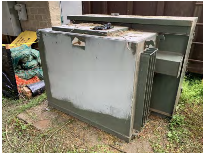
Figure 3.19 Unanchored Electrical Transformer
