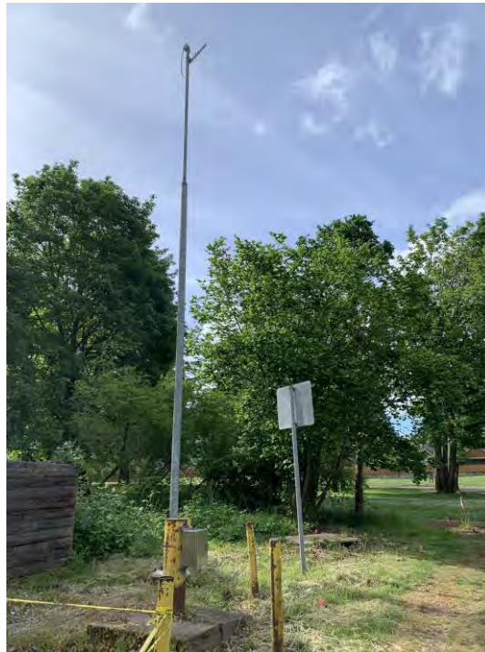
Figure 3.8 SCADA Antenna
