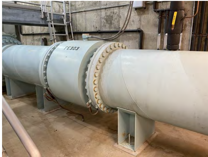
Figure 3.114 Unbraced Pipe
