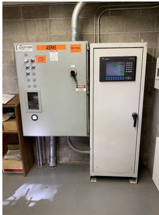
Figure 3.28 Unanchored Control Cabinet
