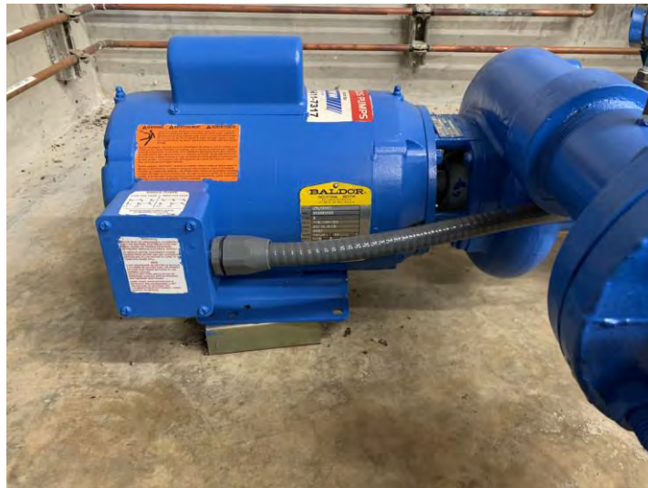
Figure 3.138 Unanchored Recirculation Pump Motor
