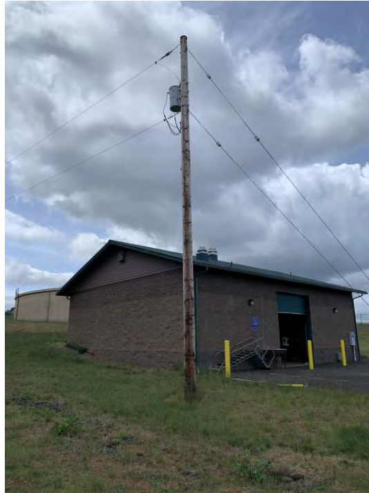
Figure 3.144 Pole-mounted Electrical Transformer
