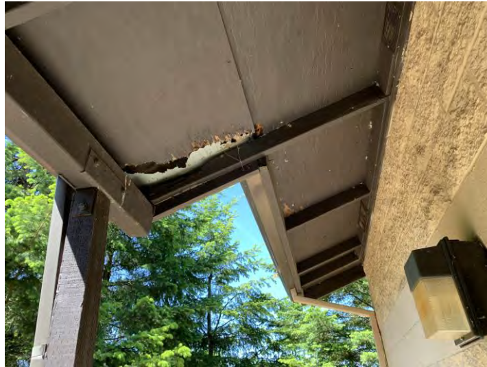
Figure 3.74 Sheathing and Framing Deterioration
