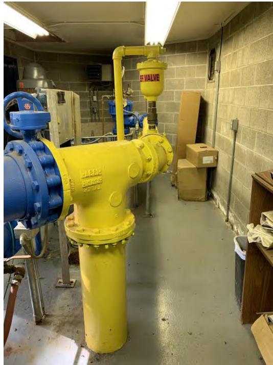
Figure 3.25 Unbraced Air Relief Valve
