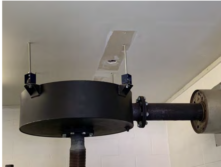
Figure 3.46 Unbraced Emergency Generator Muffler
