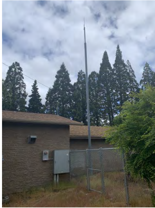
Figure 3.110 SCADA Antenna
