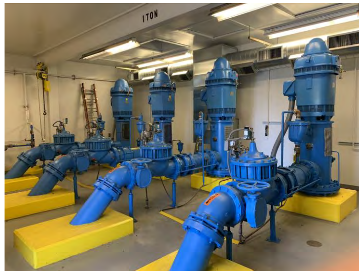
Figure 3.86 Unbraced Piping and Valves
