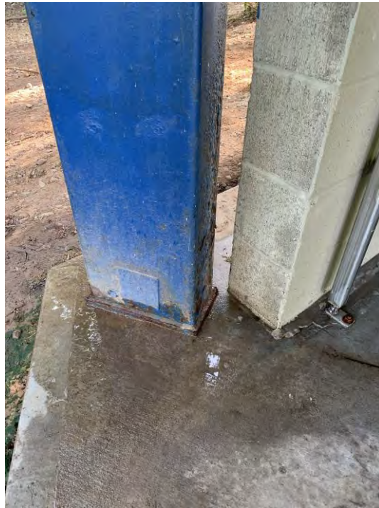
Figure 3.23 Corrosion Damage at Northern-Most Pavilion Steel Column
