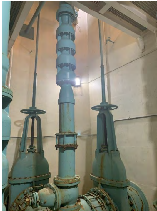
Figure 3.157 Unbraced Pump Bells and Valve Operator Riser Shafts
