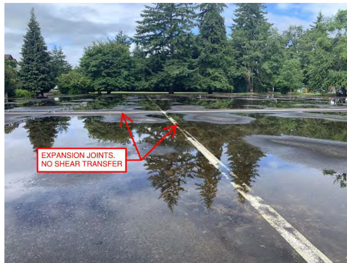
Figure 3.150 Fairmount Reservoir Roof Expansion Joints
