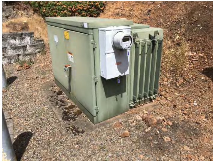
Figure 3.48 Unanchored Electrical Transformer
