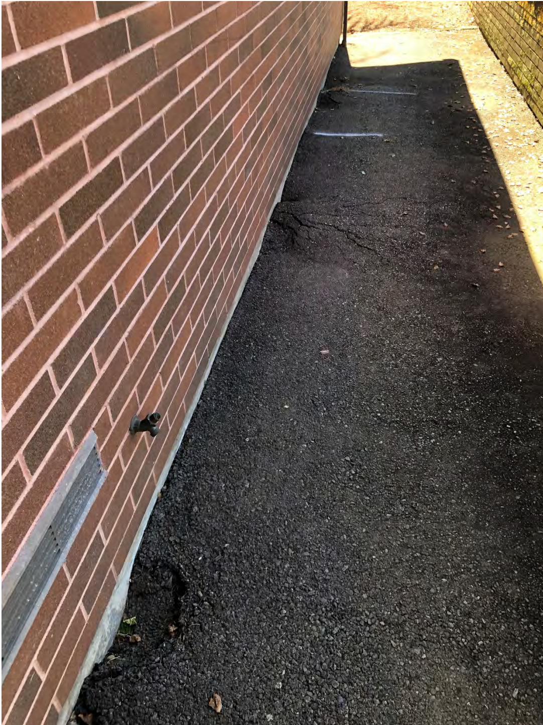
Exhibit 3-12: Photo of Cracking and Settlement along Edwards Pump Station West Wall During Site Visit
