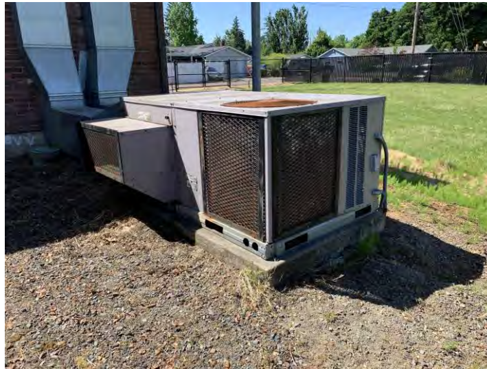
Figure 3.67 Unanchored HVAC Condenser Unit
