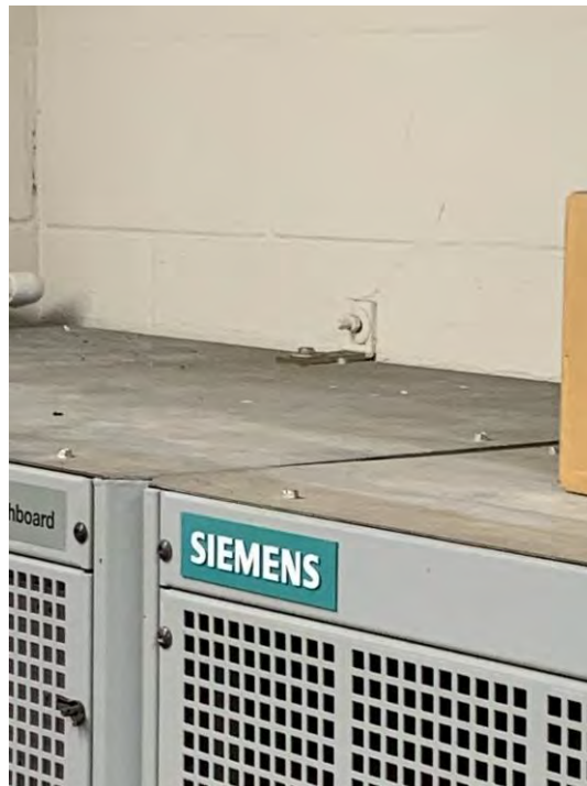
Figure 3.94 Electrical Cabinet with Single Anchor Bracket at Top of Cabinet
