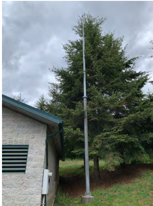
Figure 3.188 SCADA Antenna
