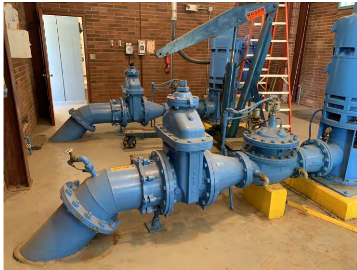
Figure 3.61 Unbraced Piping and Valves
