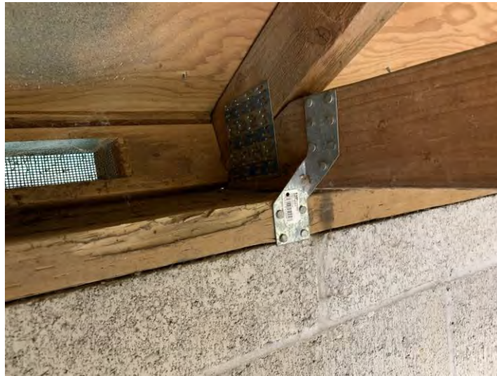
Figure 3.3 Roof Truss to Masonry Wall Top Plate Connection
