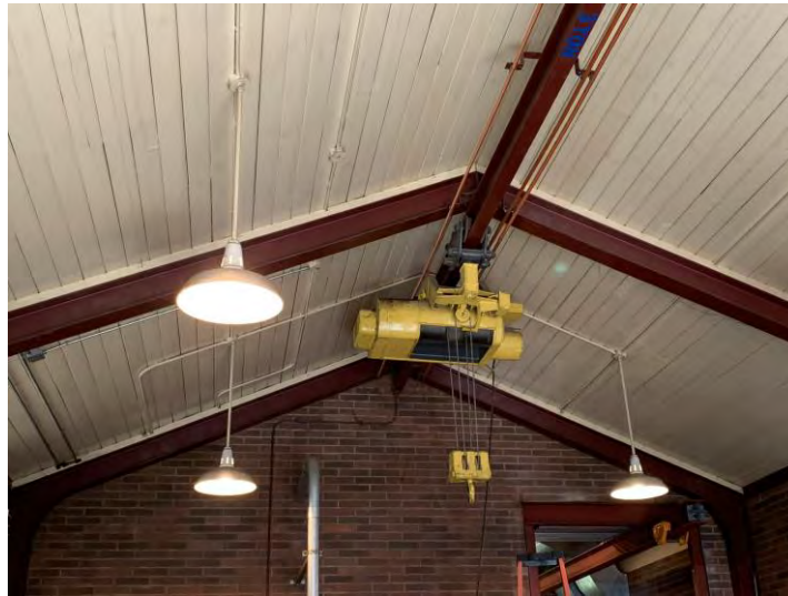
Figure 3.65 Pendant Lights without Lens Covers
