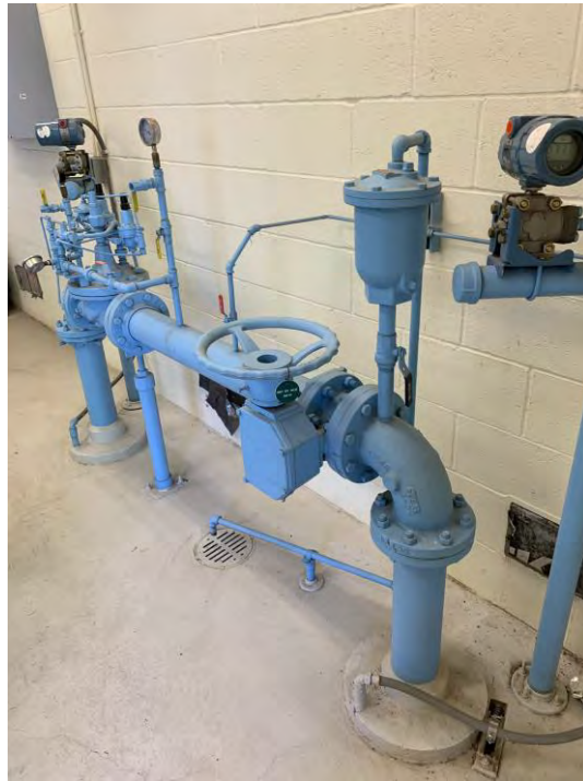
Figure 3.78 Unbraced Air Relief Valve
