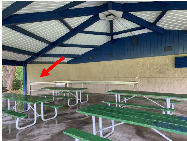
Figure 3.22 Free-Standing Masonry Wall without Bracing
