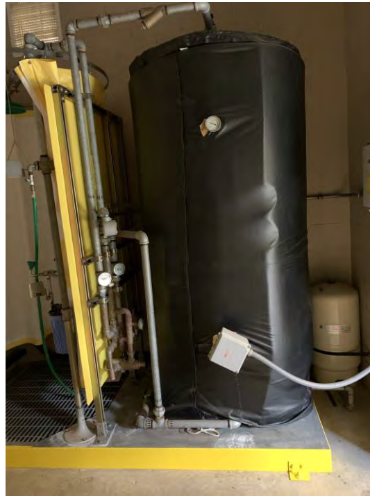
Figure 3.190 Inadequate Overturning Anchorage of Water Heater
