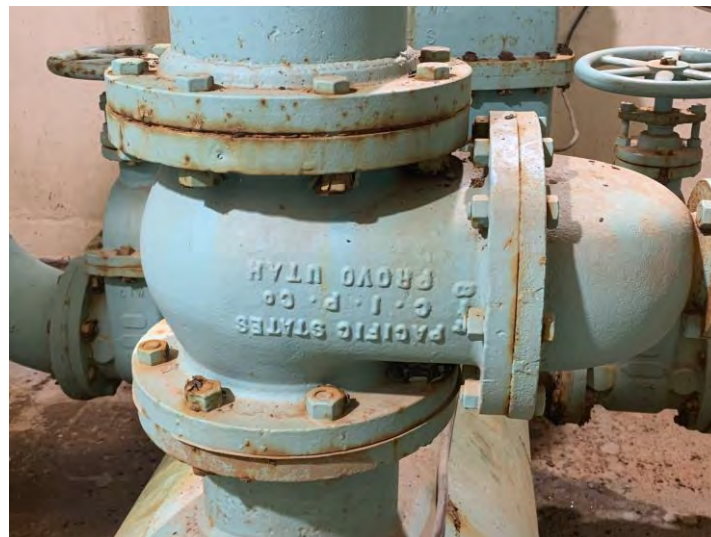
Figure 3.158 Cast Iron Valve
