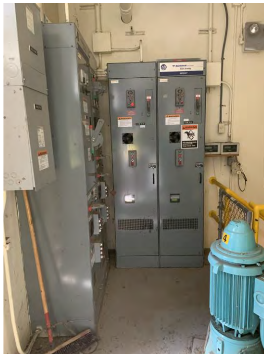
Figure 3.162 Electrical Cabinets with Unknown Anchorage Details
