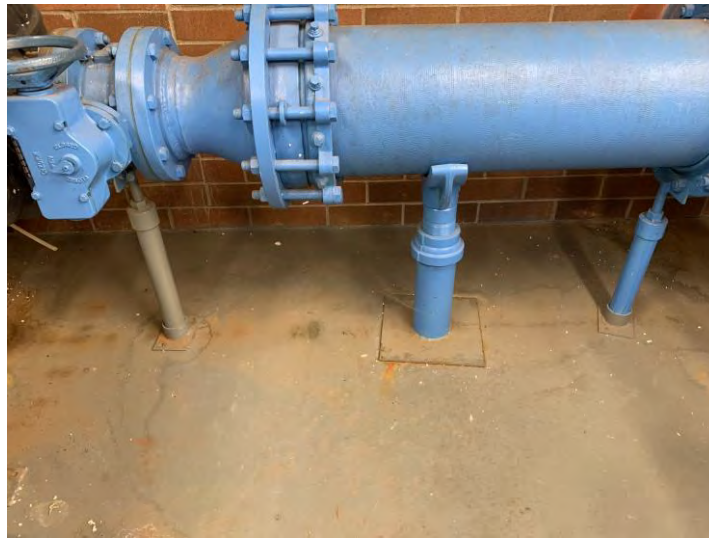
Figure 3.54 Pipe Support Stanchion Missing Anchors into Floor Slab
