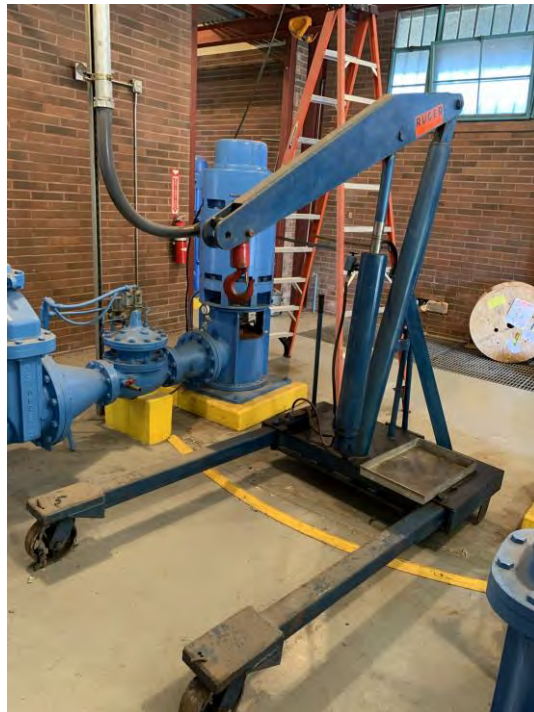
Figure 3.70 Unrestrained Ladder and Rolling Lift
