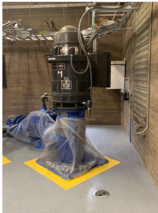
Figure 3.34 Unbraced Pump Motor
