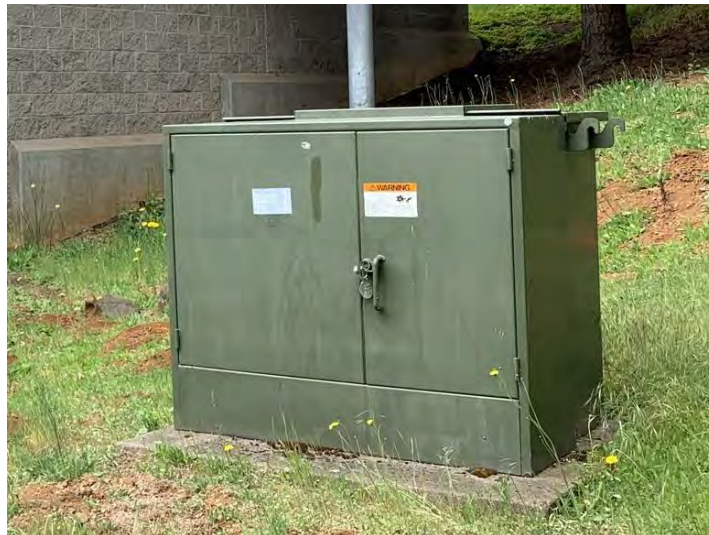
Figure 3.193 Unanchored Electrical Transformer
