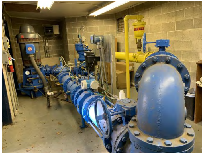
Figure 3.24 Unbraced Piping, Valves, and Air Relief Valve
