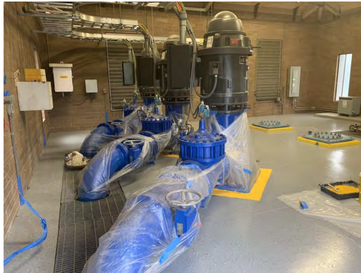
Figure 3.33 Unbraced Piping and Valves
