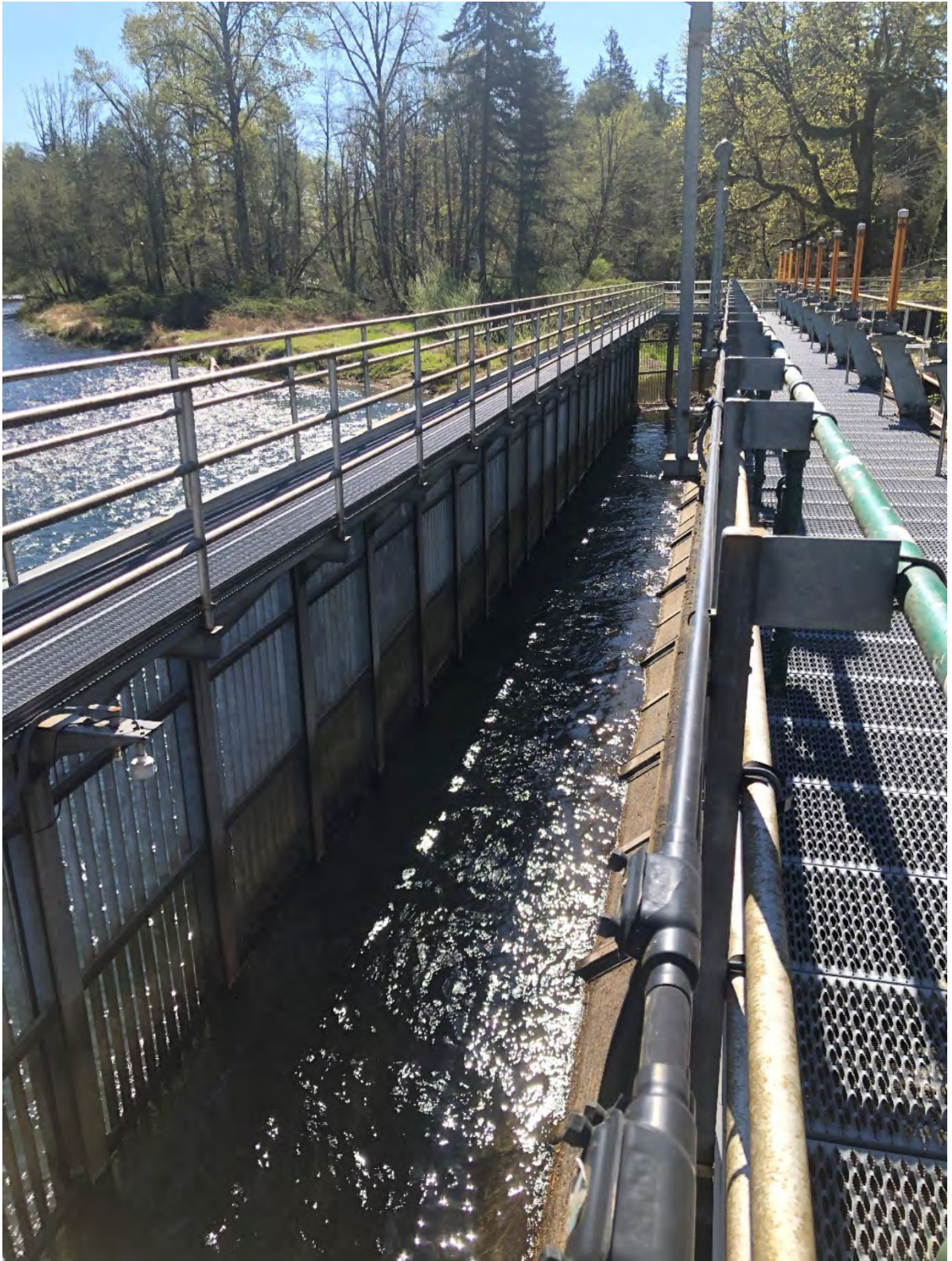
Exhibit 3-23: Photo Showing Middle Intake at Geren Island Water Treatment Plant
