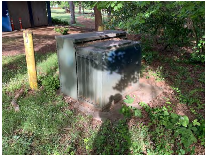
Figure 3.30 Unanchored Electrical Transformer
