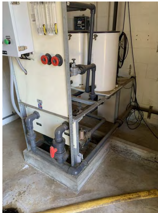
Figure 3.90 Chlorine System without Adequate Anchorage
