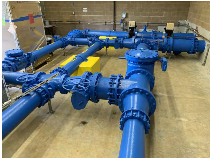
Figure 3.136 Unbraced Piping and Valves
