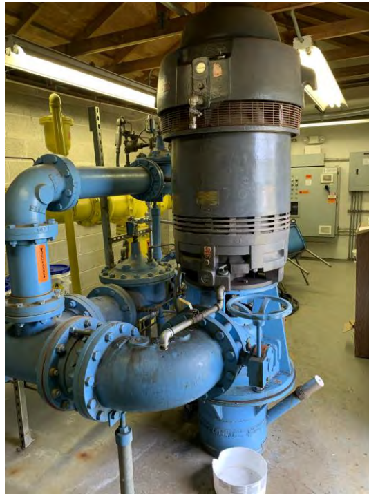
Figure 3.5 Unbraced Pump Motor
