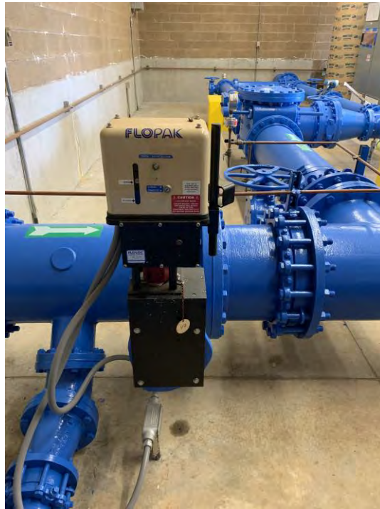
Figure 3.137 Unbraced Seismic Valve
