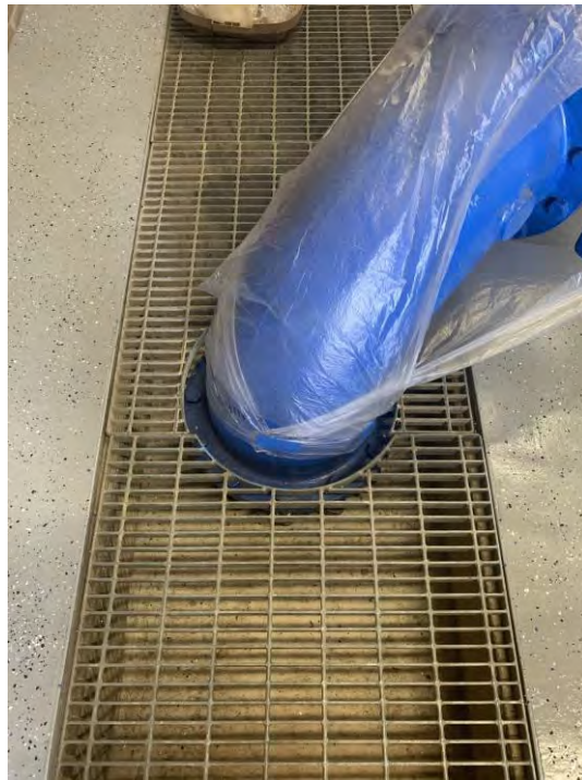
Figure 3.38 Grating without Clip Connection to Supporting Steel Framing
