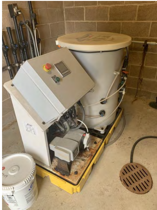
Figure 3.108 Unanchored Chlorination Skid
