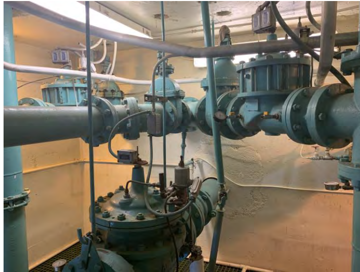
Figure 3.155 Unbraced Piping and Valves
