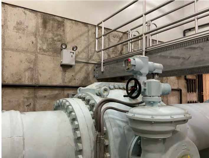
Figure 3.116 Unbraced Valve Actuator
