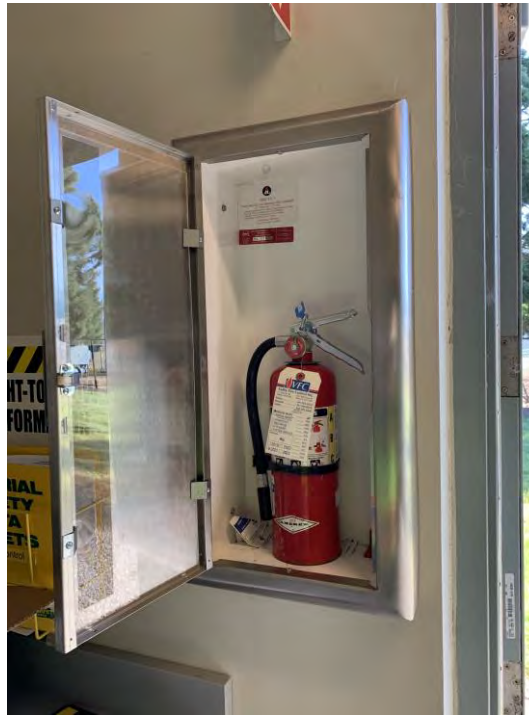
Figure 3.126 Unrestrained Fire Extinguisher
