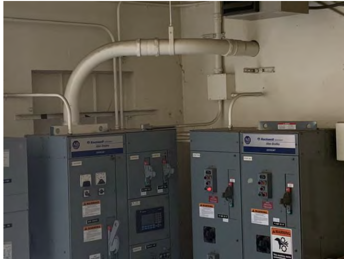
Figure 3.163 Conduits Connecting to Electrical Cabinets without Flexible Connections
