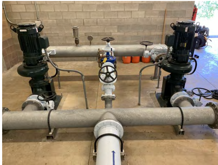
Figure 3.203 Unanchored Pump Motor
