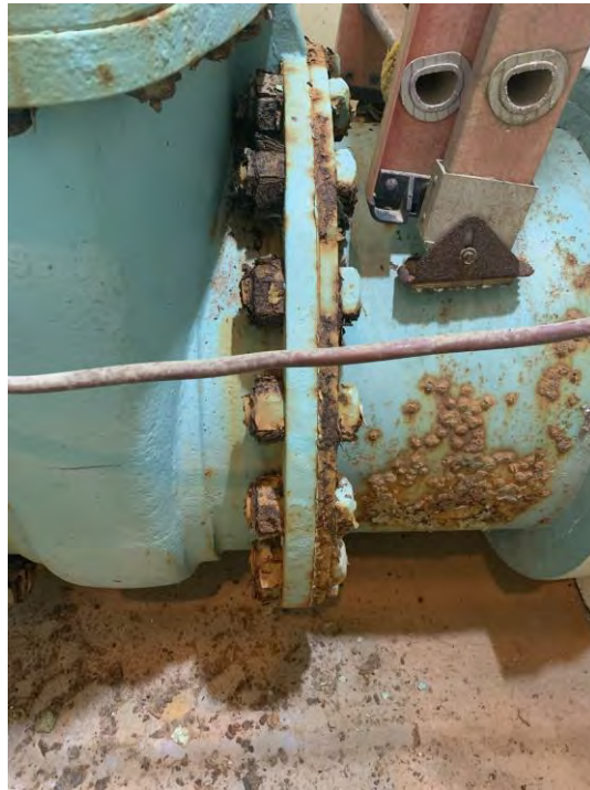
Figure 3.159 Corroded Bolts and Pipe
