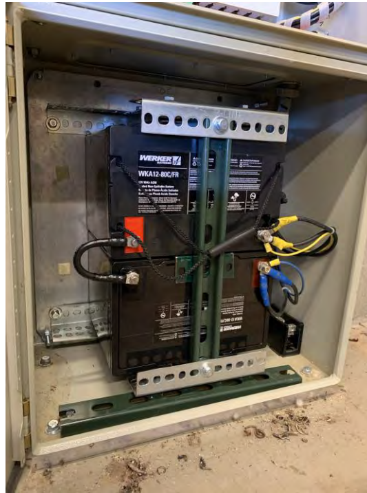
Figure 3.176 Backup Batteries without Adequate Restraint
