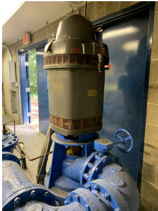
Figure 3.26 Unbraced Pump Motor
