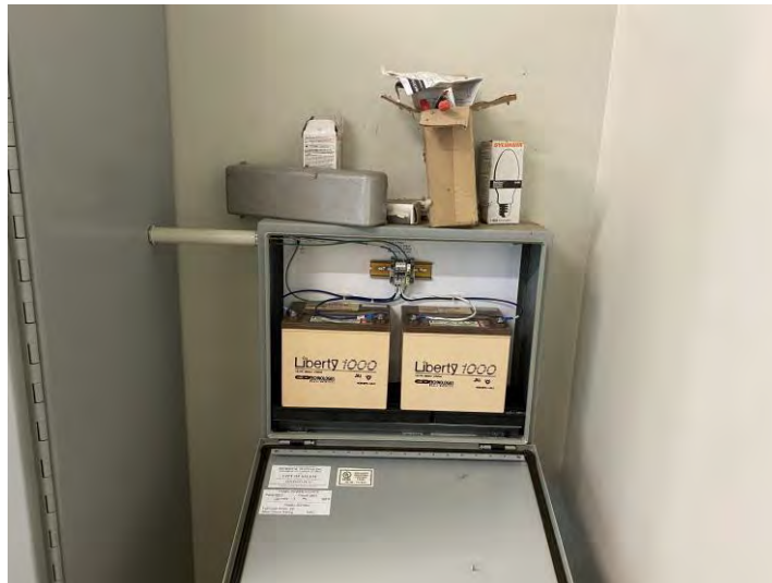
Figure 3.119 Unrestrained Backup Batteries in Battery Cabinet
