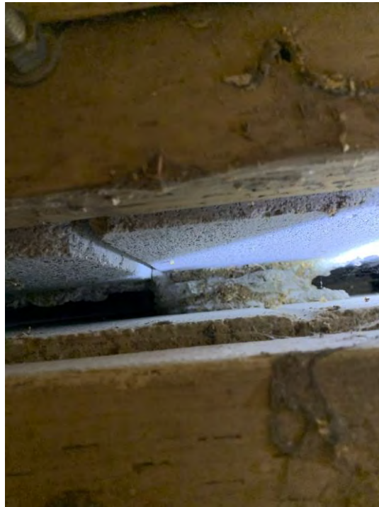
Figure 3.9 Unknown Masonry Veneer Ties to Backup Masonry Wall
