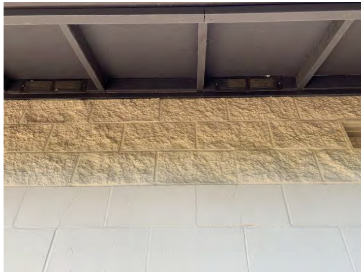
Figure 3.75 Sloped Blocking Between Wood Trusses
