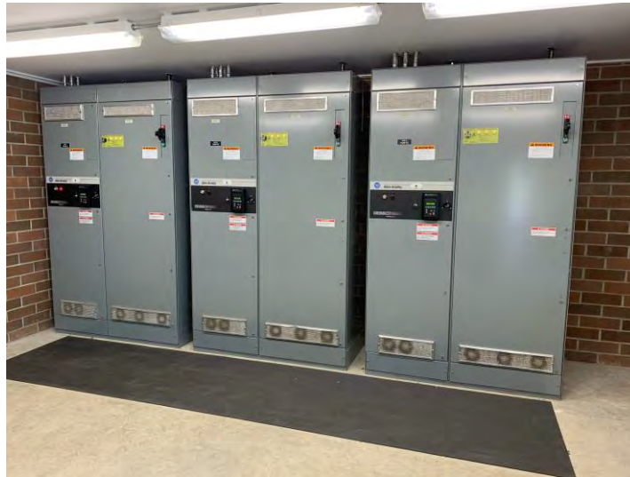
Figure 3.55 Electrical Cabinet with Unknown Anchorage Details
