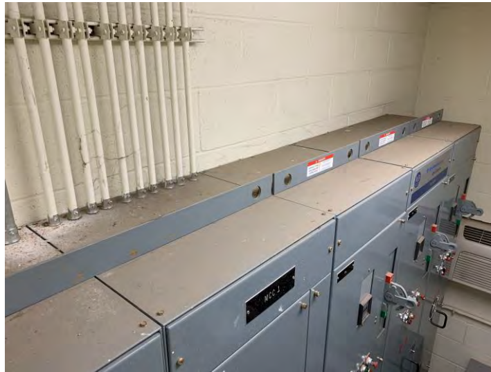
Figure 3.80 Electrical Cabinets with Unknown Anchorage Details
