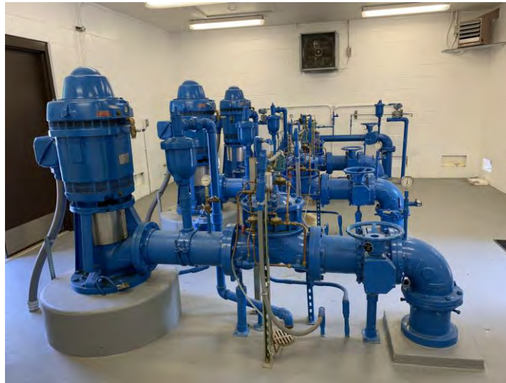
Figure 3.42 Unbraced Piping and Valves
