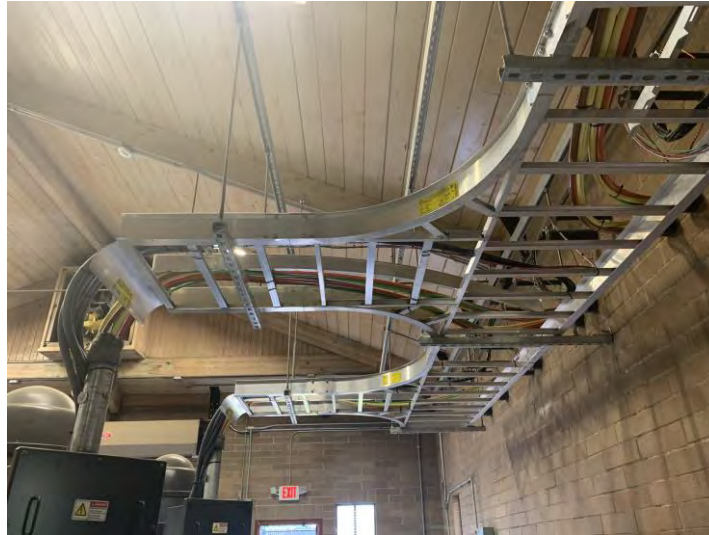
Figure 3.35 Cable Tray Lacks Longitudinal Bracing
