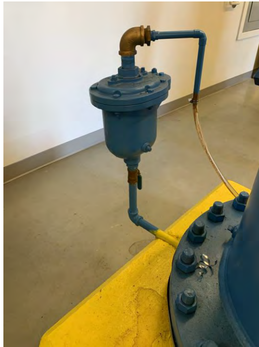
Figure 3.87 Unbraced Air Relief Valve
