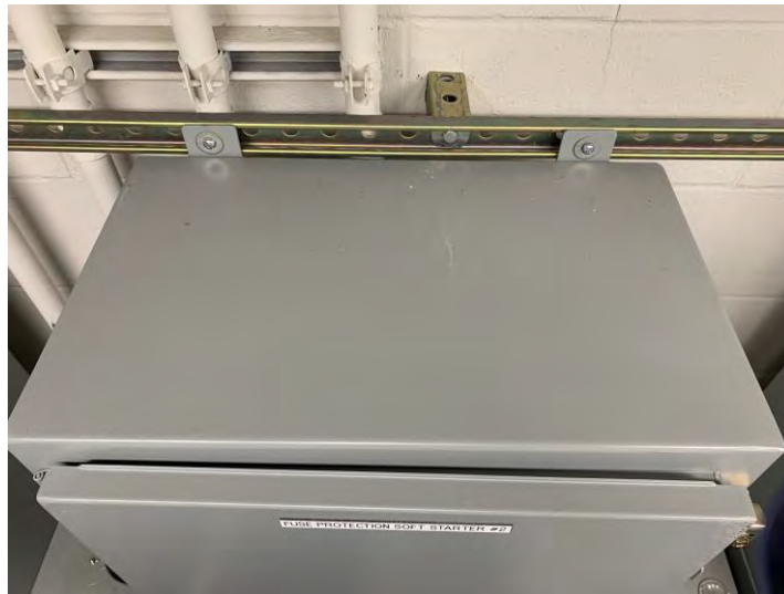
Figure 3.92 Inadequate Lag Screw and Spacer Strut Connection to Wall
