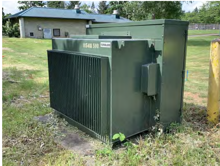
Figure 3.11 Unanchored Electrical Transformer
