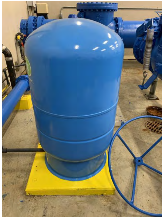
Figure 3.186 Unanchored Pressure Tank
