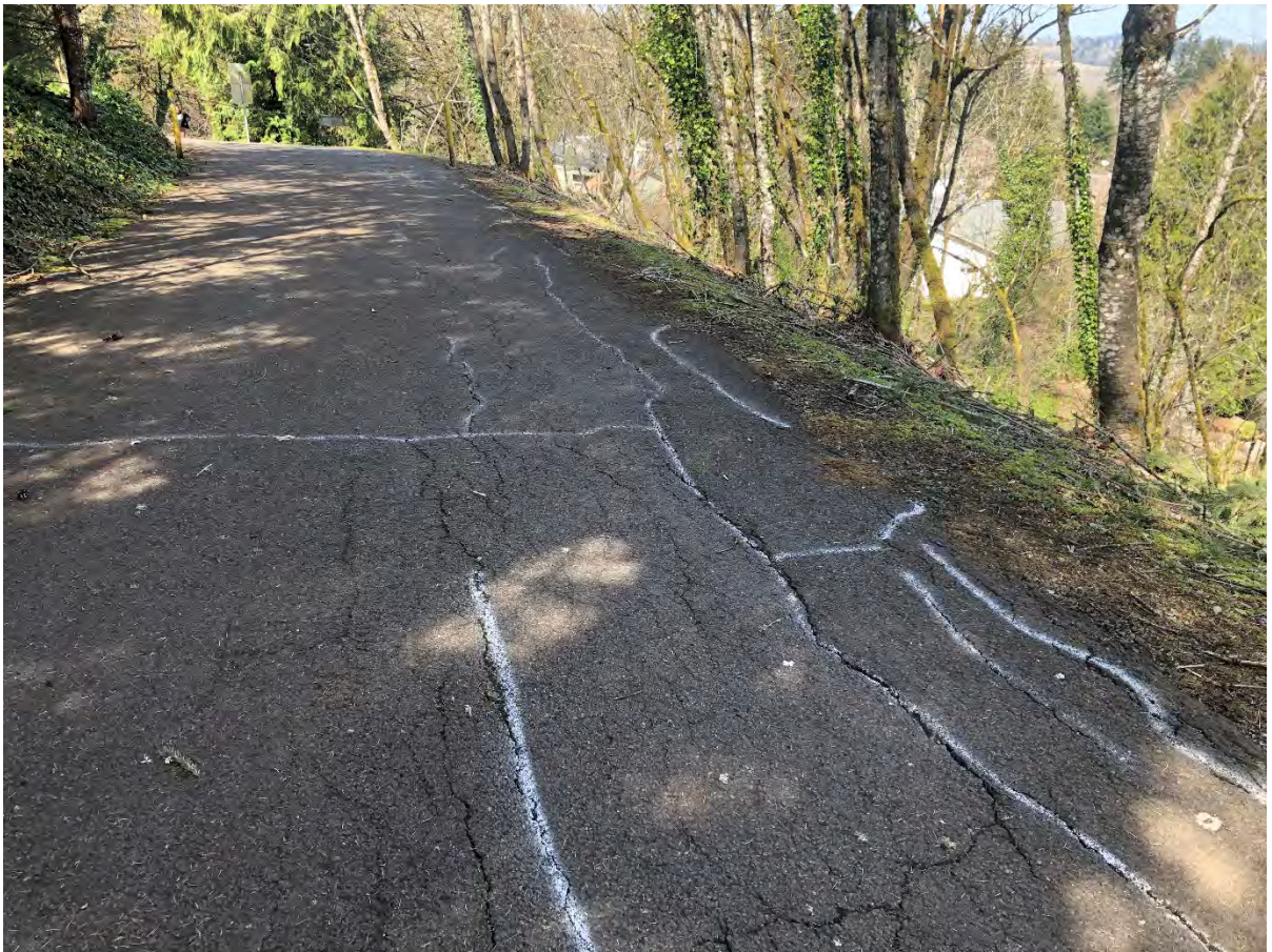
Exhibit 3-10: Photo of Cracking Observed in Driveway During Site Visit
