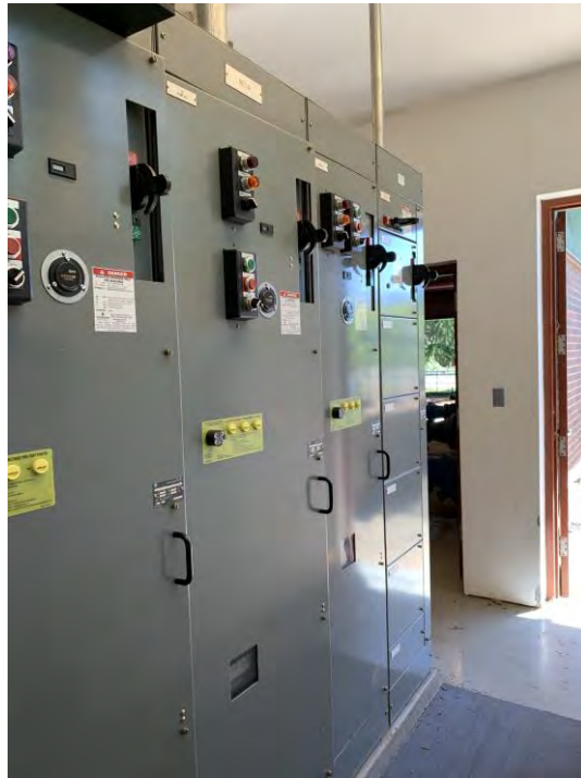
Figure 3.63 Electrical Cabinets with Unknown Anchorage Details
