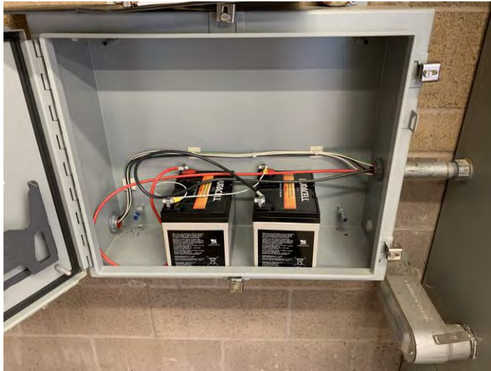
Figure 3.140 Unrestrained Backup Batteries
