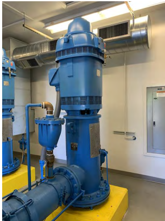
Figure 3.88 Unbraced Pump Motor
