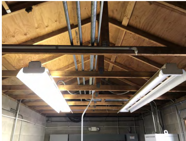
Figure 3.6 Light Fixtures without Lens Covers
