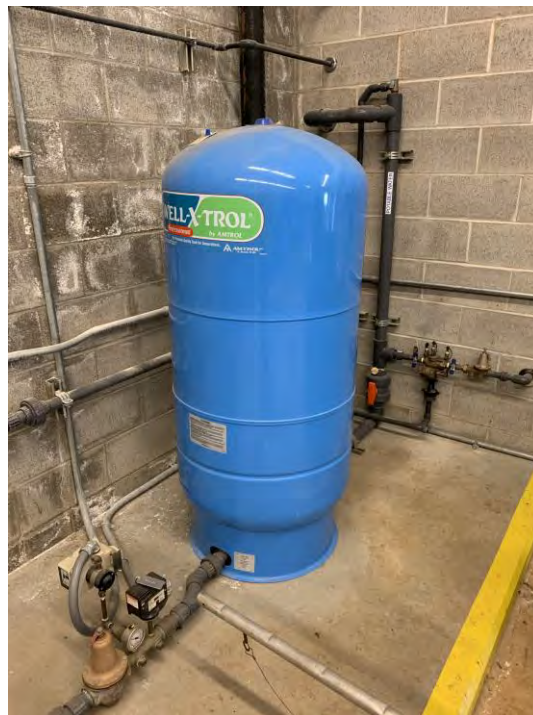
Figure 3.175 Unanchored Irrigation Pressure Tank
