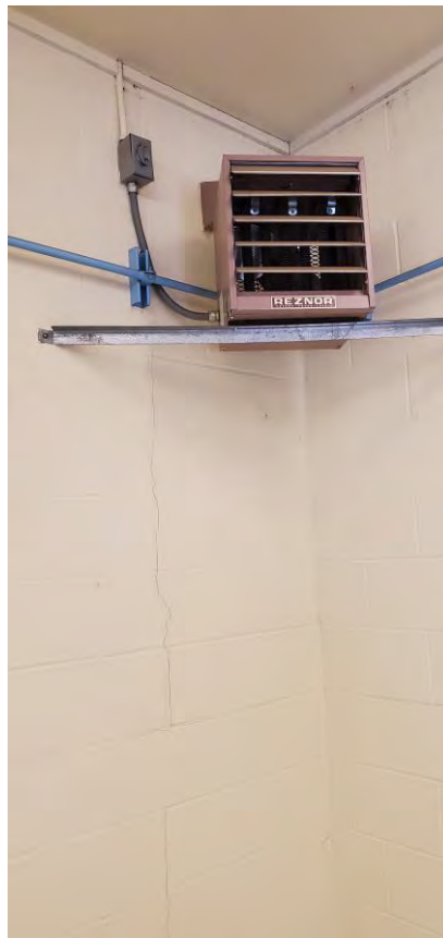
Figure 3.73 Masonry Wall Cracking
