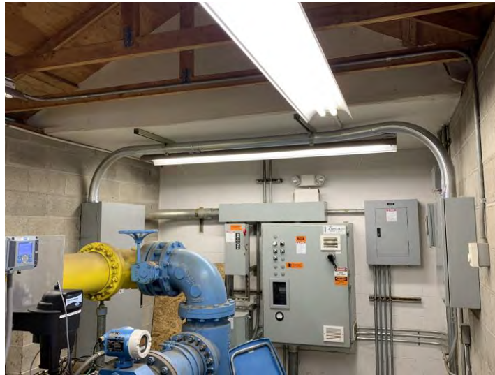
Figure 3.7 Conduit Top Connection to Electrical Panels without Flexible Connection
