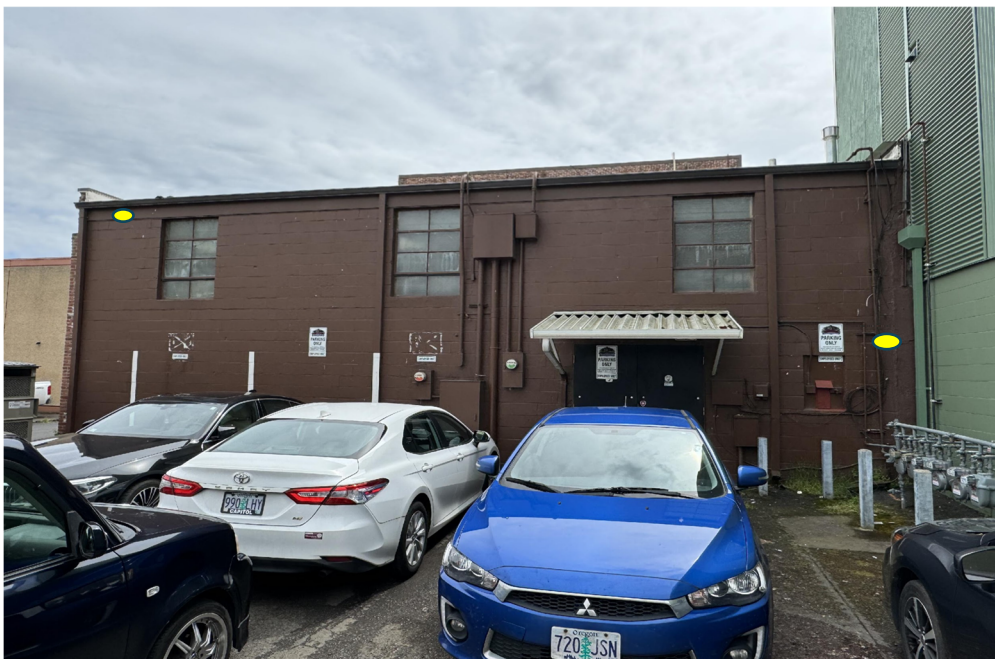
Rear exterior of building. Yellow marks represent locations for cameras.
