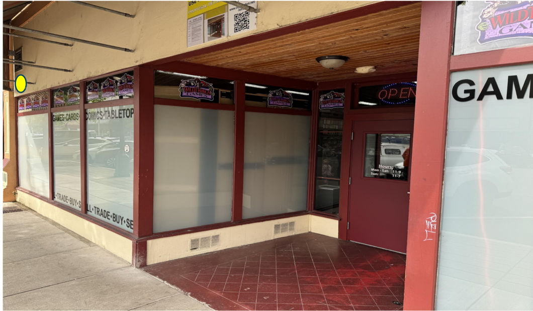
Front exterior of building. The yellow circle indicates the intended camera location.
