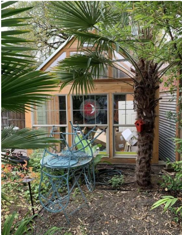
West façade - addition
