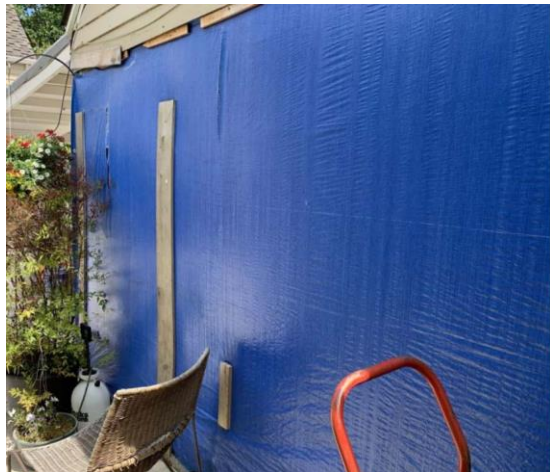
Tarps covering west end
