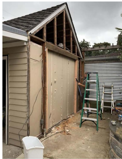
Reinforced framing – western end of garage
