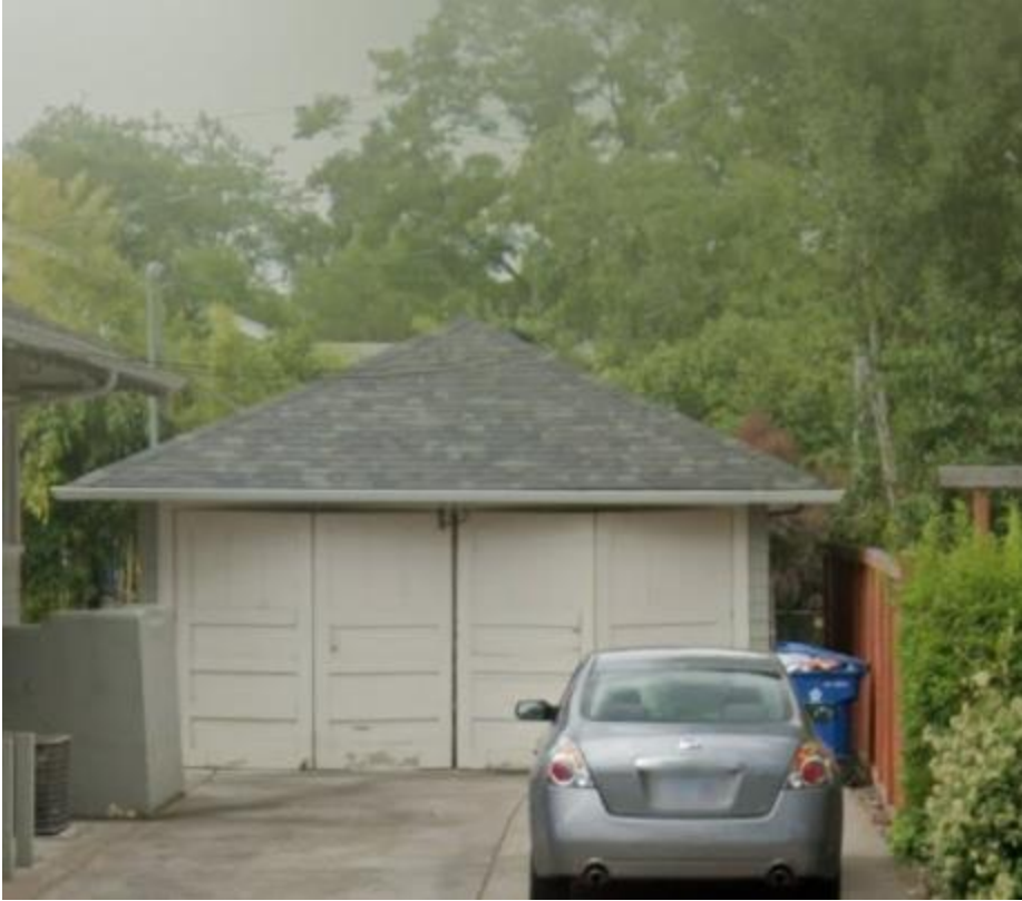
Garage – prior to Fire (Google Maps-Streetview – 2020)
