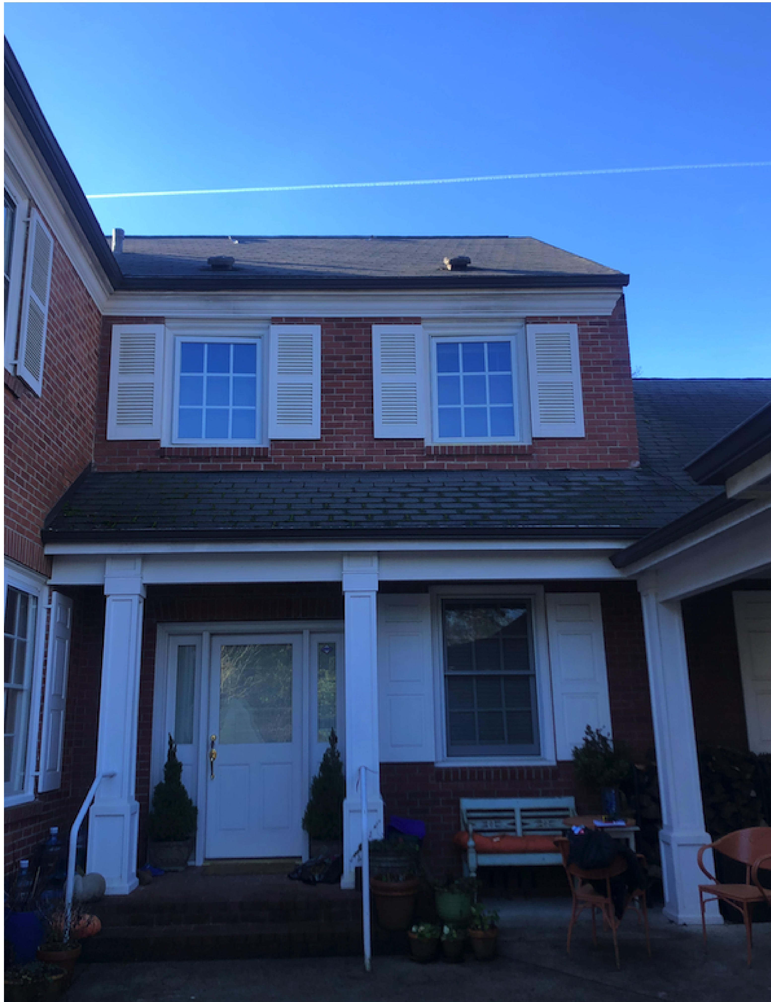
1 Existing View of East Facade A104 SCALE: 1:0.51
