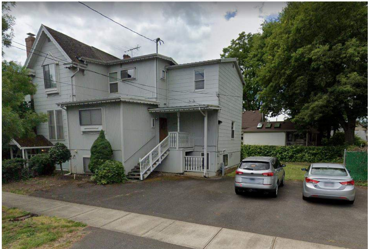
Eastern Staircase (fronting 14 th Street NE).
