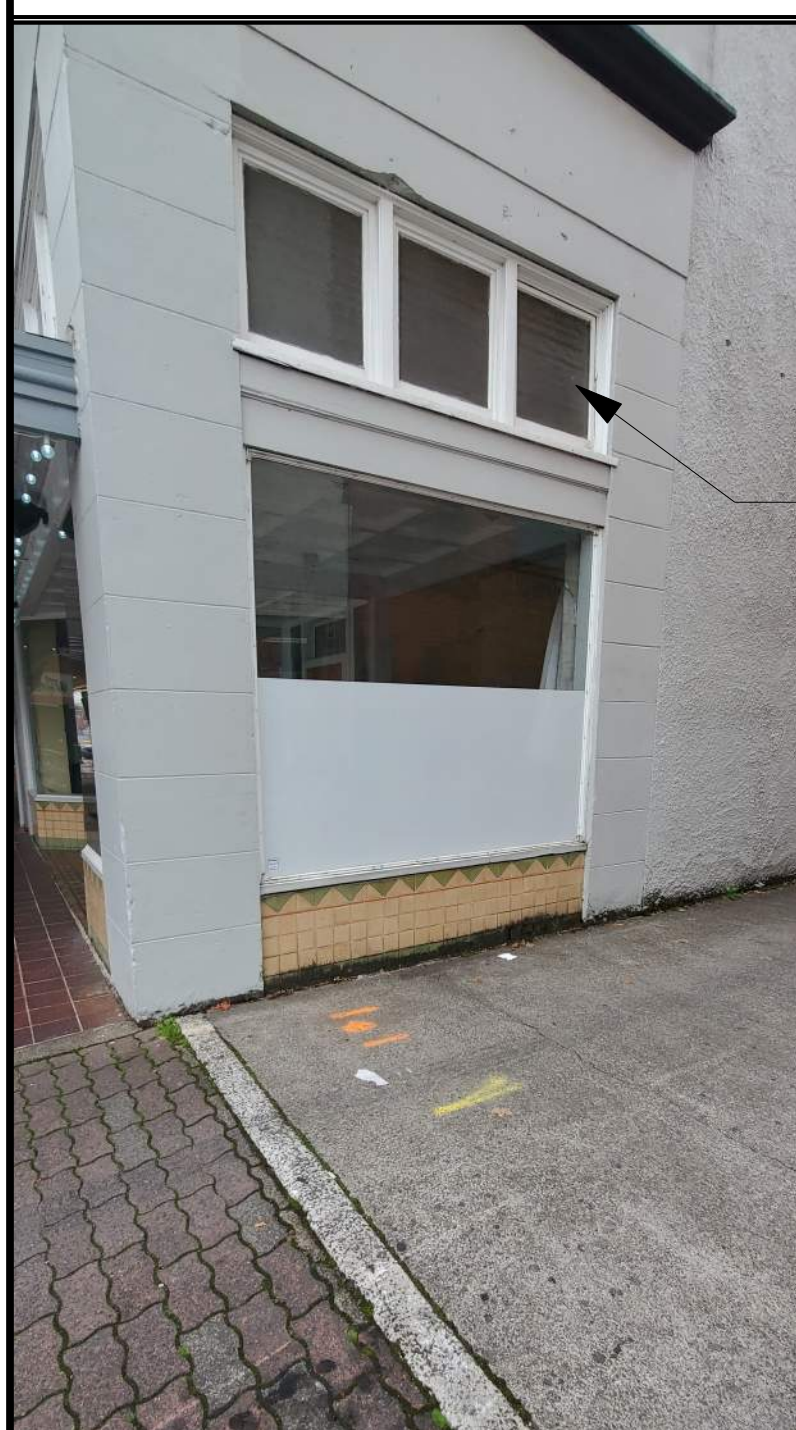
PHOTO A EXTERIOR AT ALLEY
