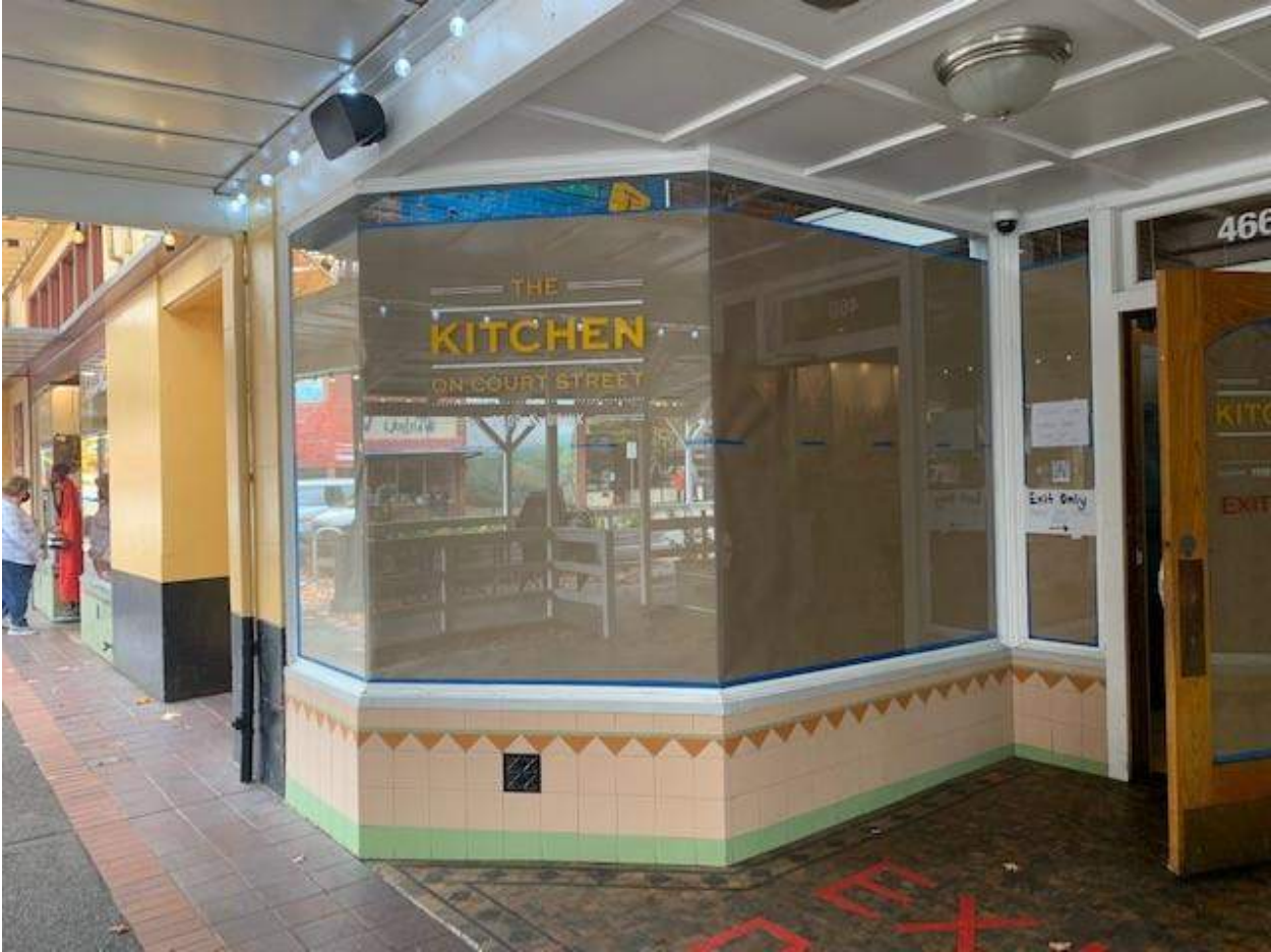
Storefront; East Side of entry
