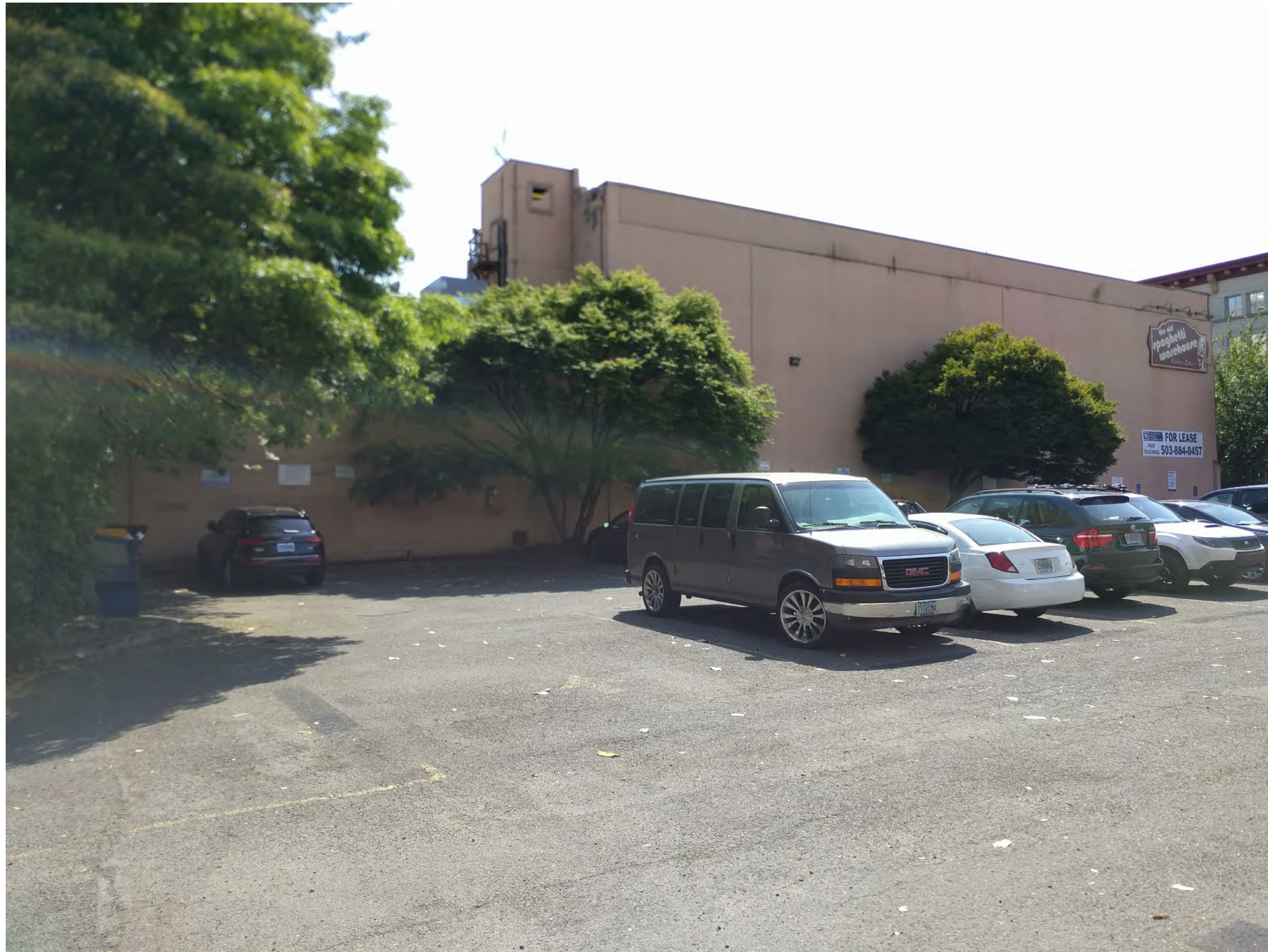
NORTH BUILDING ELEVATION - VIEW FROM ADJACENT PARKING AREA
