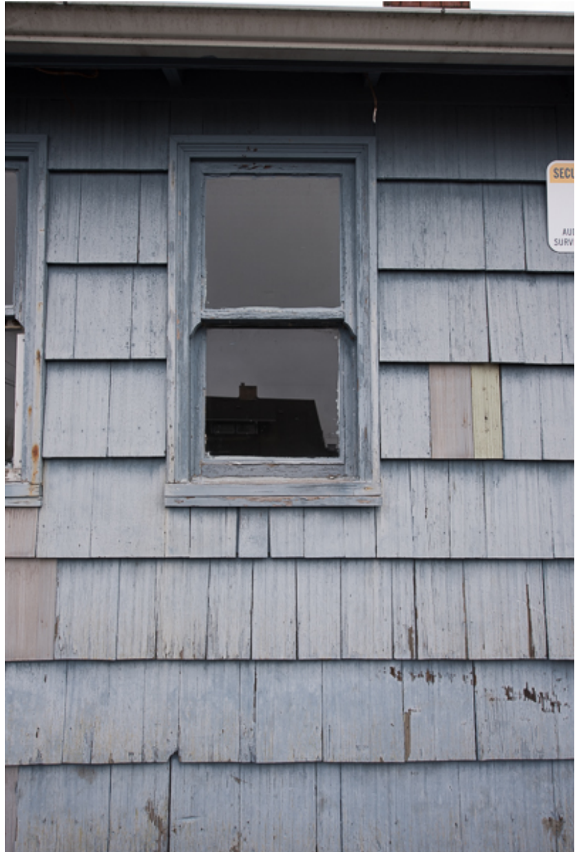
Figure 2: East Kitchen Window 4/3/2020
