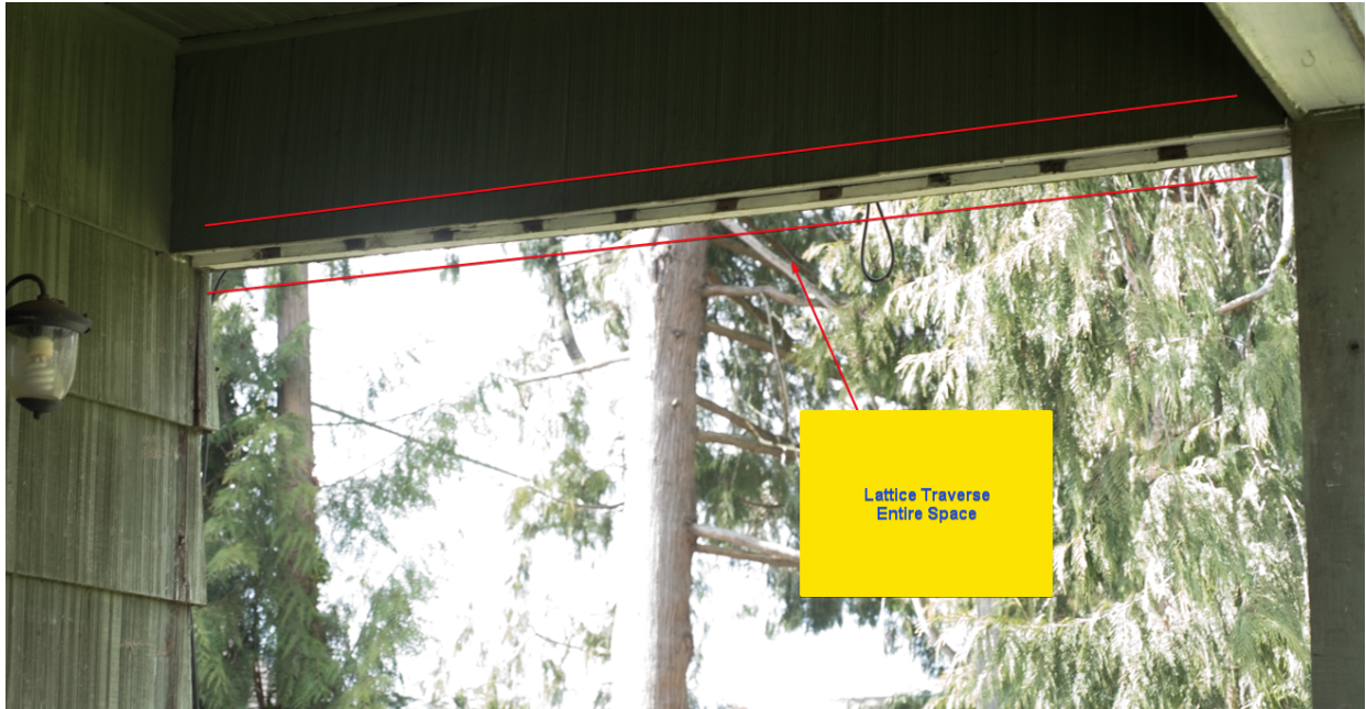
Figure 11: Front Porch West Opening - Lattice Traverses Entire Opening
