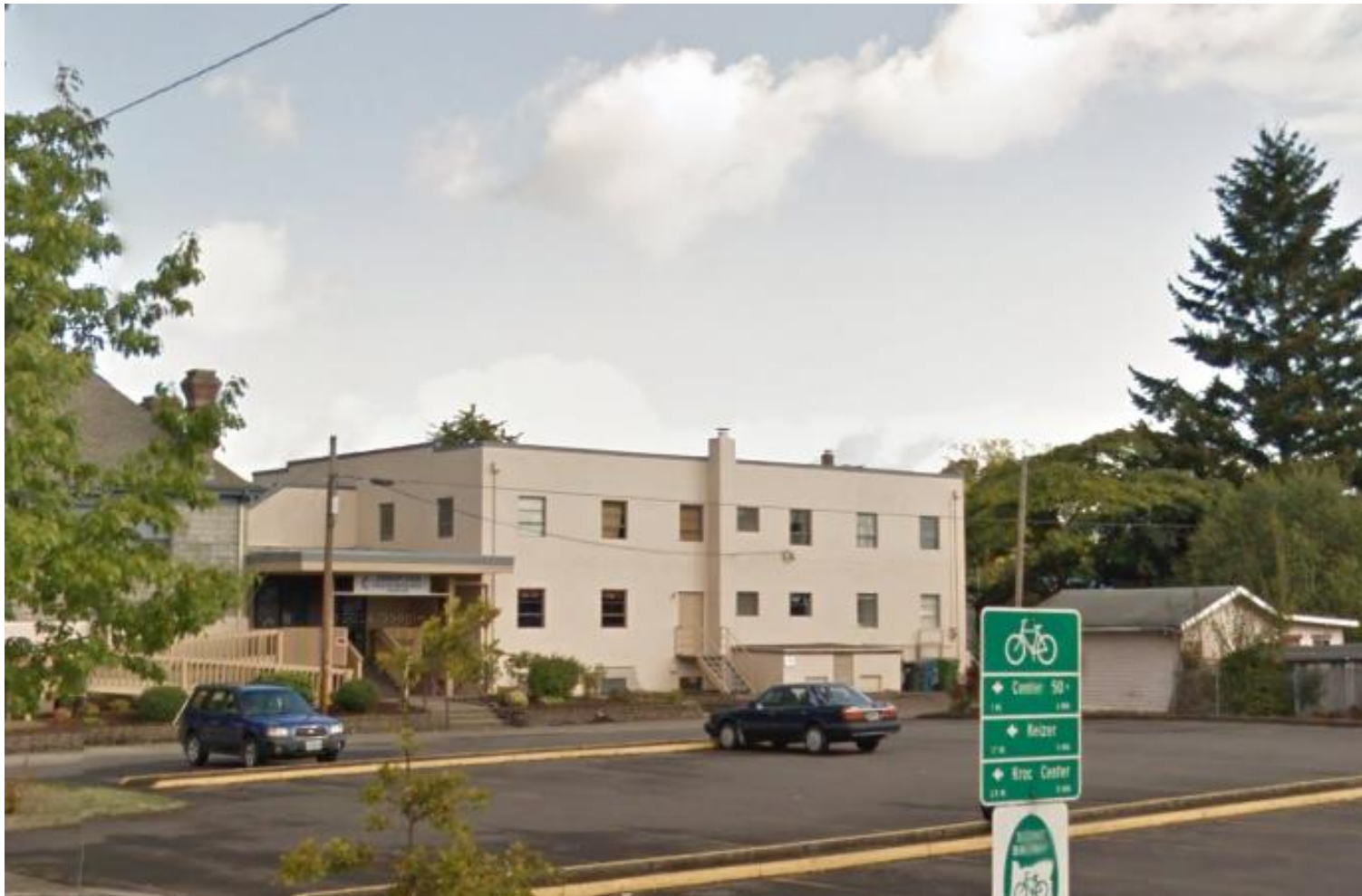
View of Education Building, south façade (looking northeast) – 820 Jefferson St. NE
