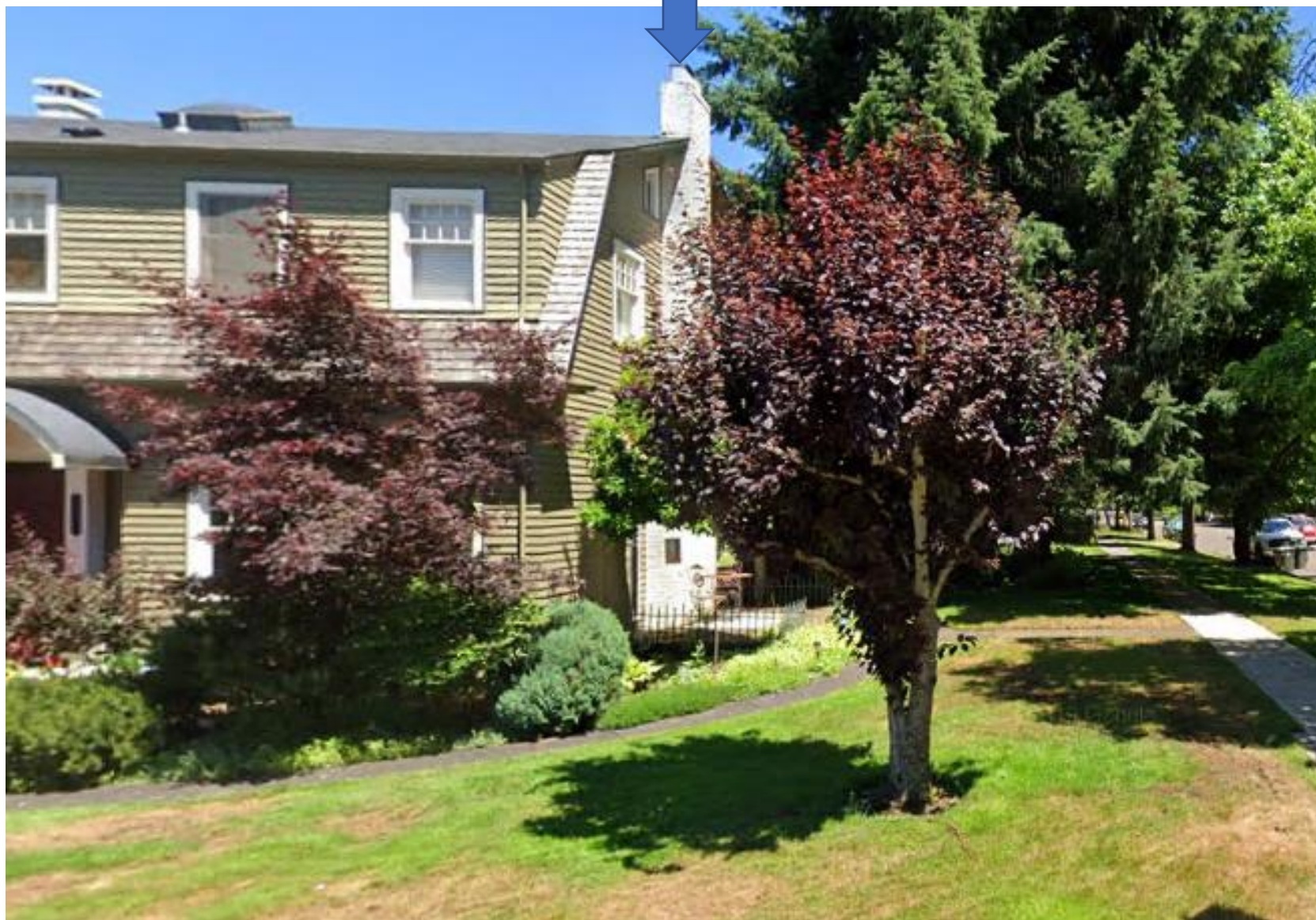
Chimney on Eastern Façade of Carkin House
