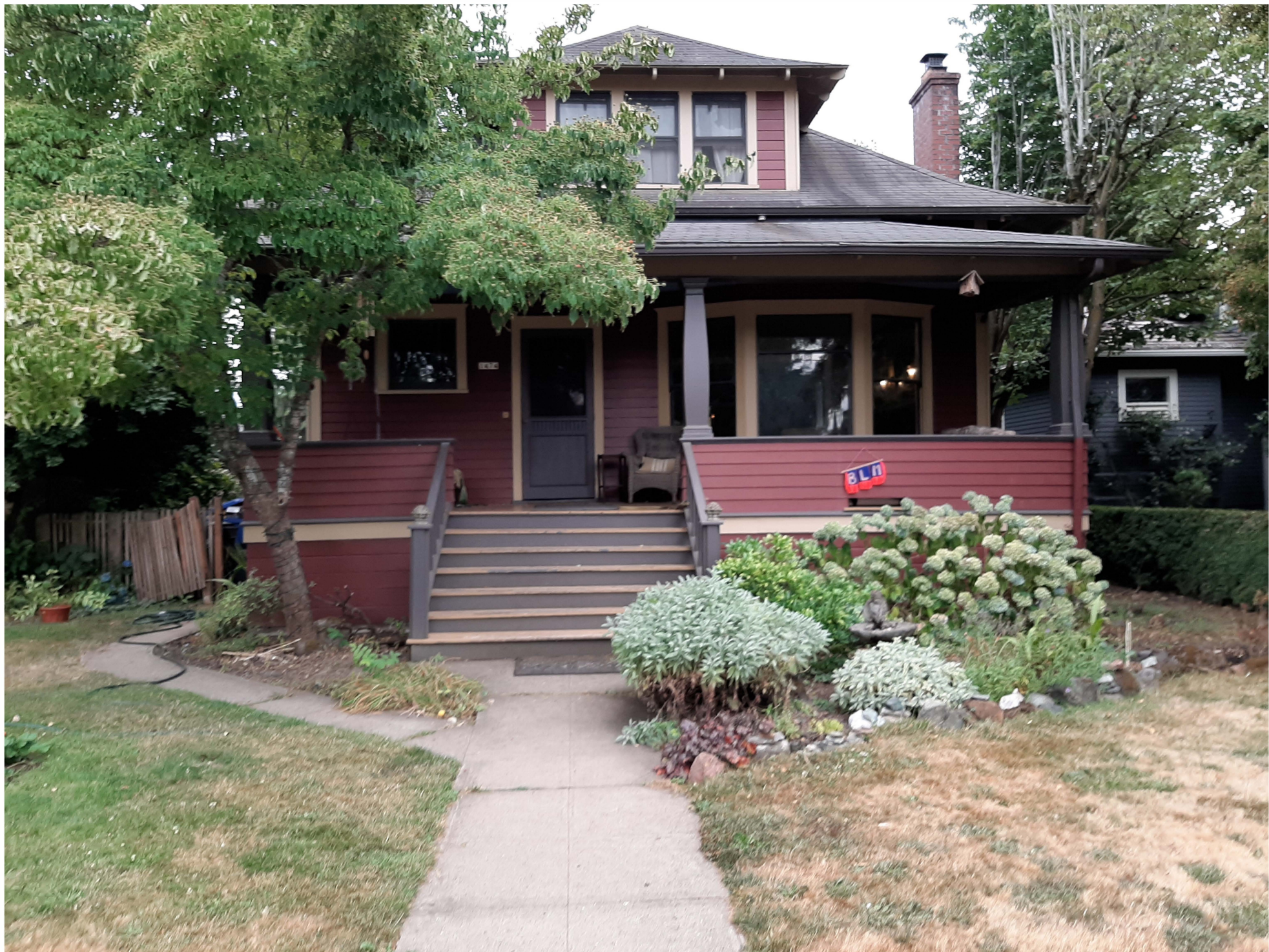
1474 Court Street porch
