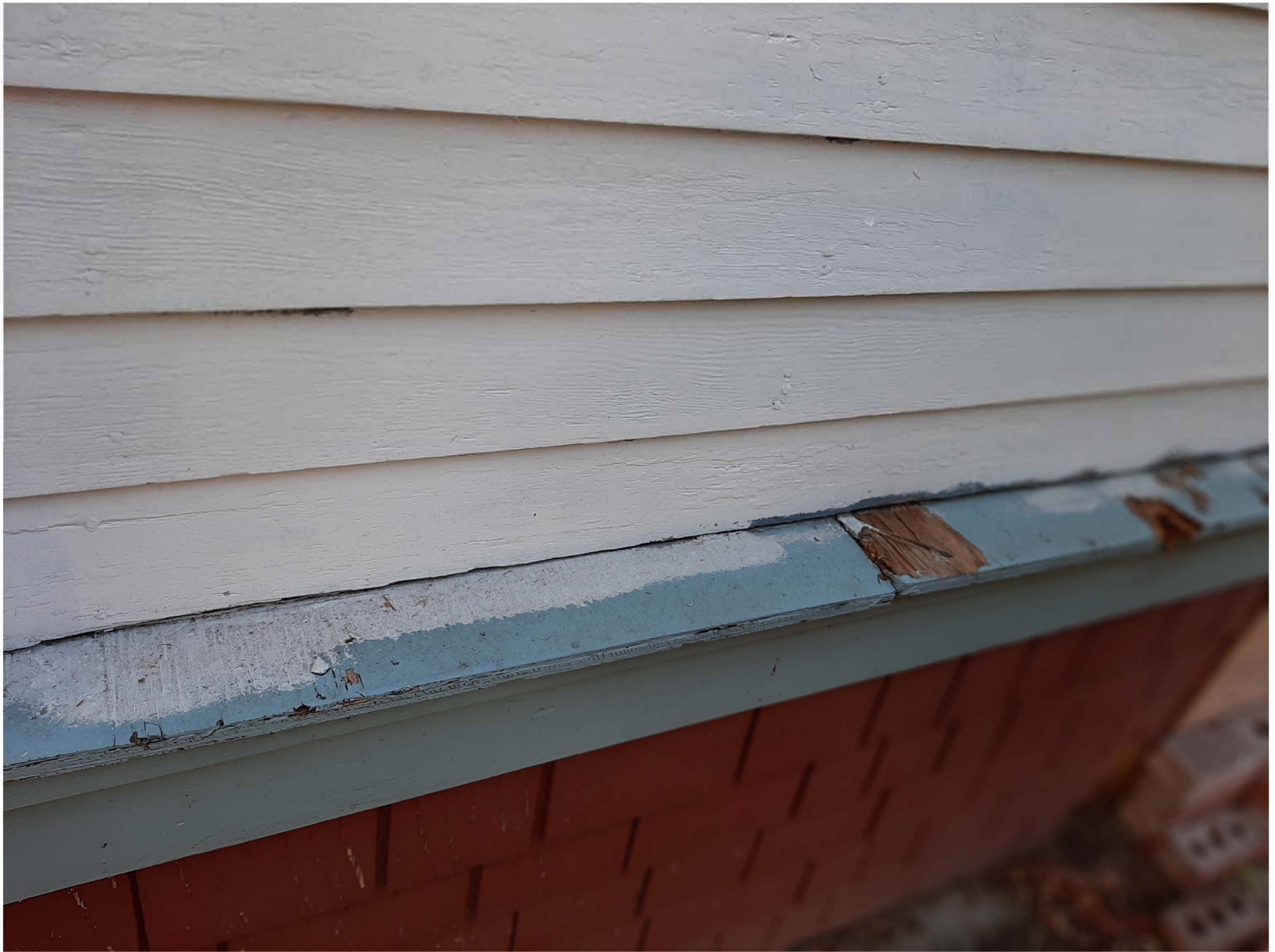
porch subfloor projection
