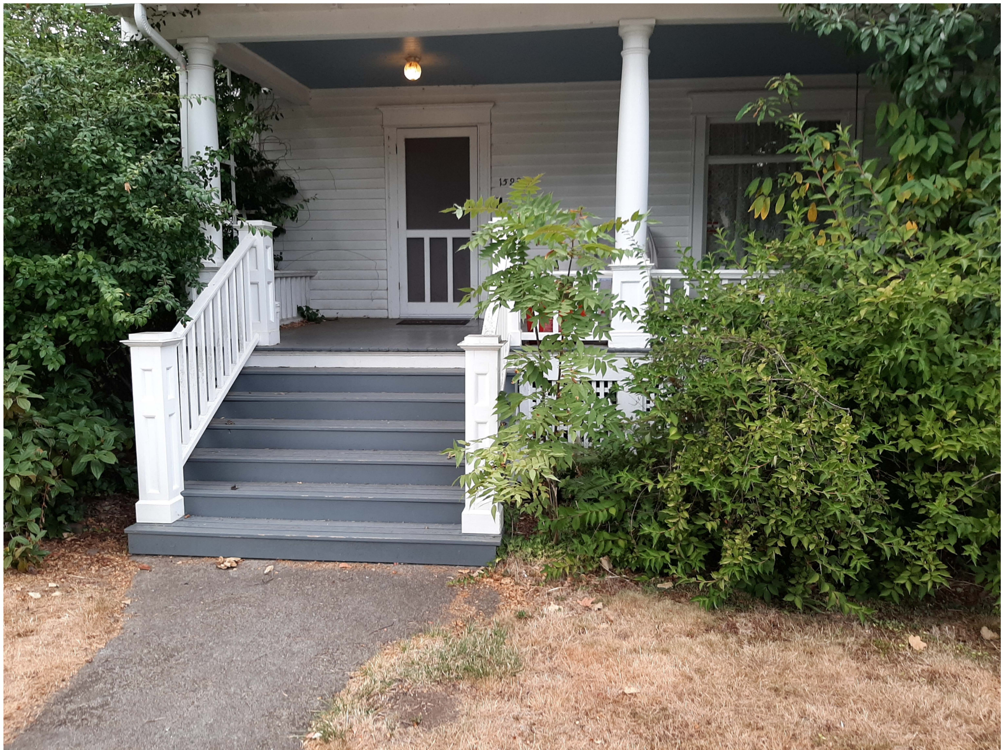
1599 Court Street porch
